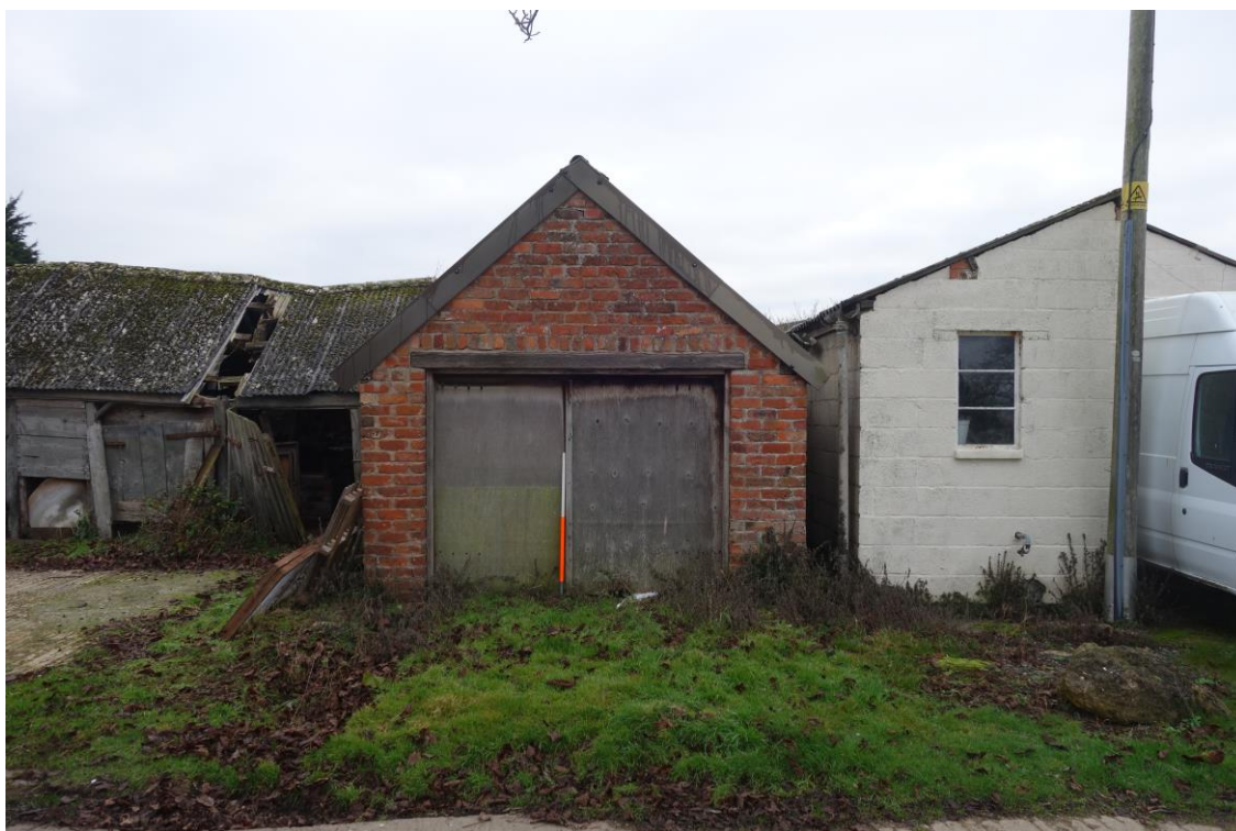
Plate 9: View looking SE showing the NW-gable end of the two-bay range with double-doors for vehicles
