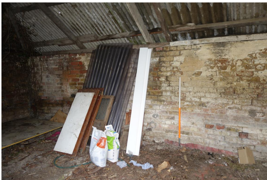
Plate 30: Internal view SE showing whitewashed SW wall of two-bay range
