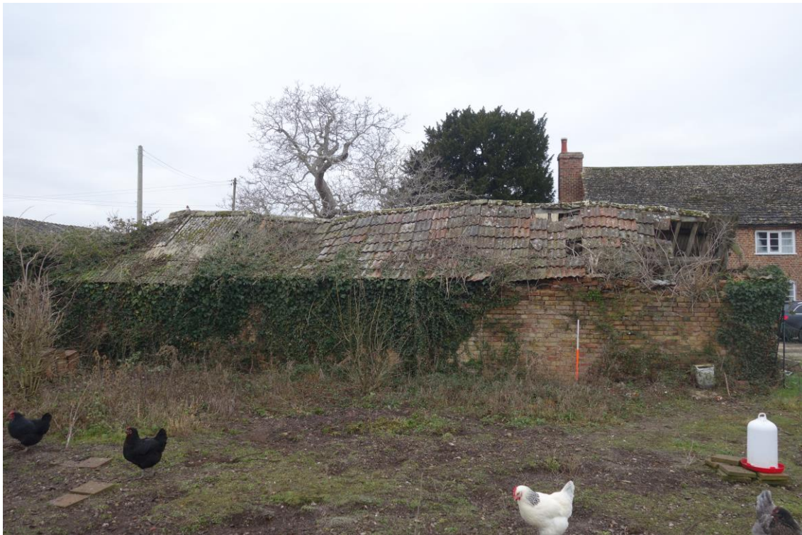
Plate 8: View NW showing the rear (SE) facing elevation of the L-plan outbuilding, heavily obscured by ivy creeper
