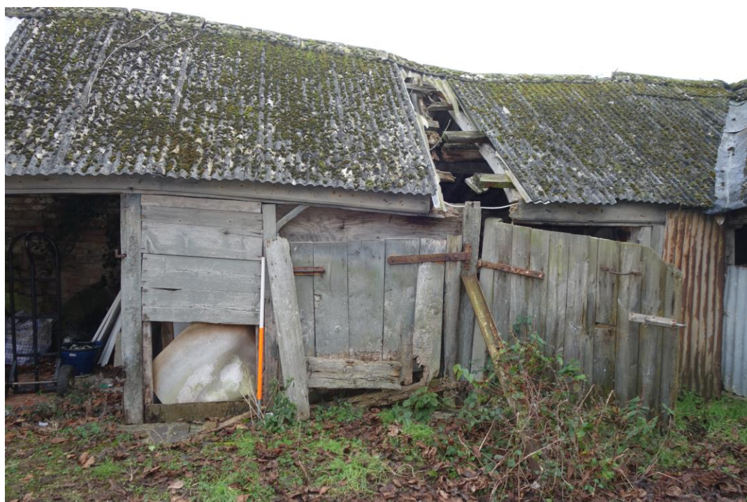
Plate 5: View looking SE showing detail of bays at SW end of four-bay range, with planked stall doors with strap hinges
