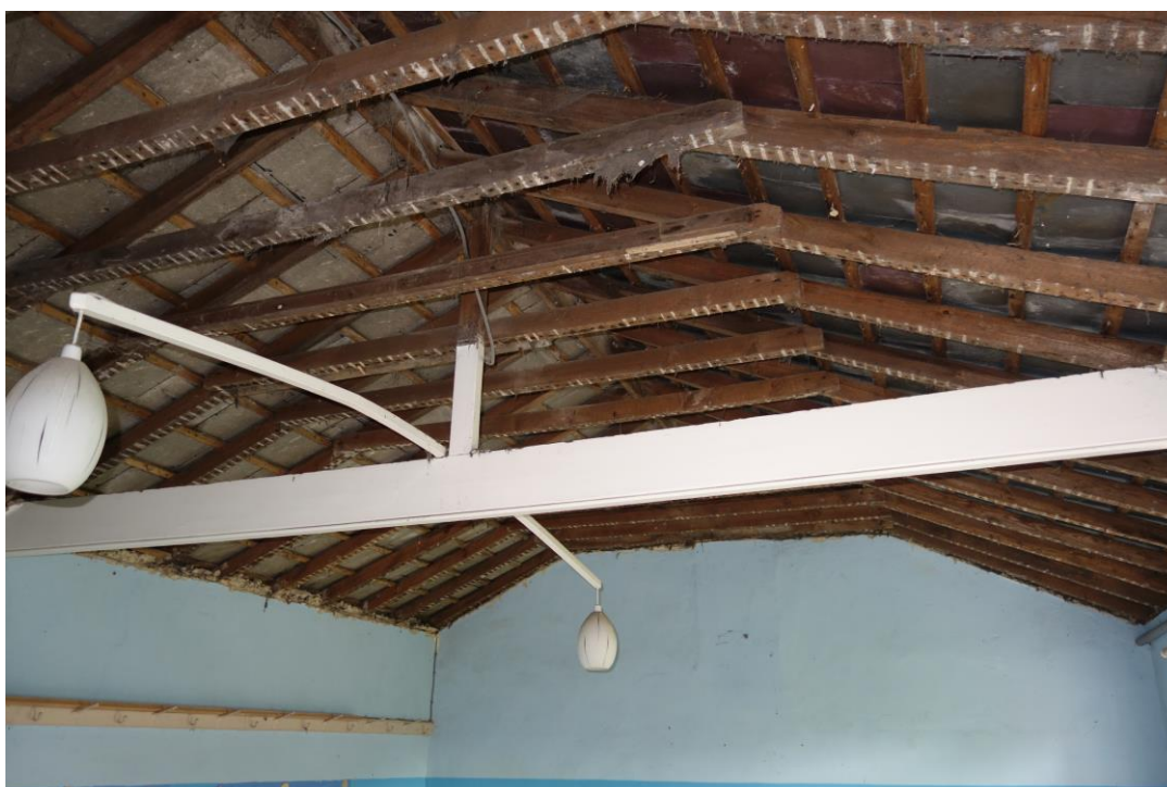
Plate 38: View looking NE showing detail of collar trusses and tiebeam in roof of former schoolroom
