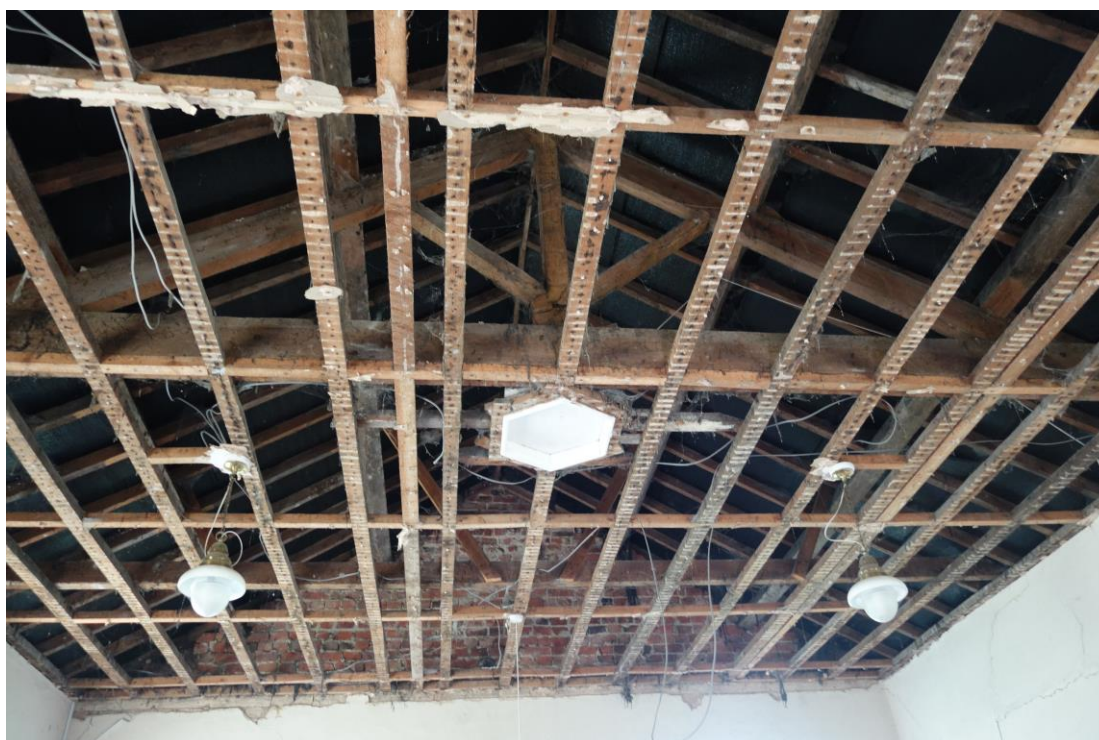
Plate 26: Views looking SE showing detail of roof structure with kingpost roof and hexagonal ceiling hatch
