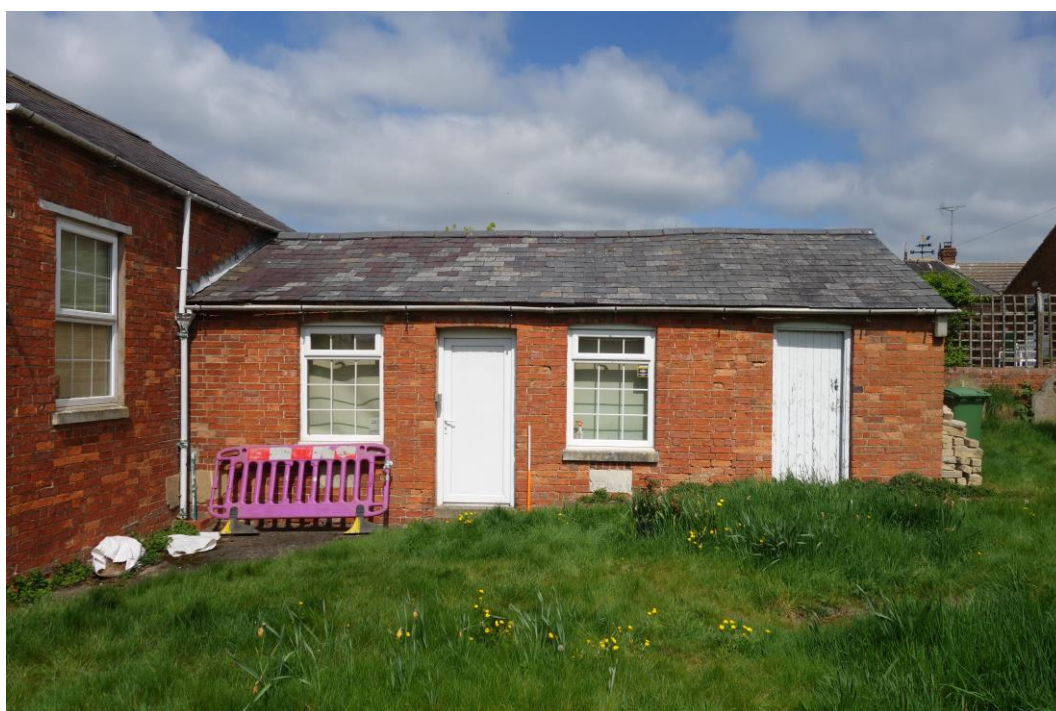
Plate 12: View looking NW showing SE-facing elevation of schoolroom annexe
