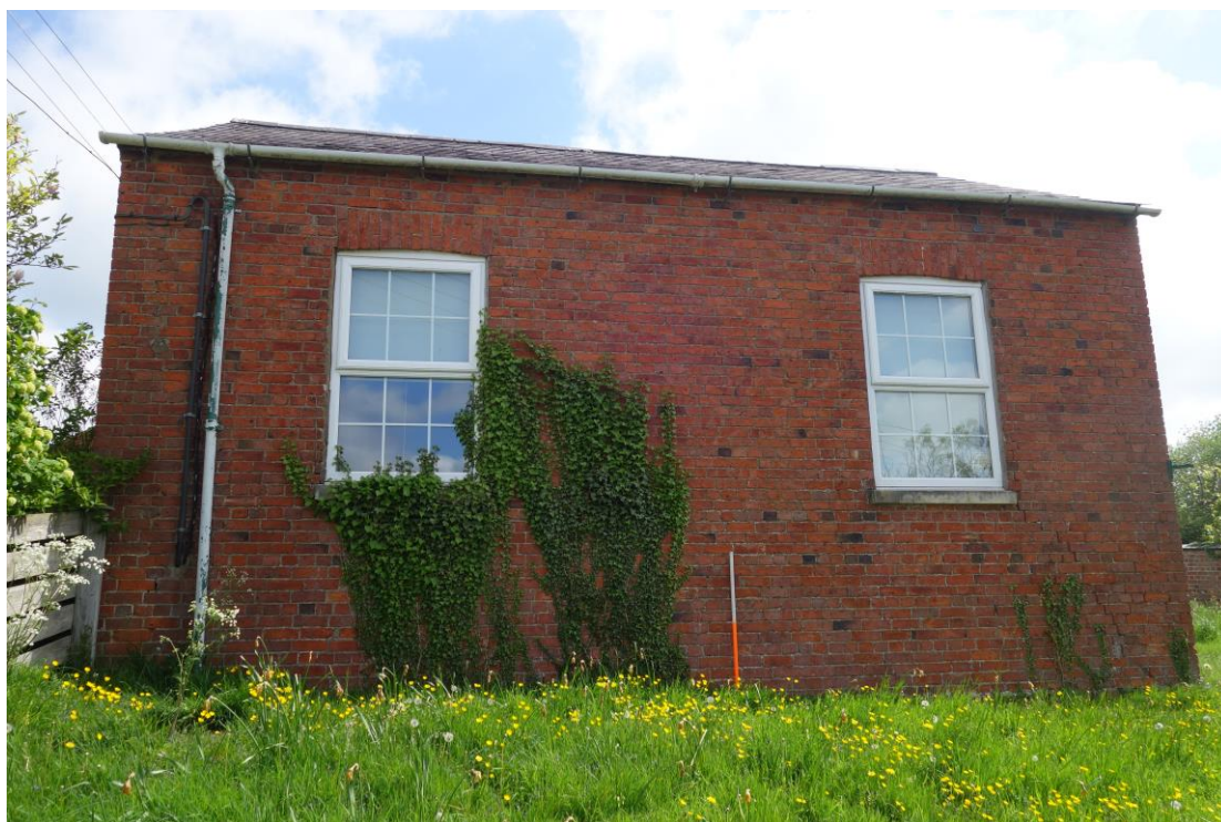
Plate 7: View looking NE showing SW-facing elevation of chapel with low-arched windows with gauged brick headers
