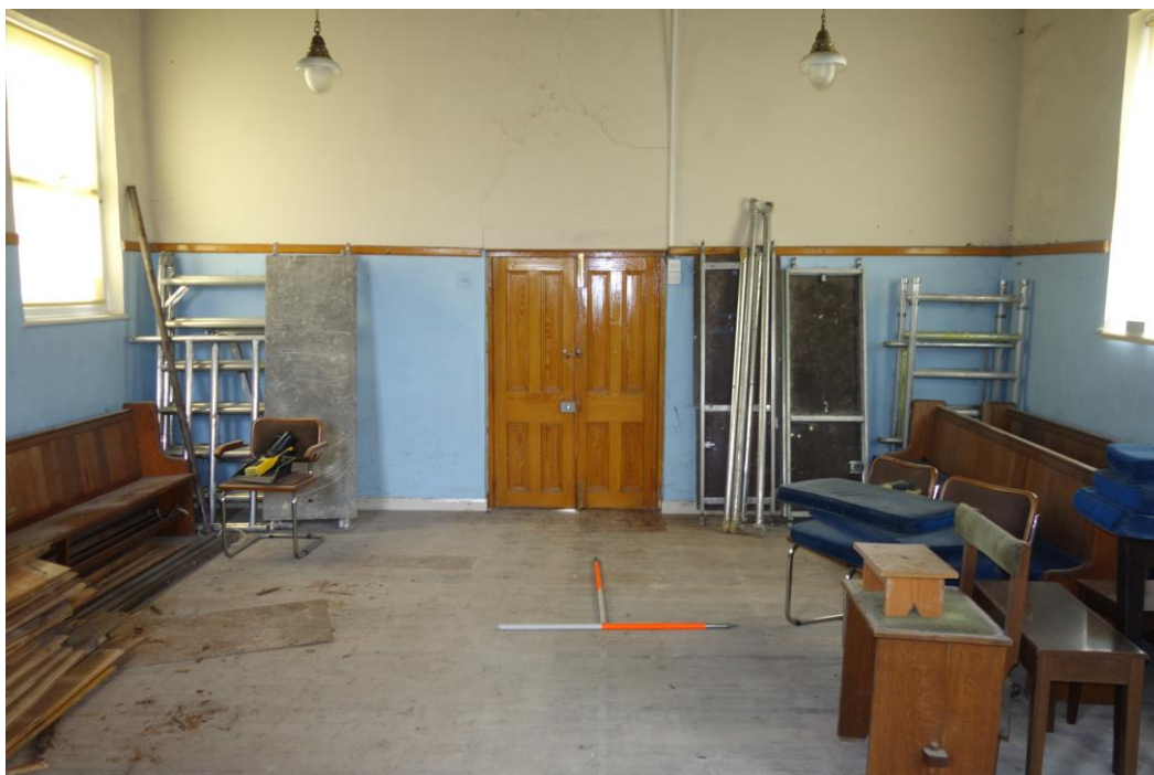
Plate 22: View looking SE towards SE end of chapel showing boarded floor and dado rail
