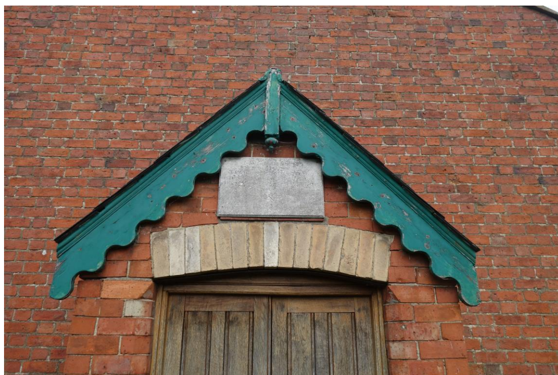
Plate 4: View looking NW showing detail of memorial tablet (1946) and wavy bargeboarding over entrance porch to chapel
