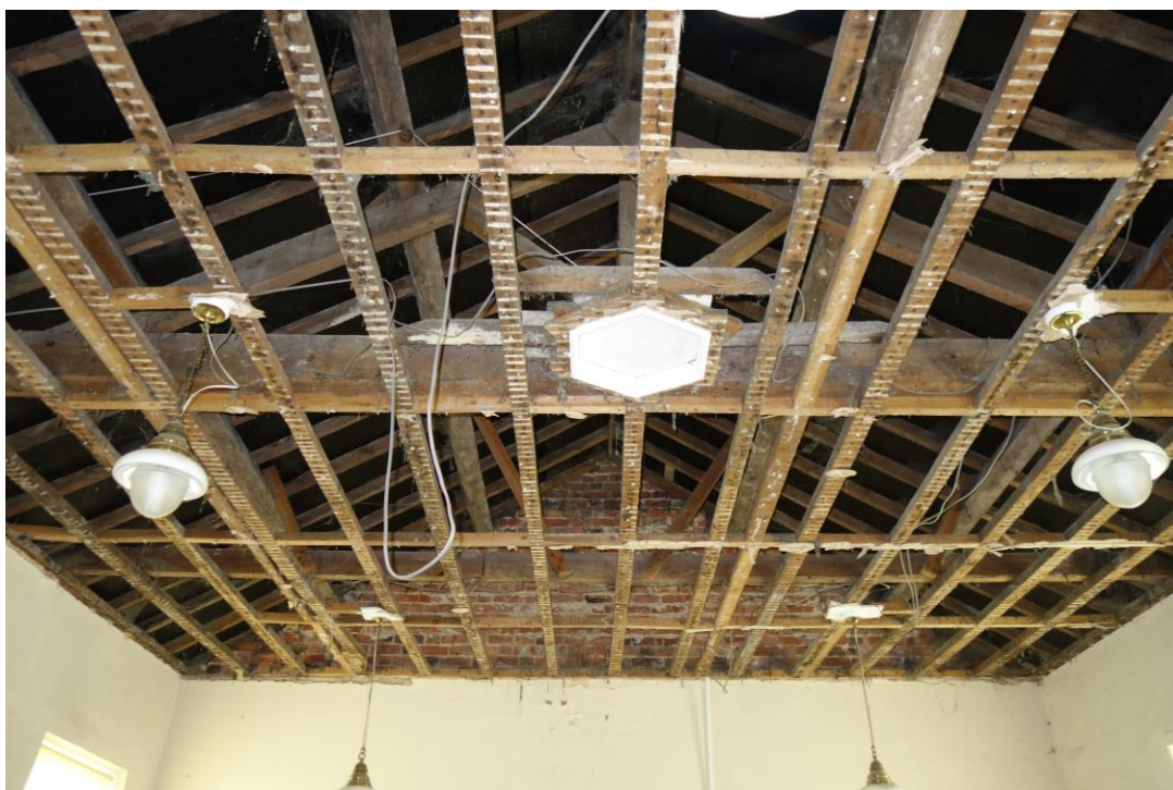
Plate 26: Views looking SE showing detail of roof structure with kingpost roof and hexagonal ceiling hatch
