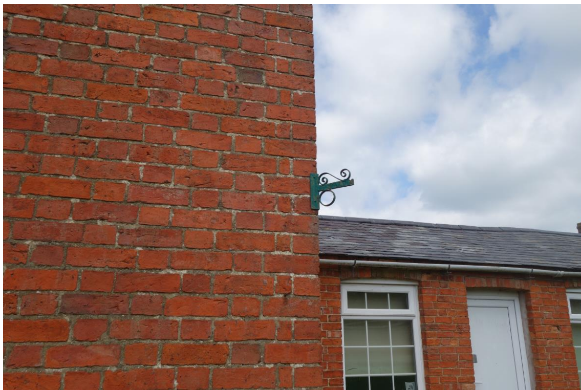
Plate 6: View WNW showing detail of cast-iron scrolled wall bracket attached to the SE corner of the front elevation
