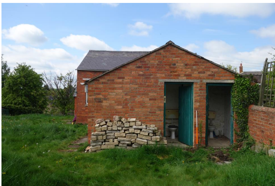
Plate 14: View looking SW showing NE gable end of schoolroom annexe
