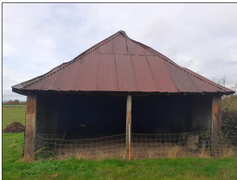
Plate 2: General view looking NW towards front (SE-facing) elevation of cart shed
