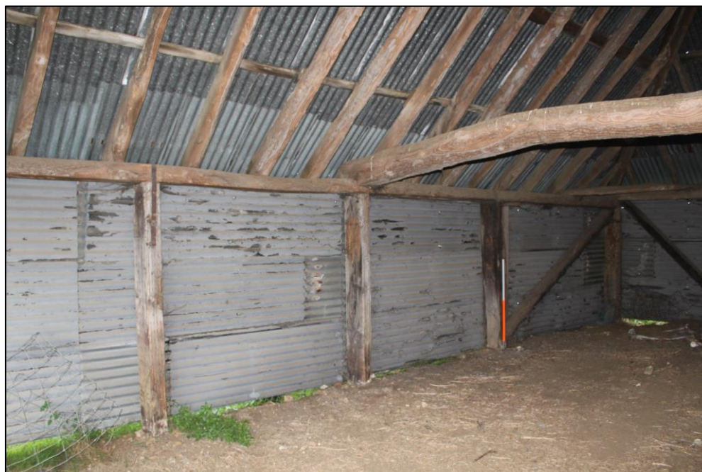
Plate 12: View looking WSW showing timber-framing along SW side of shed with subdivisions marked by vertical wall posts connected to the wallplates by metal straps
