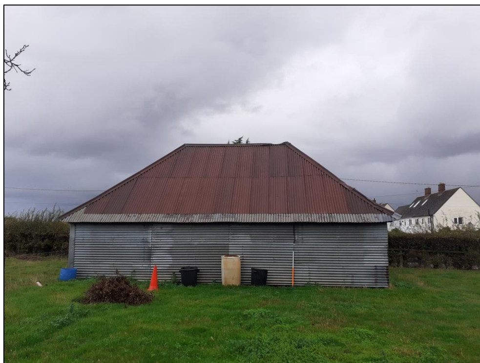
Plate 4: View looking NE showing SW facing elevation of cart shed
