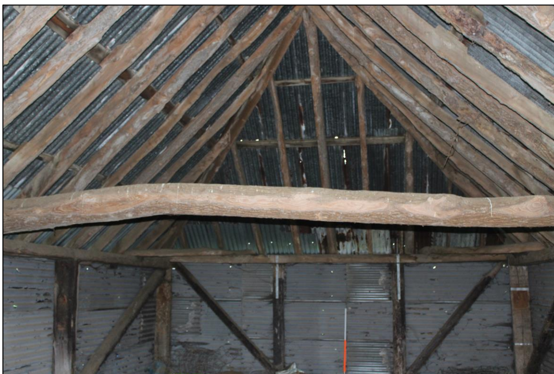
Plate 9: View looking NW showing detail of roughly chamfered central tiebeam
