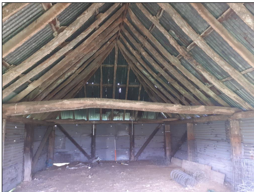
Plate 7: General view looking NW showing interior of shed from SE entrance
