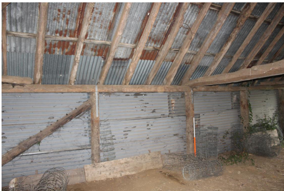
Plate 13: Oblique view looking ENE showing timber-framing along NE side of shed
