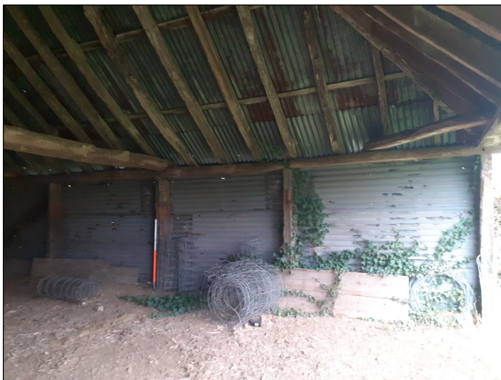
Plate 11: View looking NNE showing timber-framing along NE side of shed with subdivisions marked by vertical wall posts
