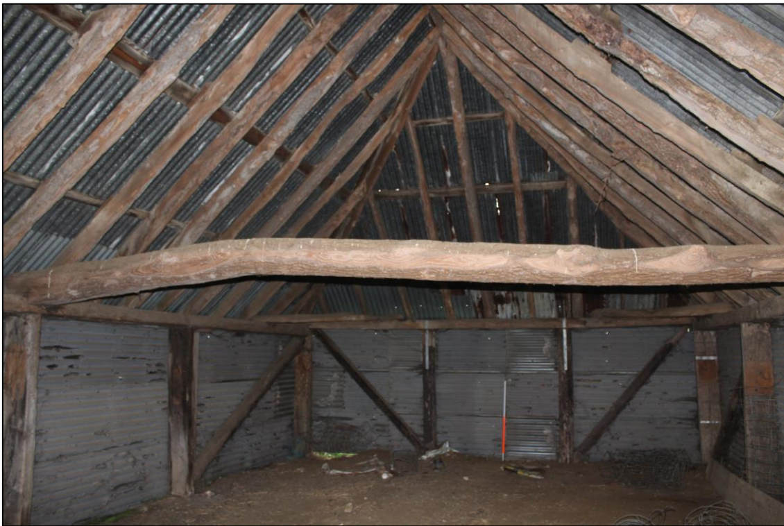
Plate 8: View looking NW showing roof structure and central tiebeam
