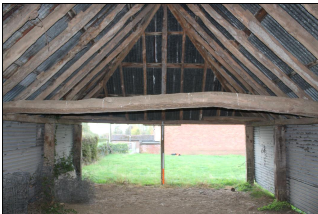
Plate 10: View looking SE showing southeastern portion of shed and tiebeam
