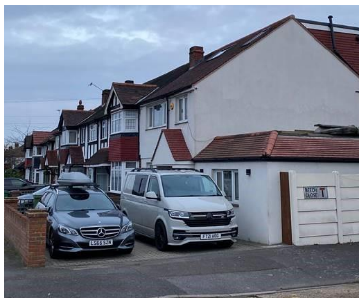
Plate 2: View looking E showing single-storey side extension attached to W end of No. 46 Culvers Avenue
