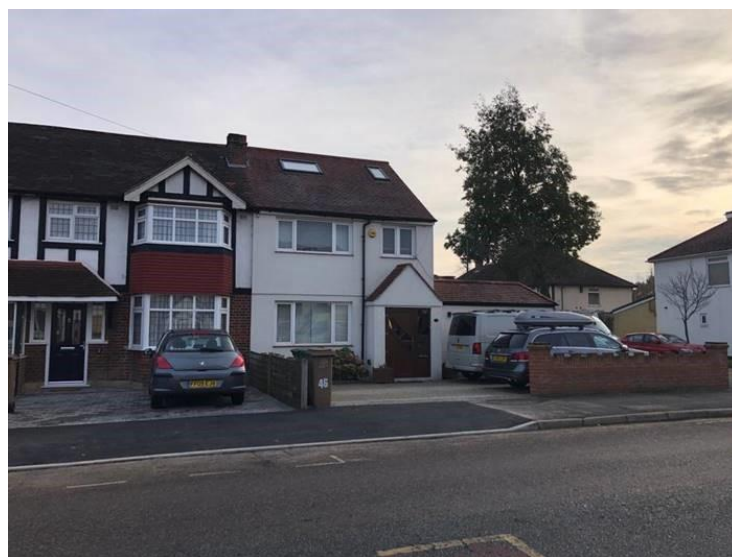
Plate 1: View looking SW towards front of existing semi-detached house at No. 46 Culvers Avenue
