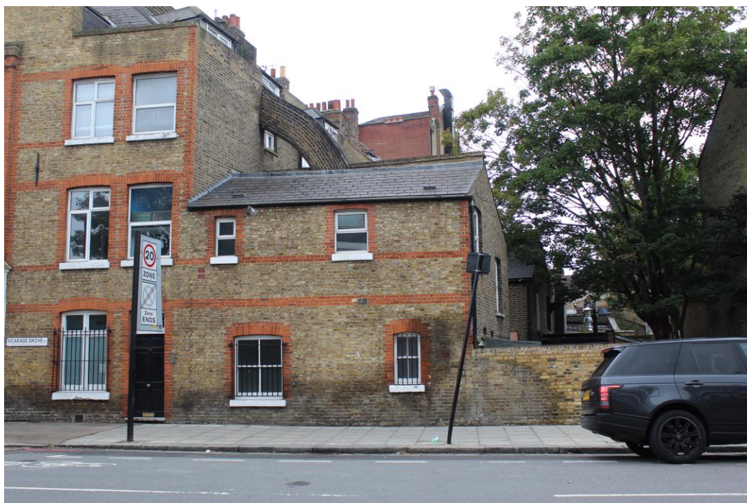
Plate 2: View looking W from Vicarage Grove towards rear portion of site
