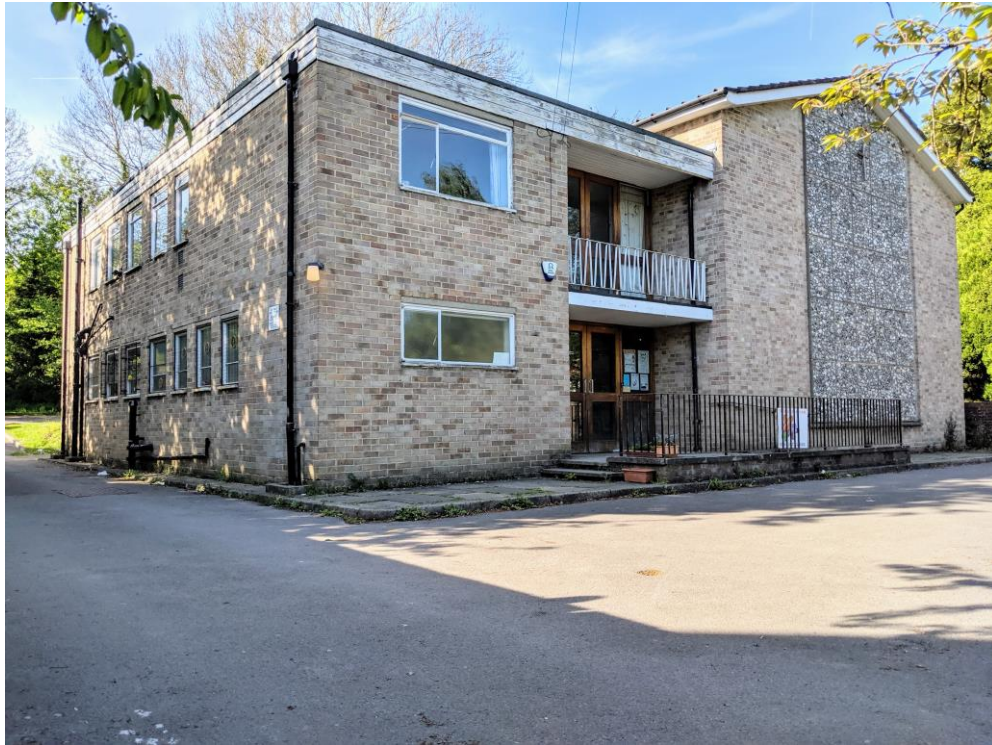
Plate 2: View looking N across car park towards front of St Mary's Church Hall
