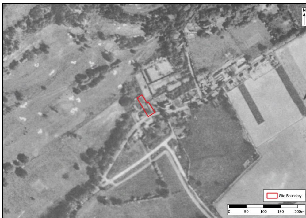
Fig. 16: Extract from an RAF vertical aerial photograph of Addington (1947) (Reproduced courtesy of the Surrey History Centre)
