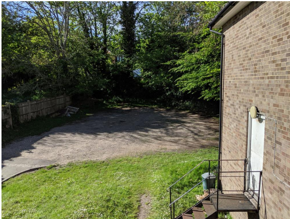
Plate 4: View looking NW showing grassed and tarmac area to rear of Church Hall
