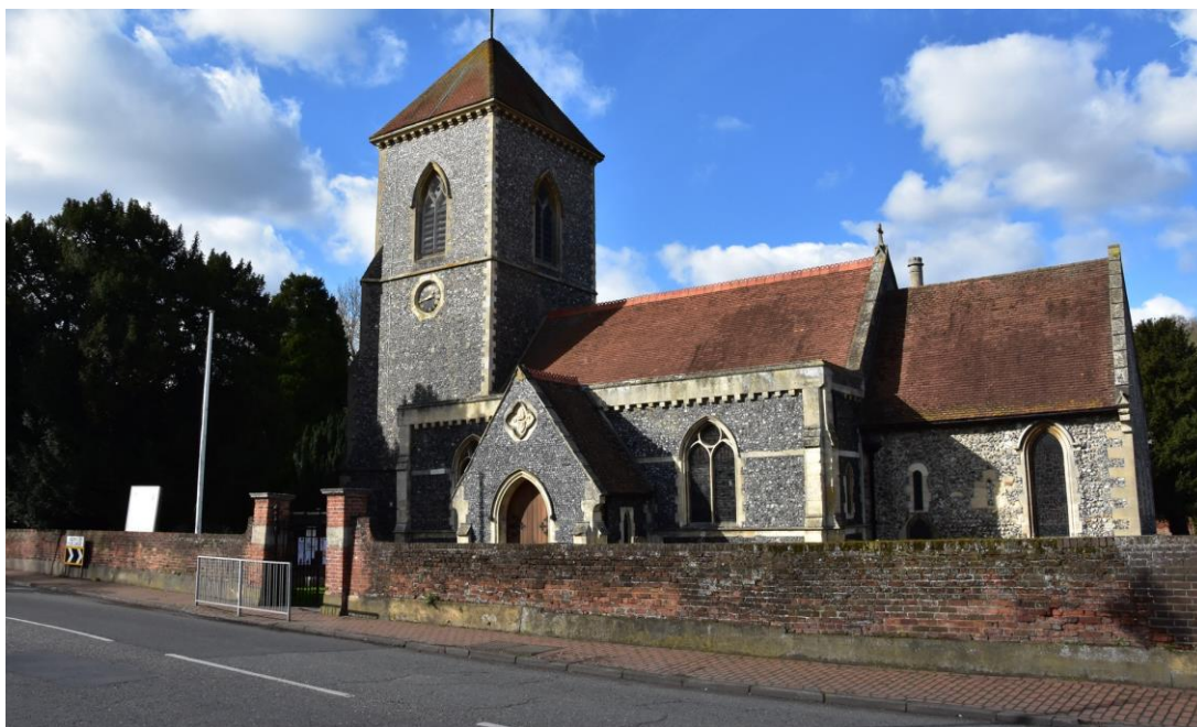
Plate 1: View looking NW towards St Mary's Church Addington
