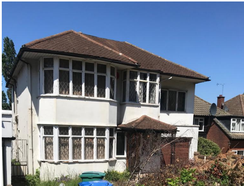
Plate 1: View looking N showing front elevation of existing detached house at No. 35 Sudbury Court Road
