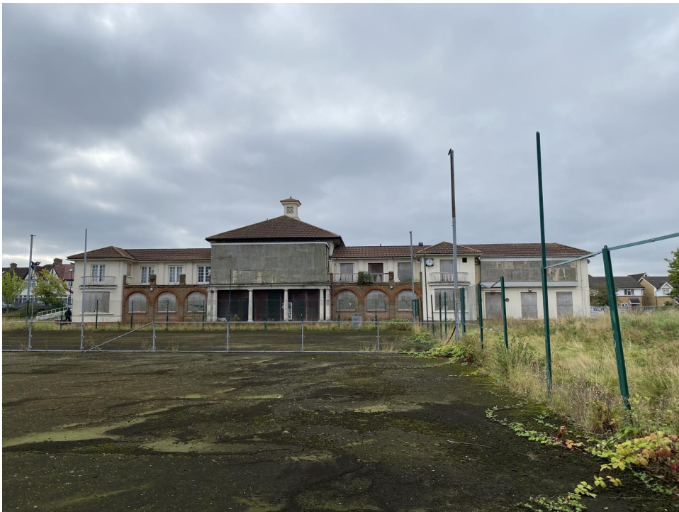
Plate 1: View looking N towards pavilion on terrace at S end of Sports Ground
