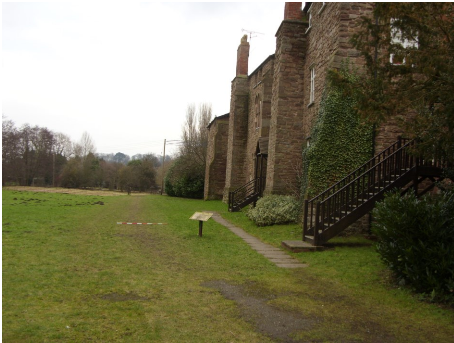
Plate 7: View E from point B (SO 49864 59340), as shown on supplied location plan, showing proximity of existing path to the Old Priory buildings (right)
