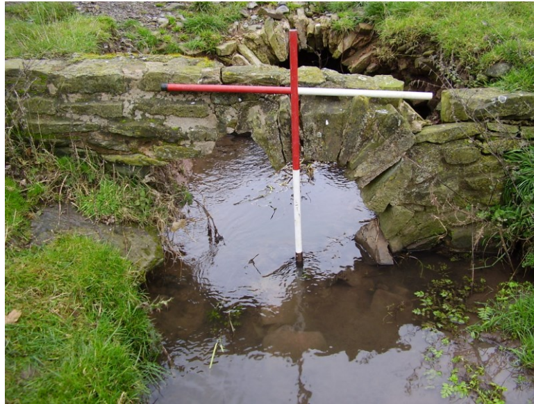
Plate 2: View NE showing SW outer face of culvert
