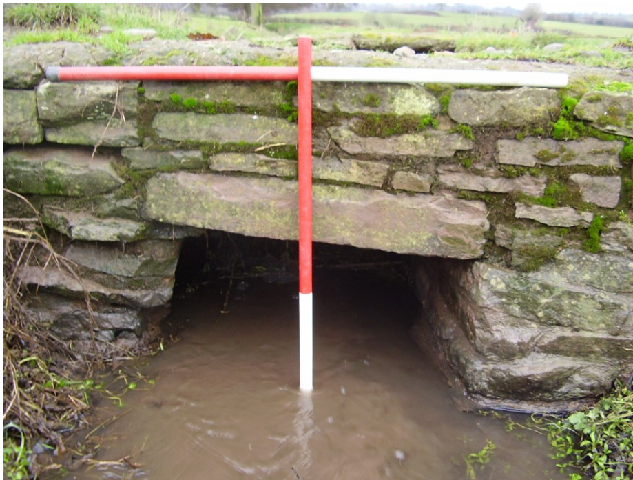
Plate 4: NE face of culvert. View SW
