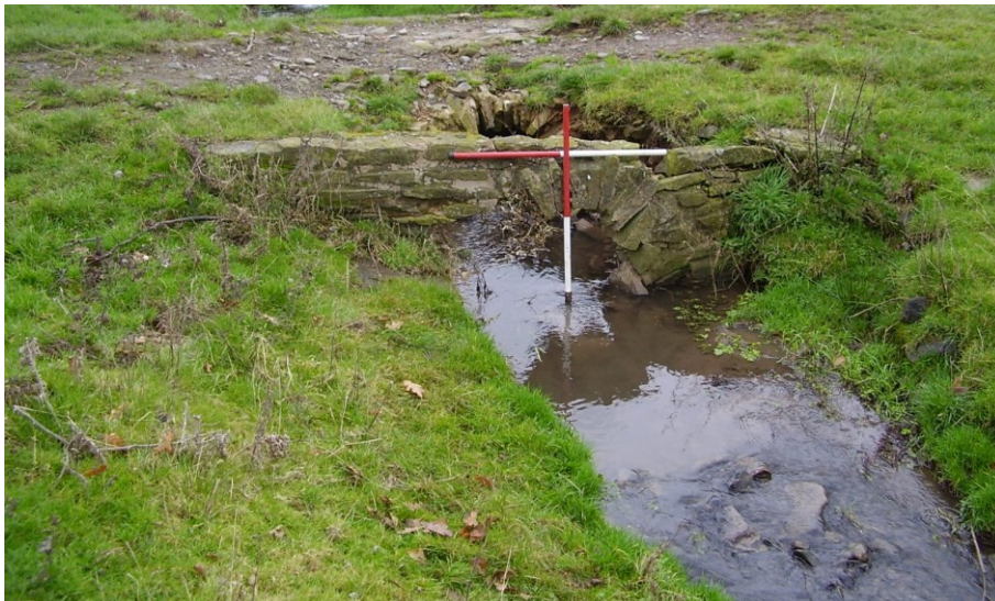
Plate 1: Overview of culvert. View NE
