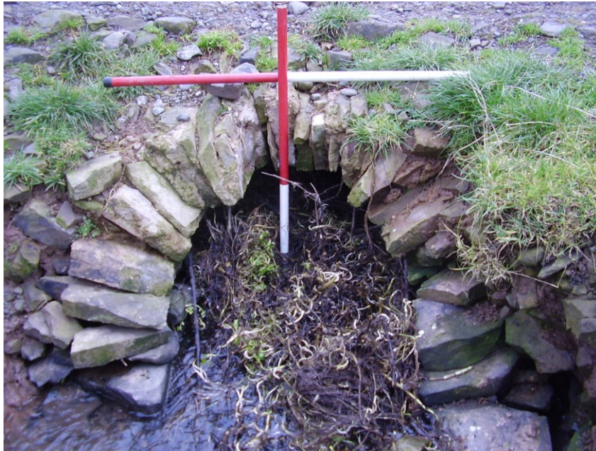
Plate 3: Central section of culvert, detailing construction. View NE.
