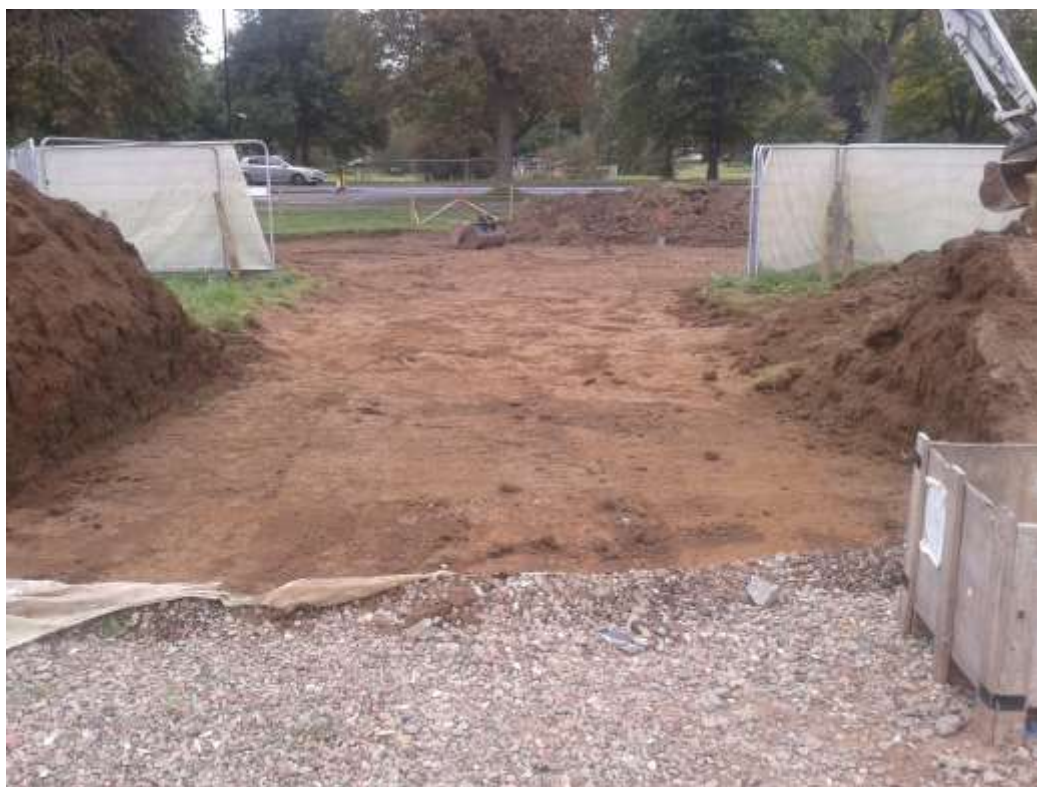
Plate 16: View E showing access way from the Compound onto the easement
