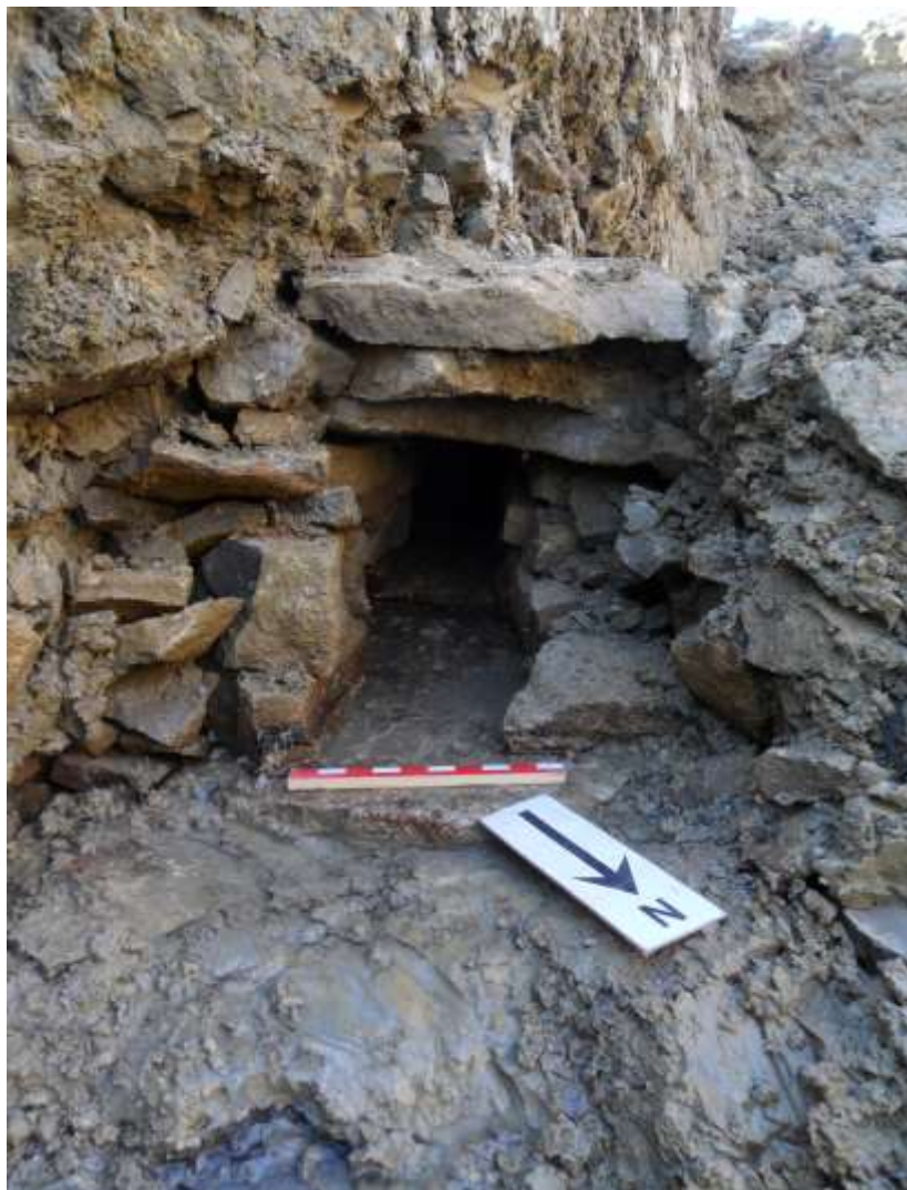
Plate 31: View SW of masonry culvert [204] (20cm scale)
