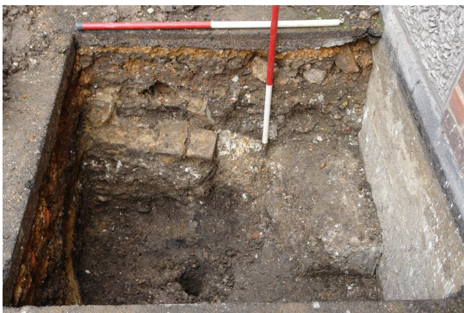
Plate 8: View looking N showing S-facing section of Test Pit 1 with shallow footings for 19 th century brick wall (202) truncated by concrete foundations for existing 1960s offices
