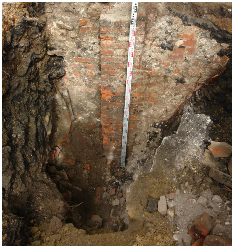
Plate 1: View looking N showing S elevation of post-medieval cellar wall (130) of brick and flint and chalk masonry construction
