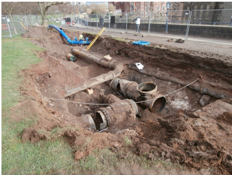
Plate 55: View to the SE, working shot of 26 showing exposed services
