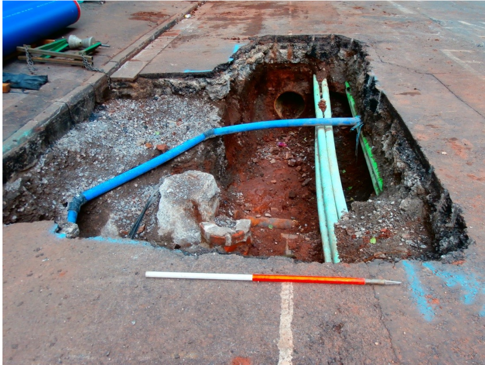
Plate 29: View to the N of Trench 12
