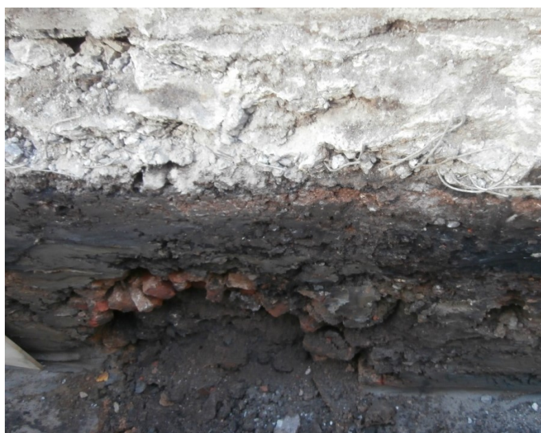
Plate 41: View NW of brick culvert (1720)
