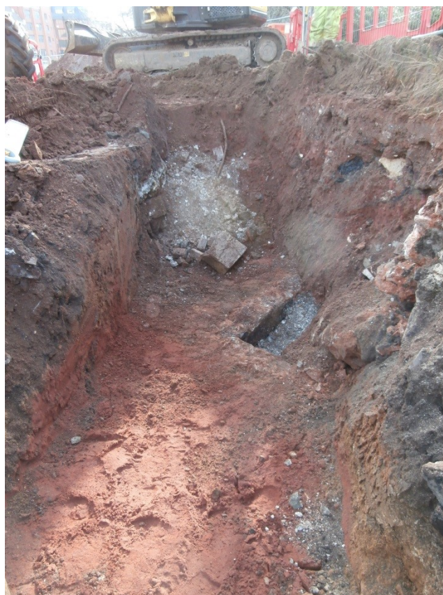
Plate 53: View SW of wall foundation (2521)
