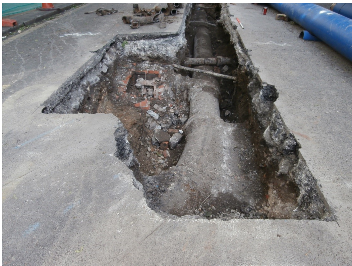
Plate 11: View N showing exposed 19 th -century water main in Trench 3
