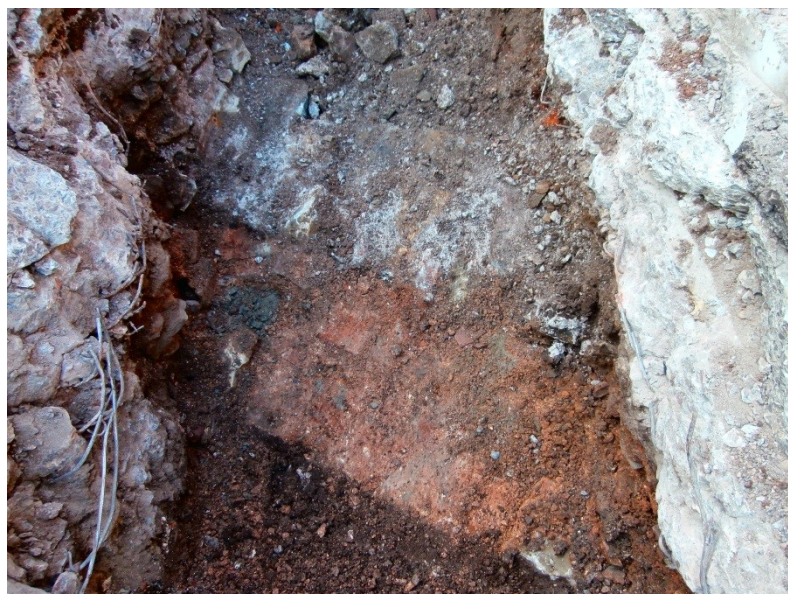
Plate 39: View NW showing wall foundation (1706)
