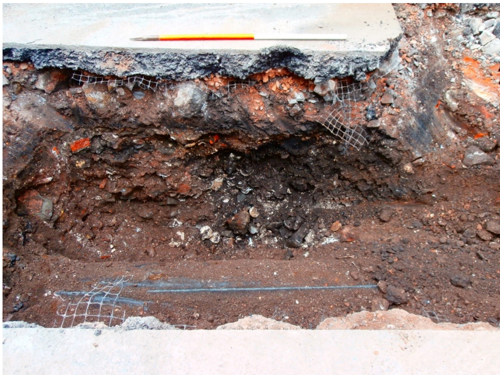
Plate 20: View to the W showing deposit (703) in the E-facing section, which would appear to represent a dump of probable domestic waste evidently predating the installation of the 19 th -century water main
