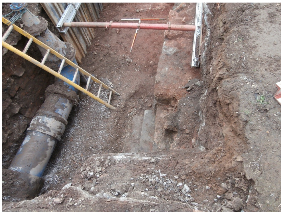
Plate 71: View to the SE of structures (3203) and (3206)
