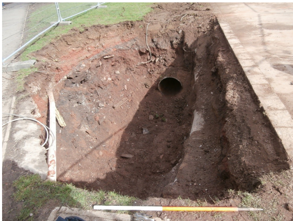
Plate 58: View to the W of Trench 28
