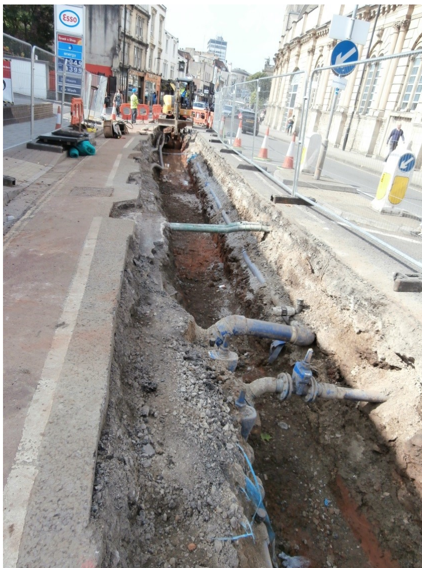
Plate 43: View to the W of Trench 18
