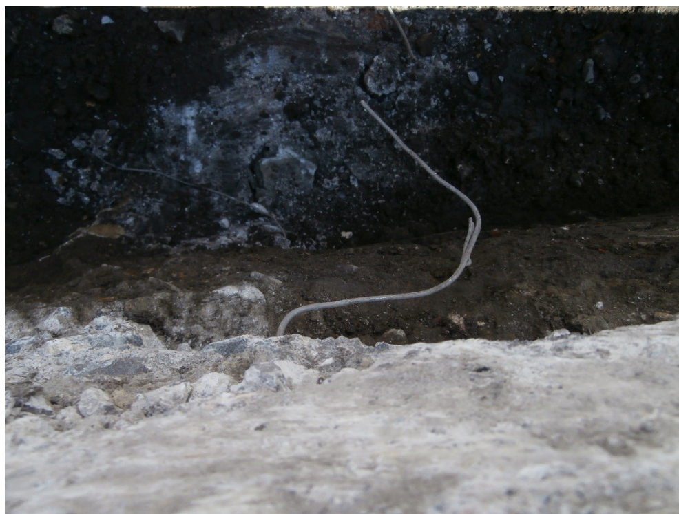
Plate 84: View to the NE of wall foundation (4305)
