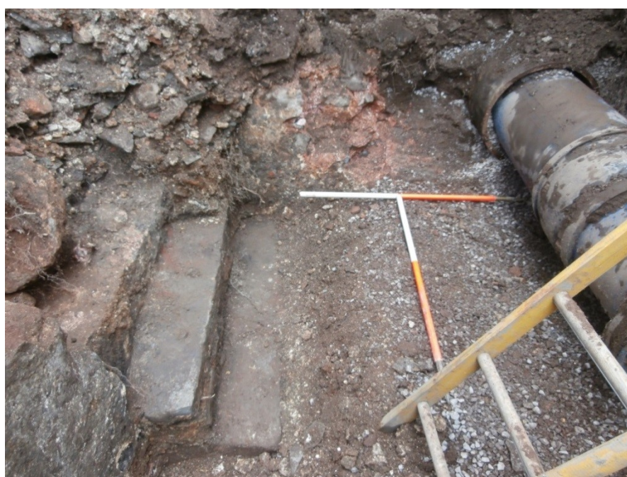
Plate 67: View to the NW of structure (3203)
