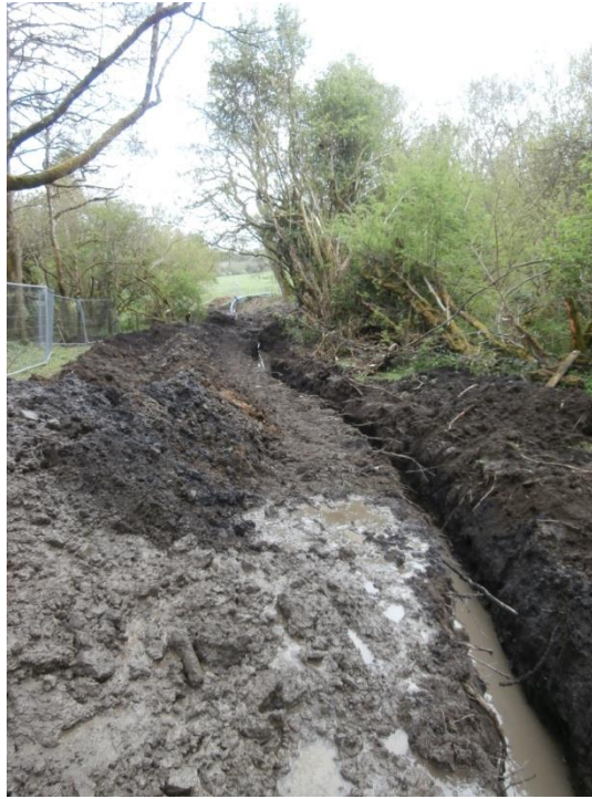
Plate 2: Open-cut trenching in colliery area facing ESE
