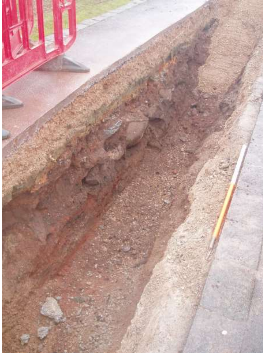
Plate 8: View looking NNE along Trench 7 showing concentration of worked stone in demolition deposit (705) in SE-facing section of trench
