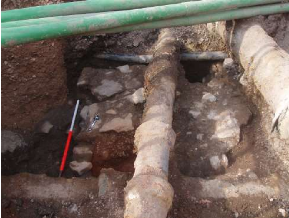
Plate 11: View looking NW showing wall (909) overlaid and partially truncated by late 19 th -20 th century service pipes
