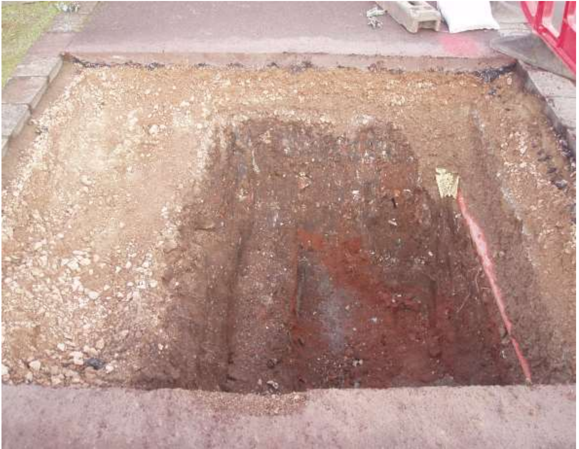
Plate 6: View looking NE showing SW-facing section of Pit 4
