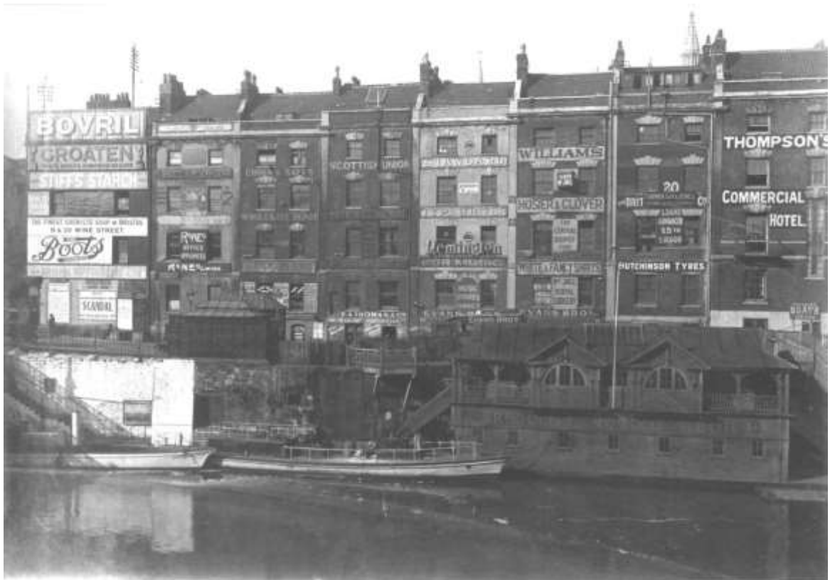
Plate 13: Photograph taken in the early 1920s looking NW across the river towards Back Bridge Street, showing the archway and landing stage in the bottom left-hand corner of picture (Reproduced by courtesy of Bristol Record Office)
