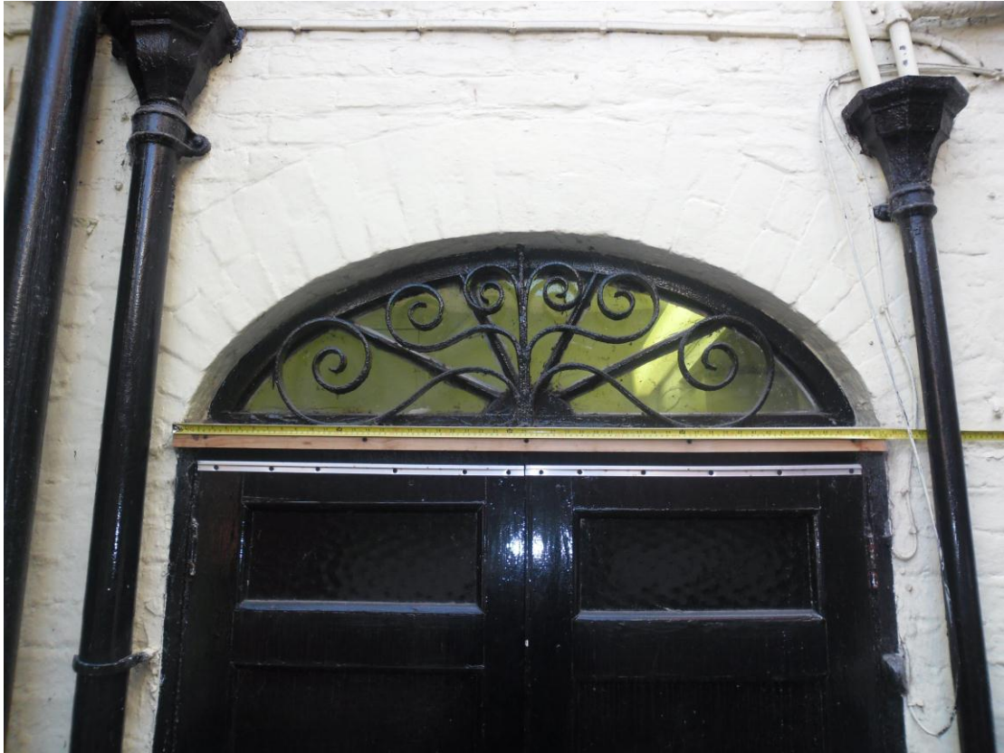
Plate 5: View SW showing detail of wrought-iron scrollwork in front of fanlight above doorway in NE-facing elevation
