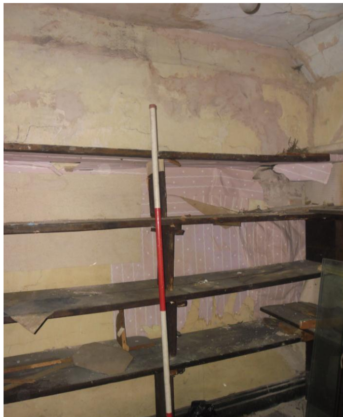
Plate 34: Internal view looking SE showing shelving in storeroom adjacent to second-floor room at SE end of corridor
