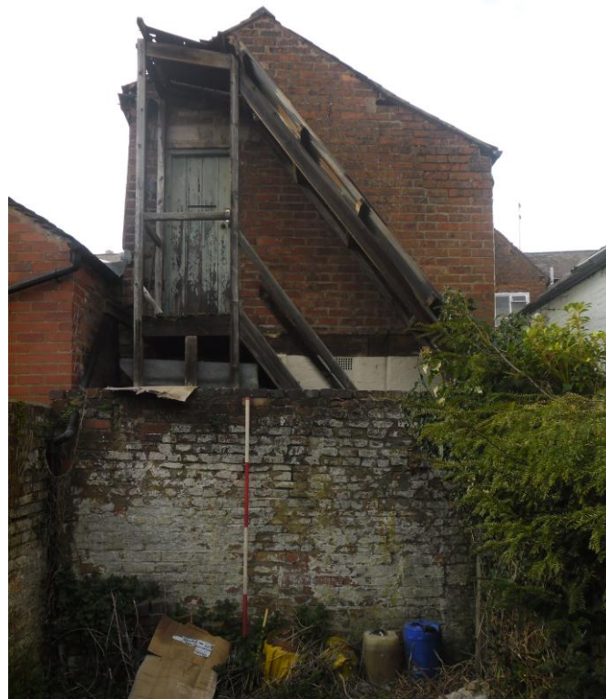
Plate 12: View looking NW showing SE-facing gable elevation of gabled extension to printing works, with wooden stair leading to entrance at first-floor level.
