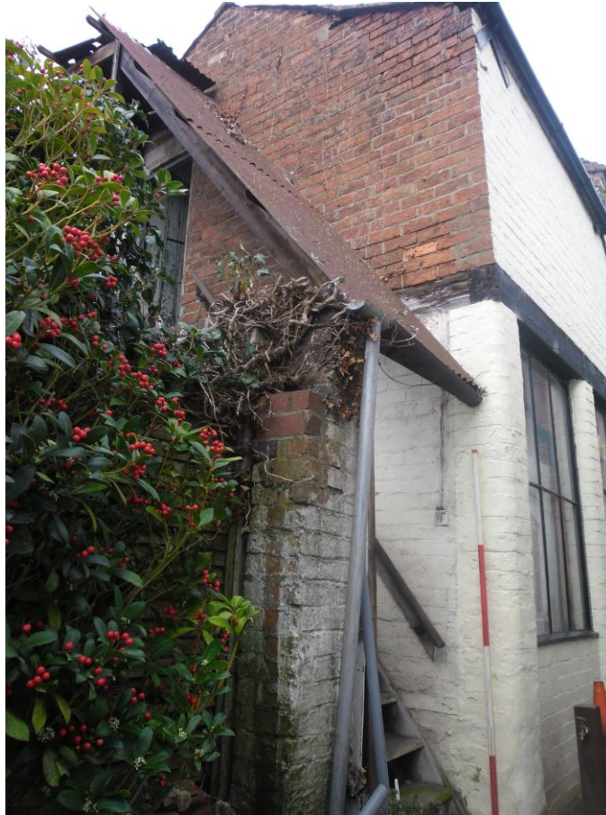
Plate 11: View NNW showing gabled extension at SE end of printing works (with cross ties inserted in the NE-facing elevation at eaves level)
