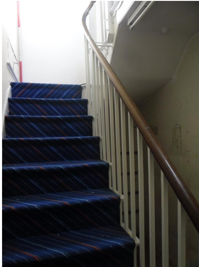
Plate 24: Internal view looking up first-floor staircase to half-landing showing newel posts and iron rods connecting the treads to the opposite handrail and balusters
