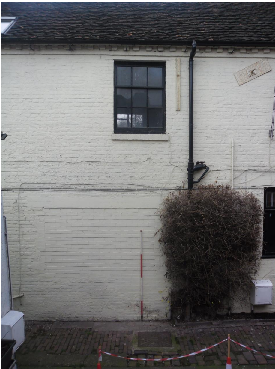
Plate 10: View looking SW showing blocked window opening in centre of NE elevation of printing works, with 19 th century sash window visible at first-floor level
