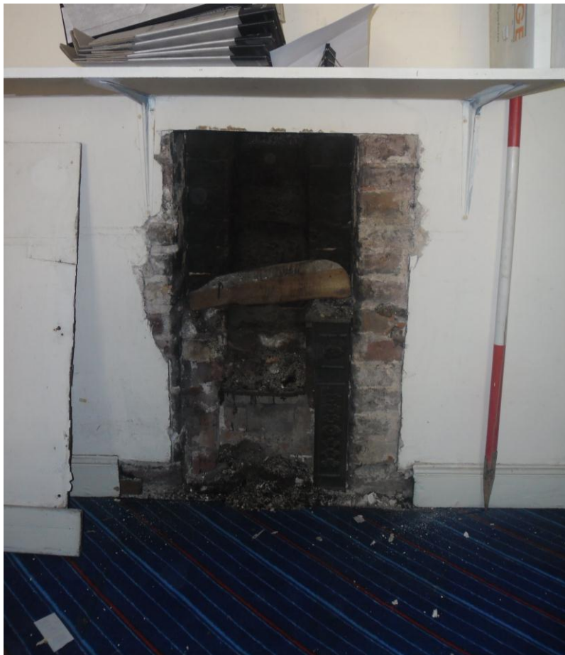
Plate 28: Internal view looking SE showing detail of fireplace grate with foliage decoration in second-floor room overlooking Load Street
