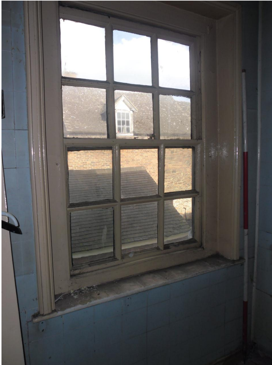
Plate 16: Internal view looking E showing box-framed sash window in bathroom/shower-room on first floor surrounded by modern ceramic panels
