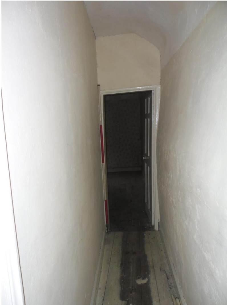
Plate 26: Internal view looking SE along second-floor corridor, showing coved ceiling
