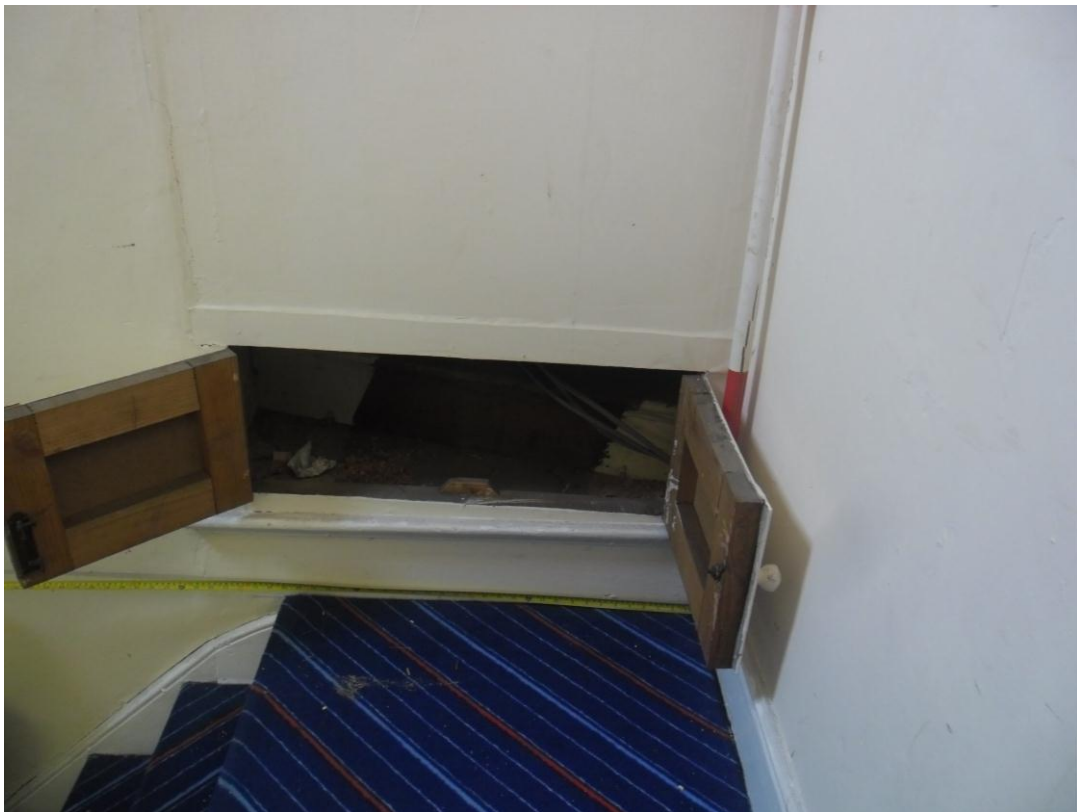
Plate 23: Internal view looking NW showing blocked doorway and stairs in SE-facing wall on half-landing between first and second floors
