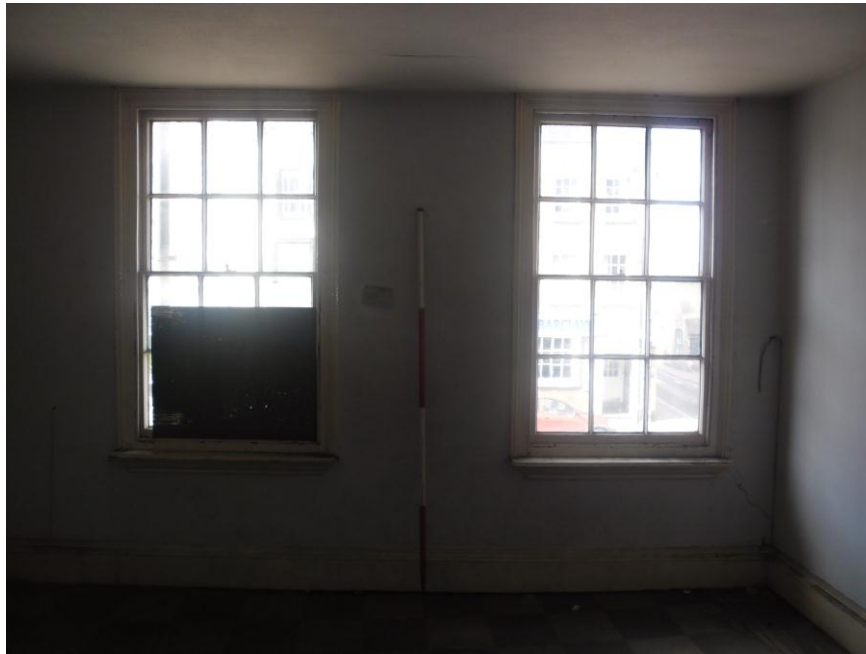
Plate 19: Internal view looking NW showing 12-pane sash windows in first-floor room overlooking Load Street
