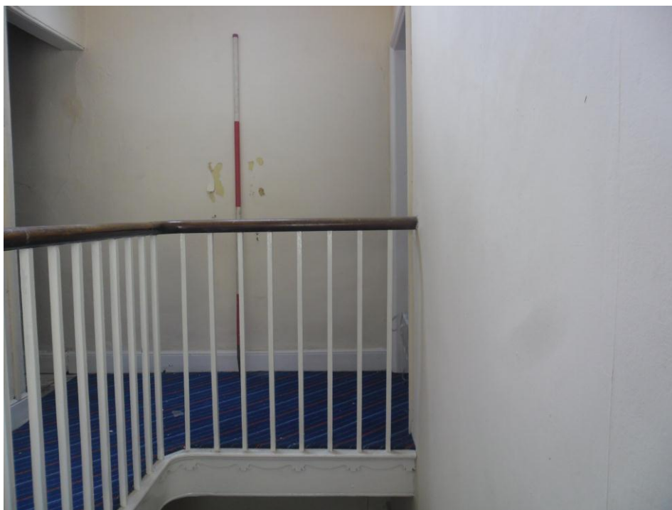
Plate 25: Internal view looking SW showing second-floor landing
