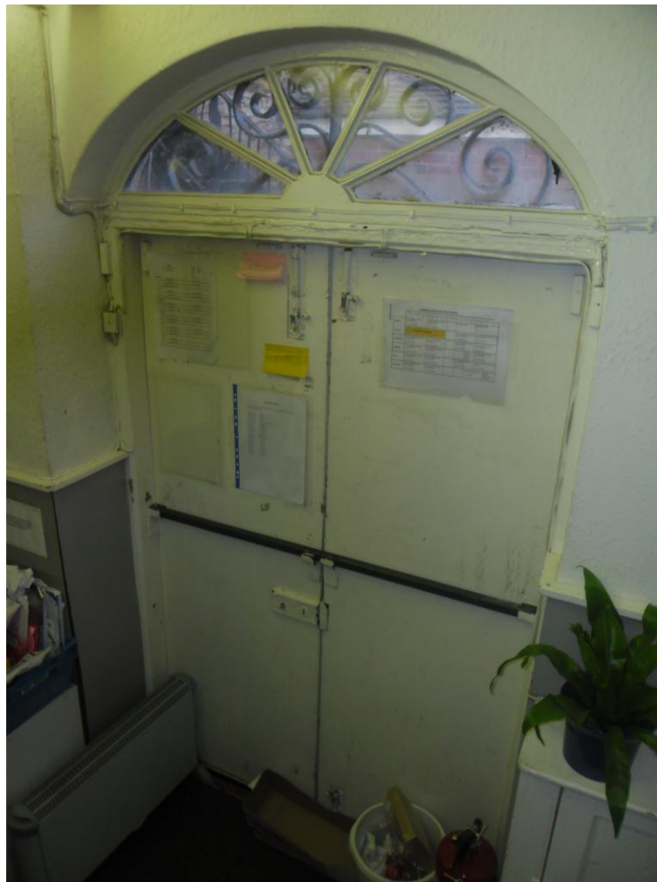
Plate 14: Internal view looking NE showing the round-headed door in the ground floor lobby with 5-pane fanlight and external wrought iron scrollwork
