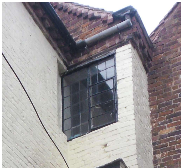
Plate 7: Detail showing second-floor casement window in SE-facing elevation with splay to left
