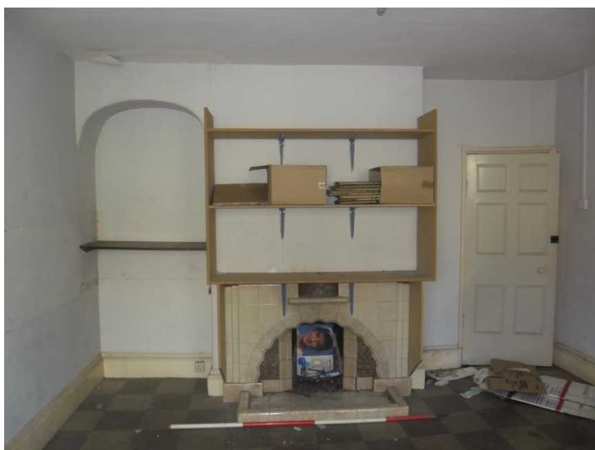
Plate 20: Internal view SE showing Art Deco fireplace in first-floor room and arched recess to left
