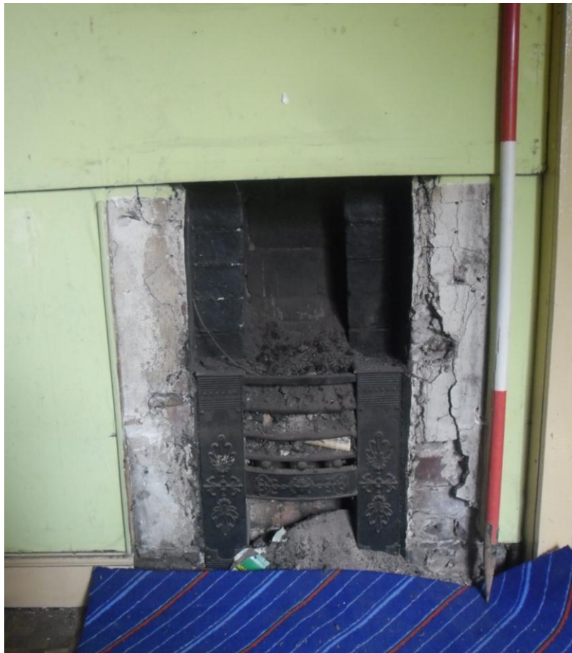
Plate 18: Detail of iron fireplace grate in first-floor room showing acanthus leaf detailing in panels and crosspiece
