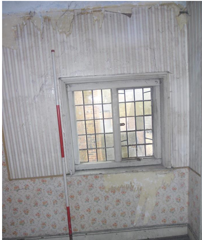
Plate 33: Internal view looking NE showing casement window in SW-facing wall of room to SE of corridor
