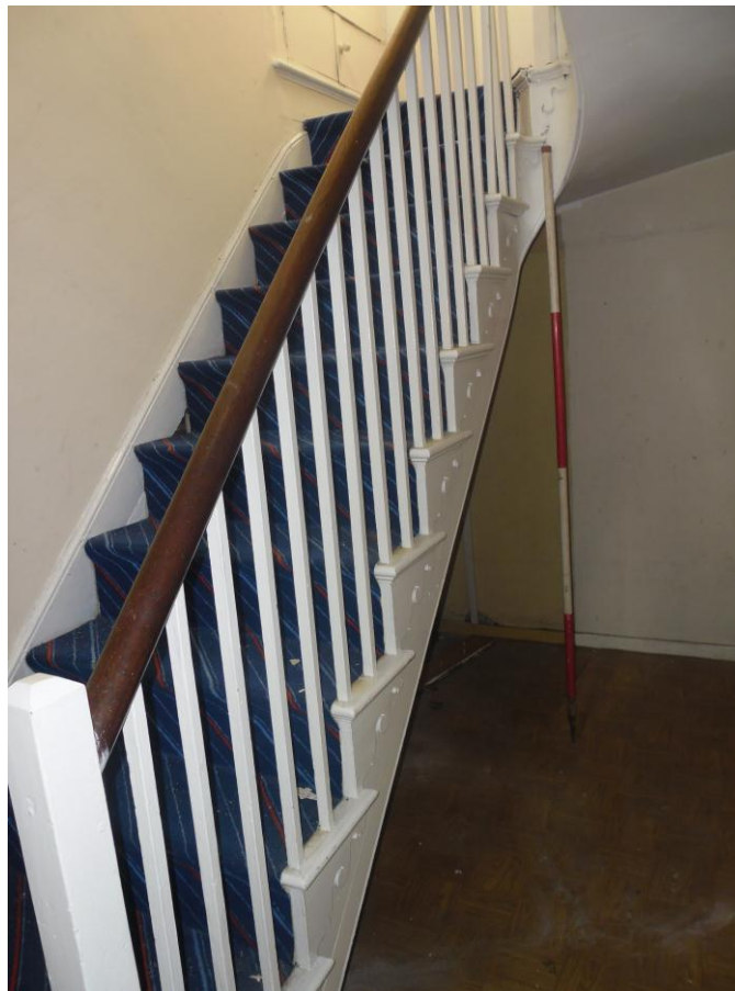
Plate 21: Internal view looking NE showing dog-leg staircase leading from first to second floor with 'Vitruvian Scroll' decoration on brackets to tread ends
