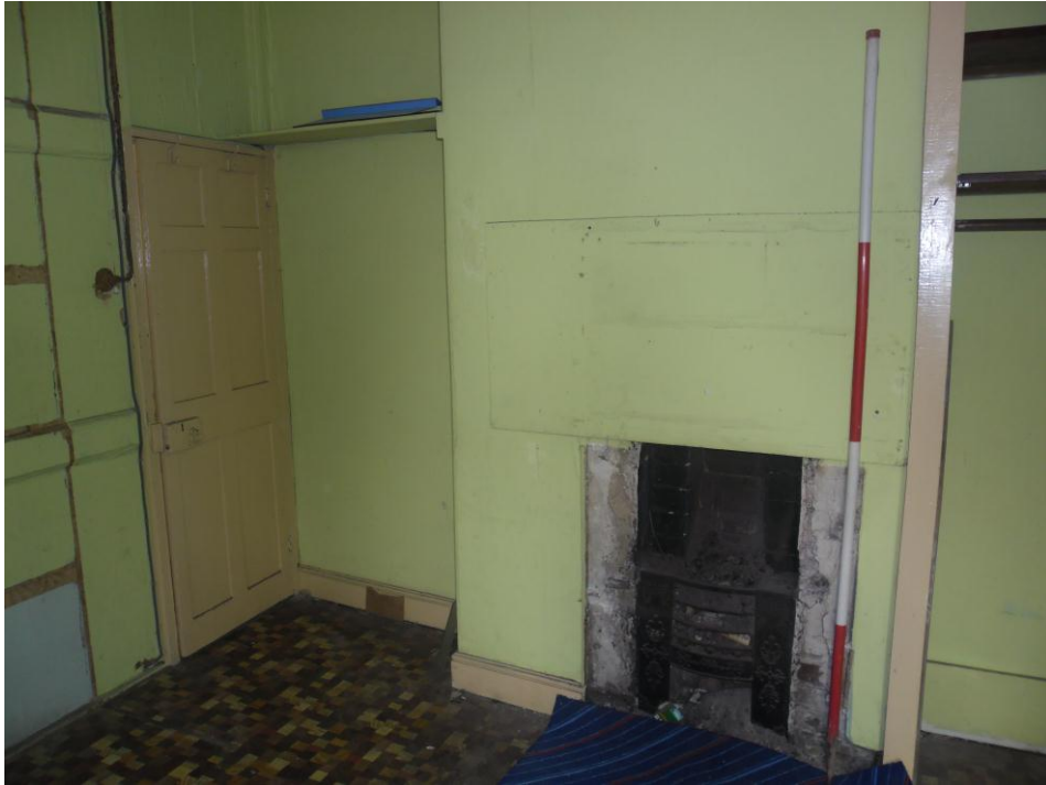
Plate 17: Internal view looking NW showing first-floor room with fireplace (with intact iron grate in the SE-facing wall) flanked by recesses
