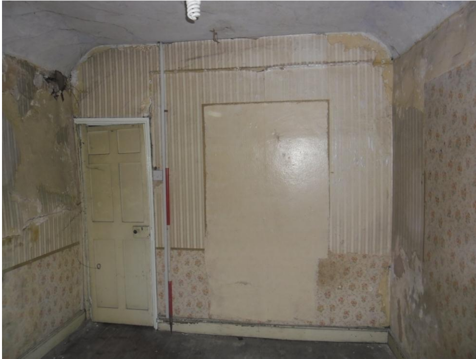
Plate 32: View looking NW showing interior of second-floor room at SE end of corridor
