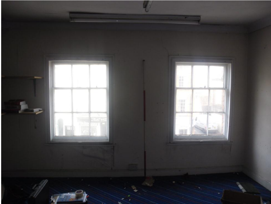
Plate 27: Internal view looking NW showing 9-pane sash windows with reeded architraves in second floor room overlooking Load Street
