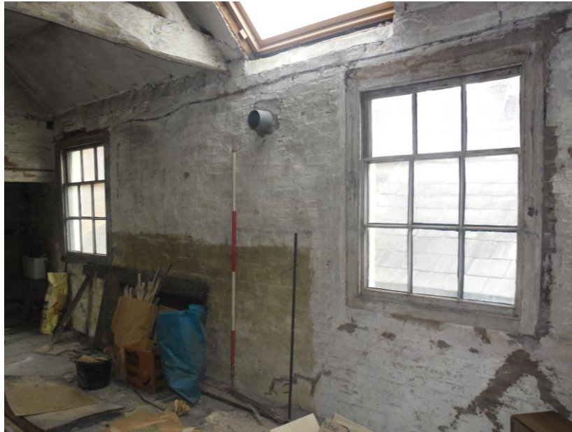
Plate 37: Internal view looking N showing 9-pane sash windows in SW-facing wall
