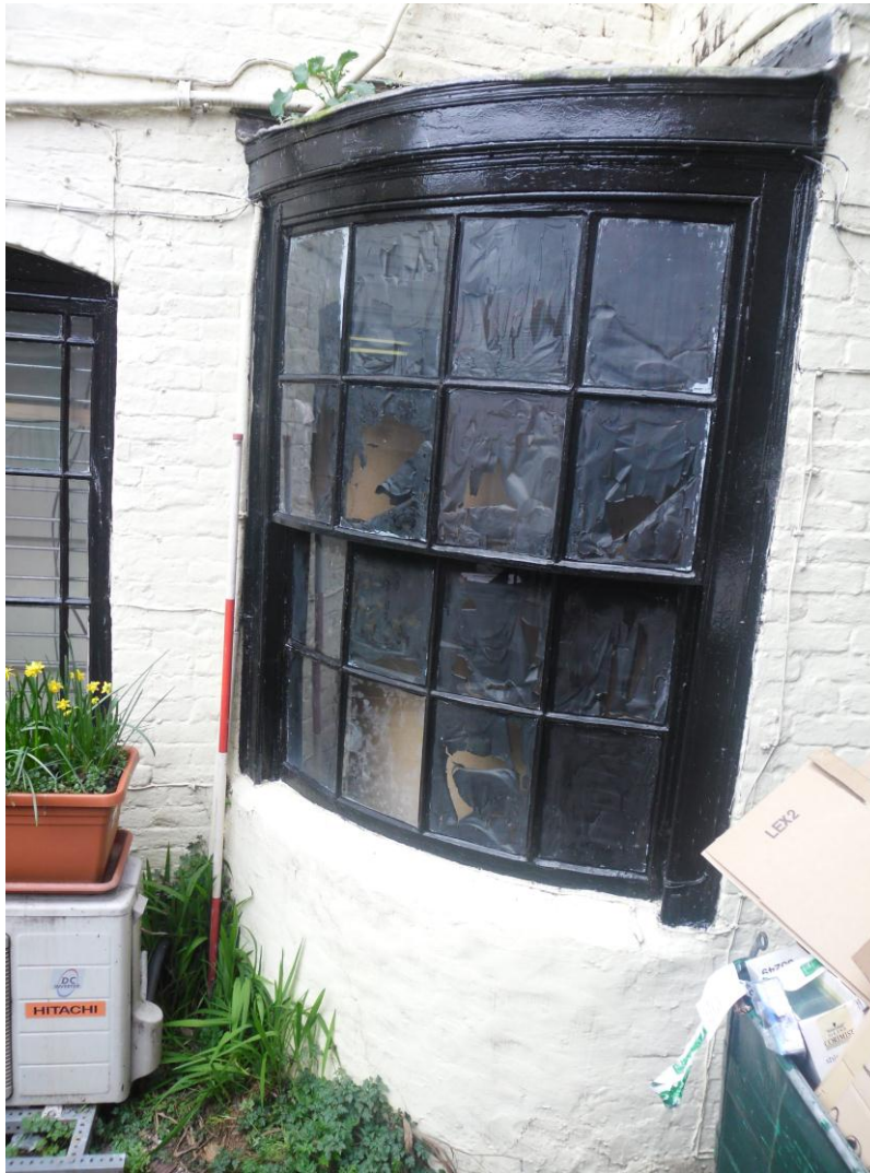
Plate 3: View looking SW showing detail of 16-pane bow window in NE-facing elevation
