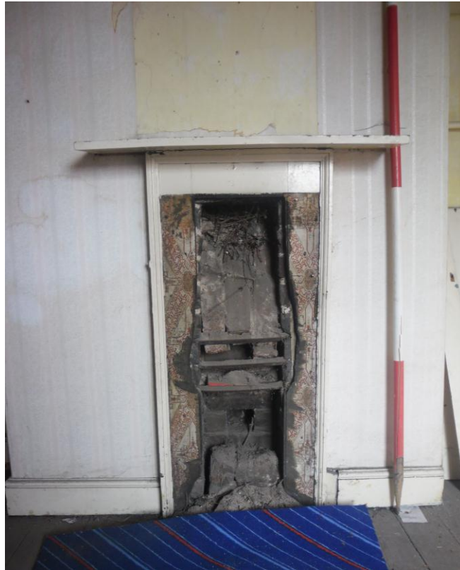
Plate 30: Internal view looking NW showing fireplace in SE-facing wall of second-floor bedroom
