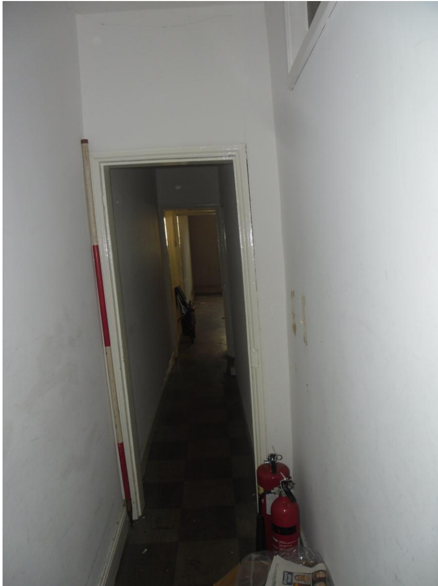
Plate 15: Internal view looking NW along corridor at first-floor level towards staircase to second floor
