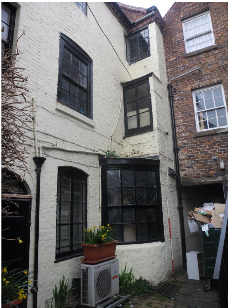
Plate 2: View NW showing NE-facing elevation to the rear of the house, with 16-pane bow window in foreground and casement window above, with cobbled passageway to right
