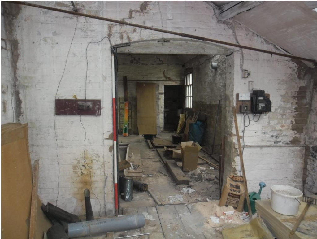
Plate 35: Internal view looking NW showing first floor of two-storey outbuilding (printing works) with segmental-arched door opening
