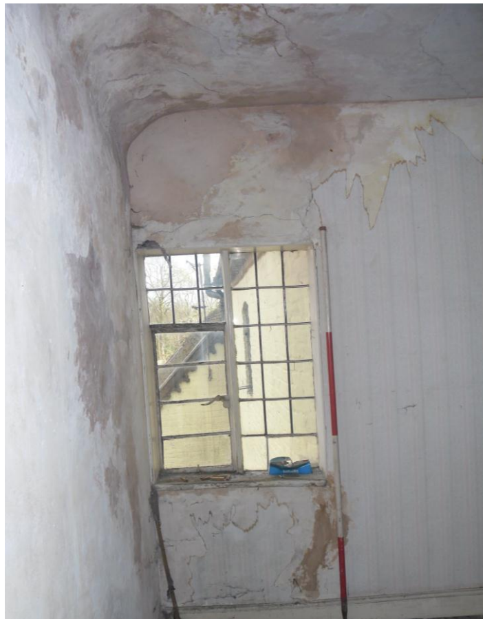
Plate 31: Internal view looking SE showing coved ceiling & casement window in second-floor bedroom
