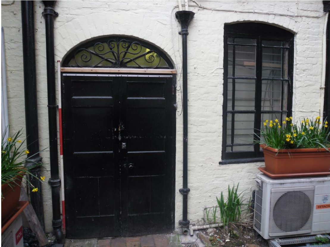
Plate 4: View looking SW showing NE-facing elevation with round-arched doorway and casement window to right
