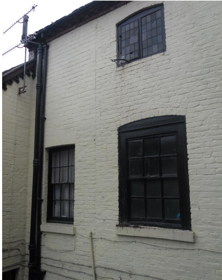
Plate 6: View looking S showing fenestration of NE-facing elevation at first- and second-floor level, with a segmental-arched box-framed sash window and segmental-arched casement window above, and a vertical construction break visible to the left of these windows at first- and second- floor level
