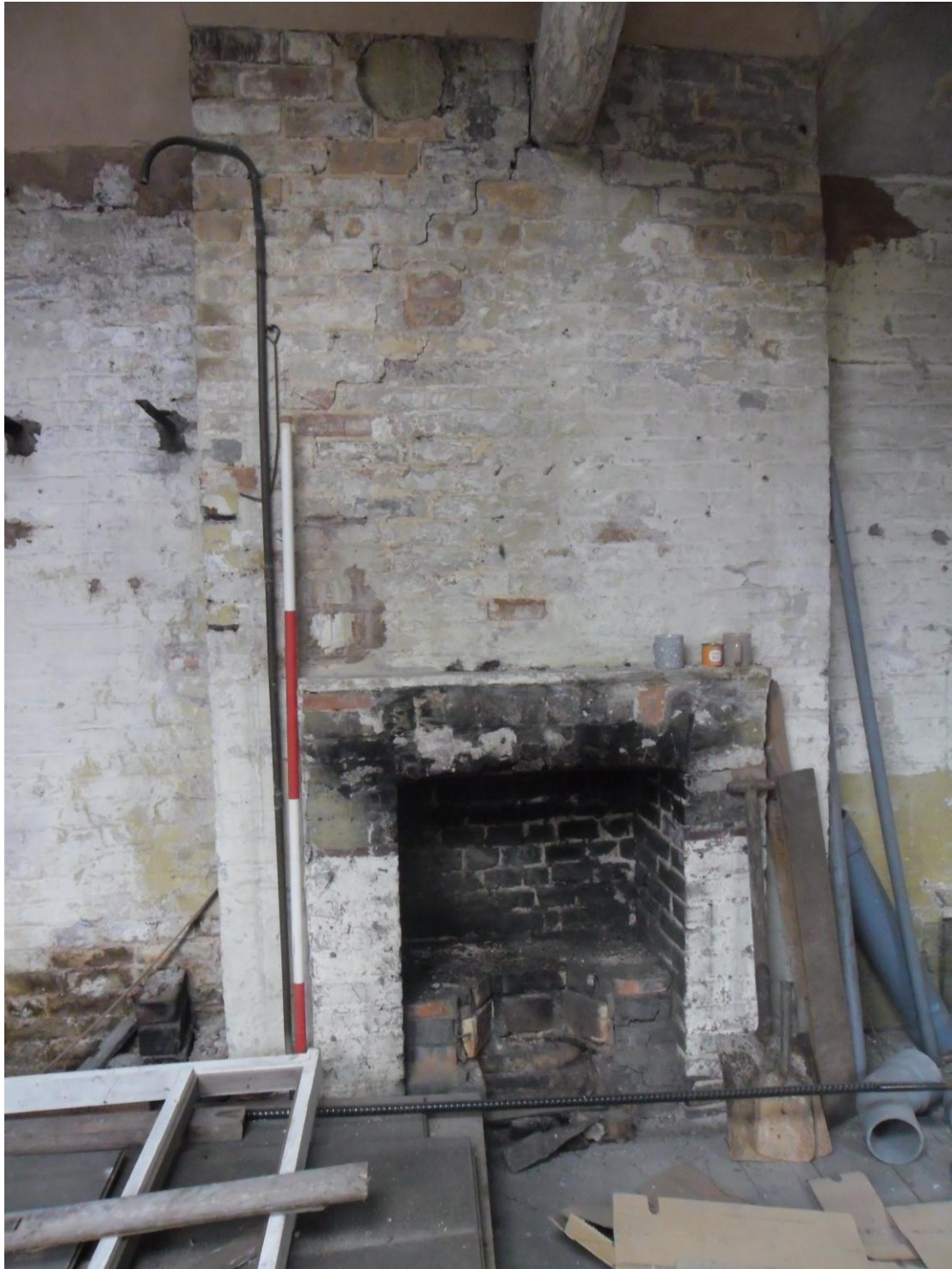
Plate 38: Internal view looking SW showing fireplace in NE-facing wall
