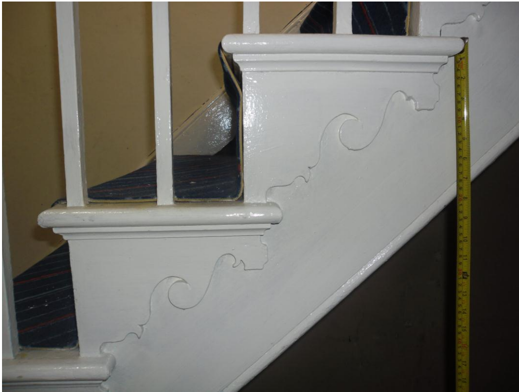
Plate 22: Detail showing plain 'Vitruvian Scroll' detailing of brackets to tread ends of dog-leg staircase to second floor
