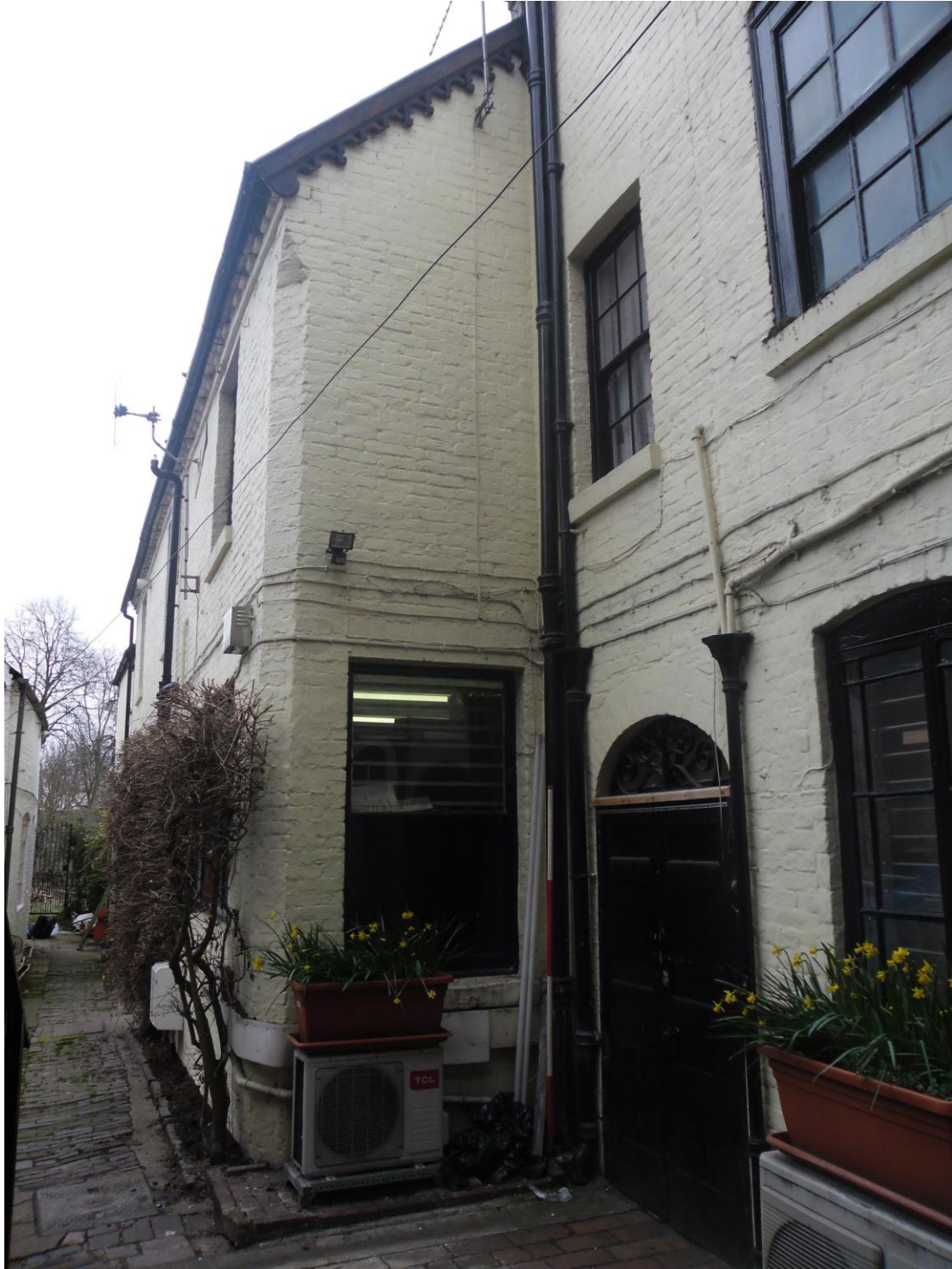
Plate 9: View SE showing NW-facing gable elevation of printing works with ornate scrollwork decoration at eaves level
