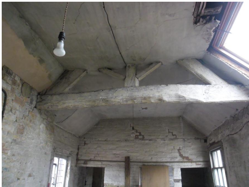
Plate 36: Internal view looking NW showing kingpost roof truss (partially concealed by a coved plaster ceiling) in central compartment of printing works/workshop
