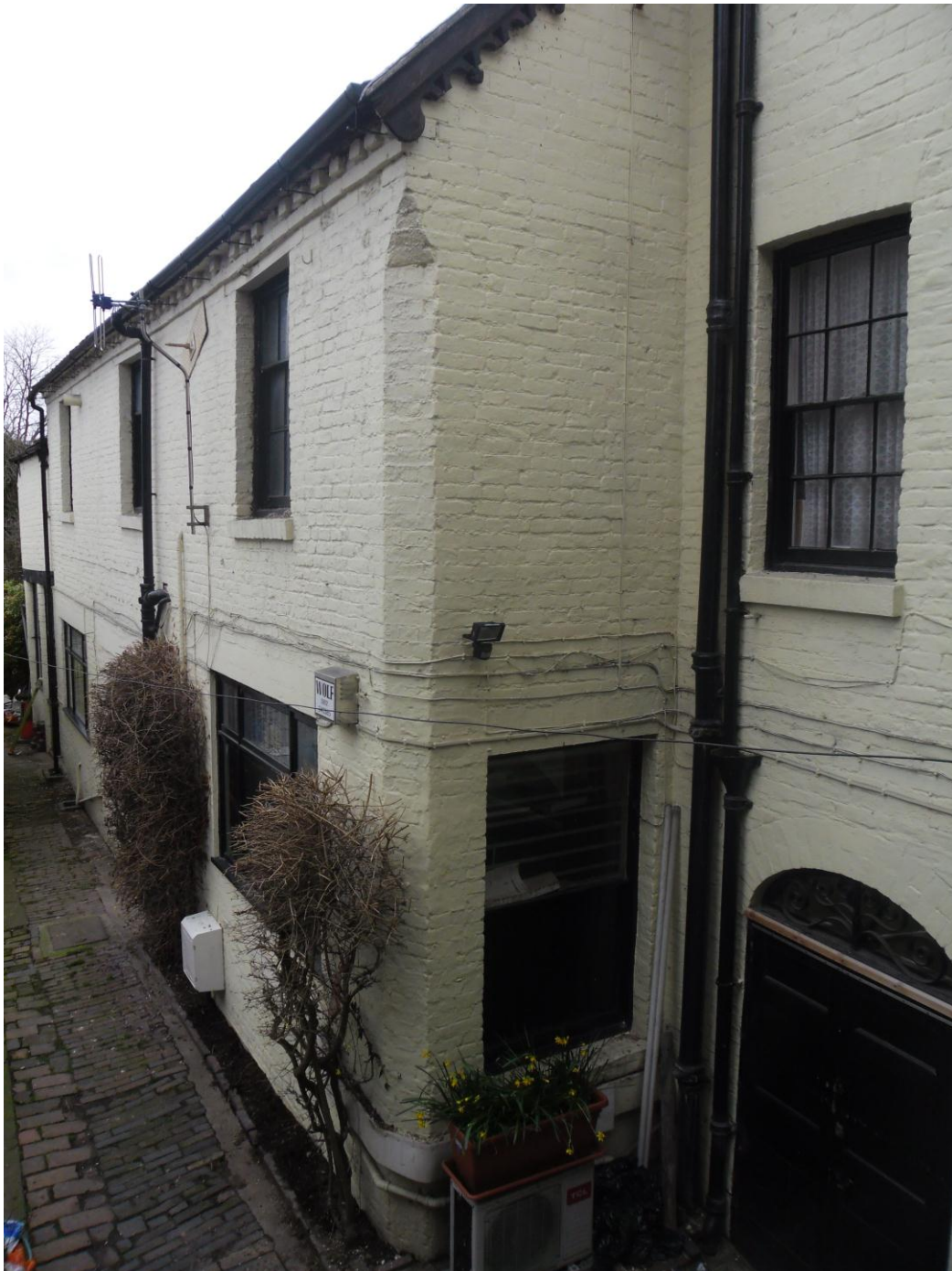
Plate 8: View looking SSE showing NE-facing elevation of printing works with dentilled eaves cornice and chamfer at the NW gable end of the building
