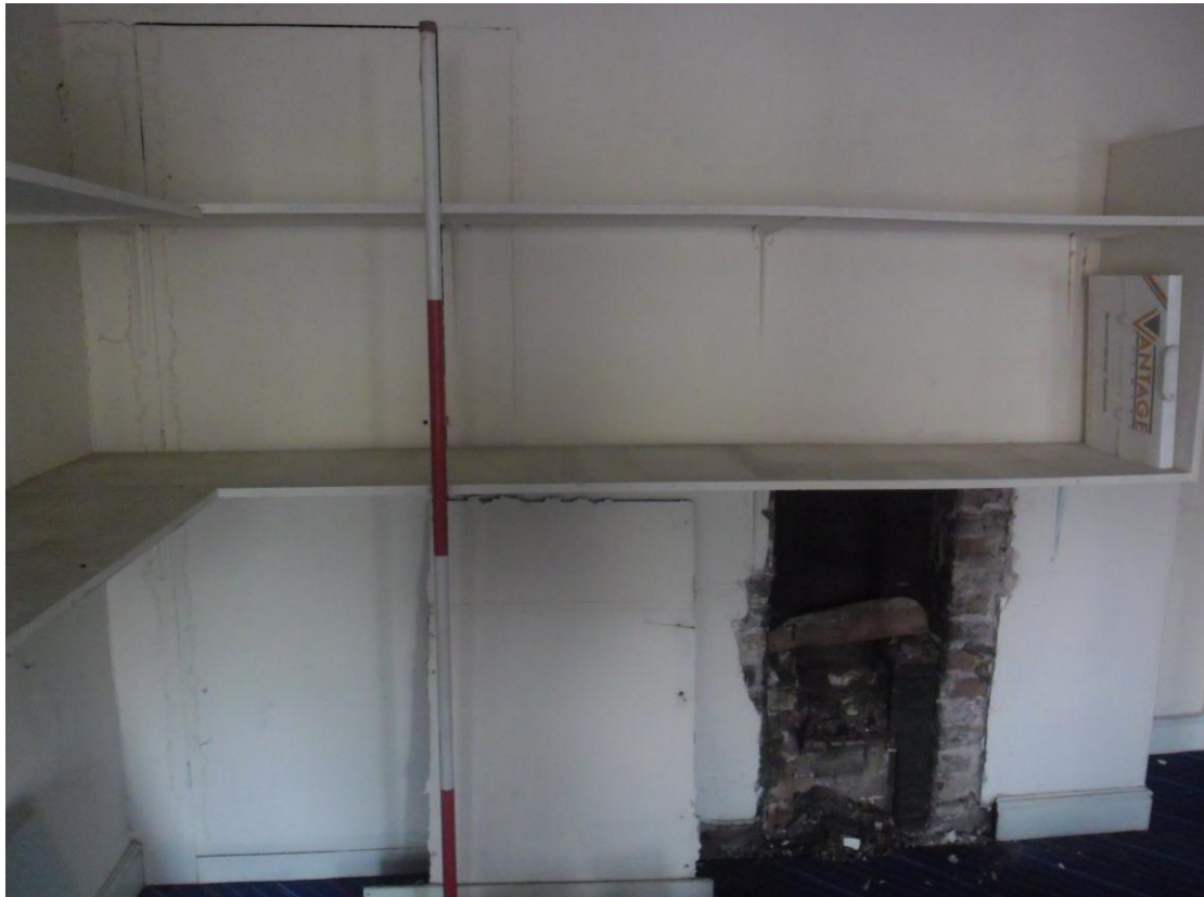
Plate 29: Internal view looking SE showing fireplace and blocked-up doorway in second-floor room overlooking Load Street
