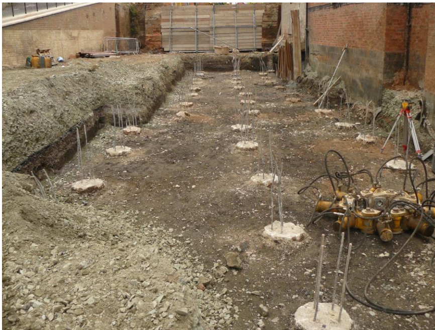
Plate 2: View N of piling for access-road construction
