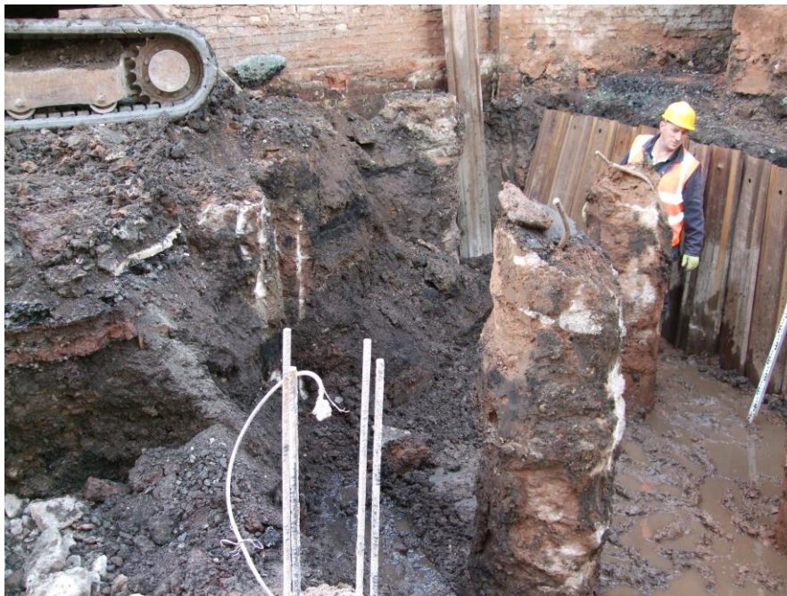
Plate 1: View NW showing groundworks in progress to S of Town Wall
