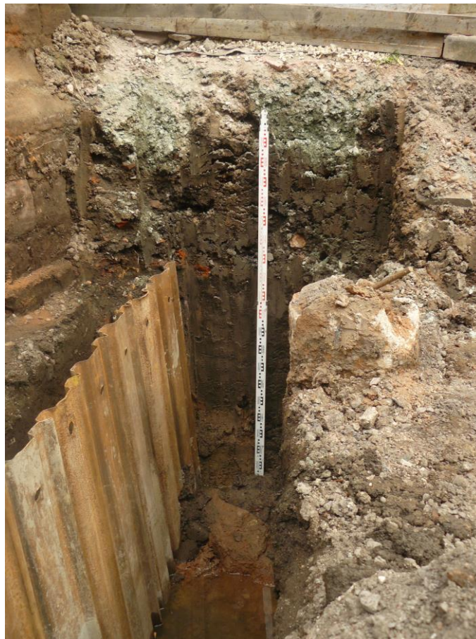
Plate 3: View NE showing deposits revealed adjacent to the southern elevation of the Town Wall
