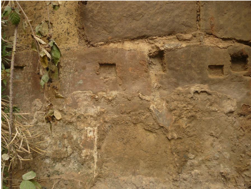
Plate 6: Regular indentations on S elevation of the Town Wall
