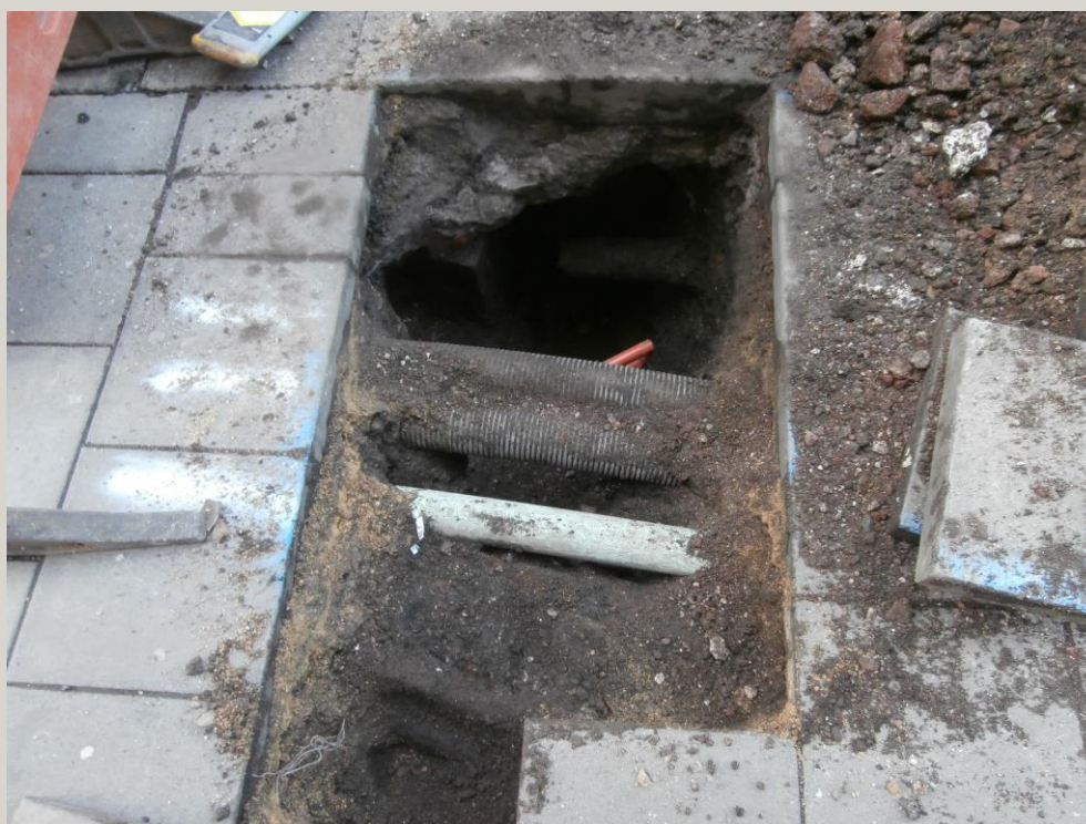
Plate 15: View to the W of Trench 8
