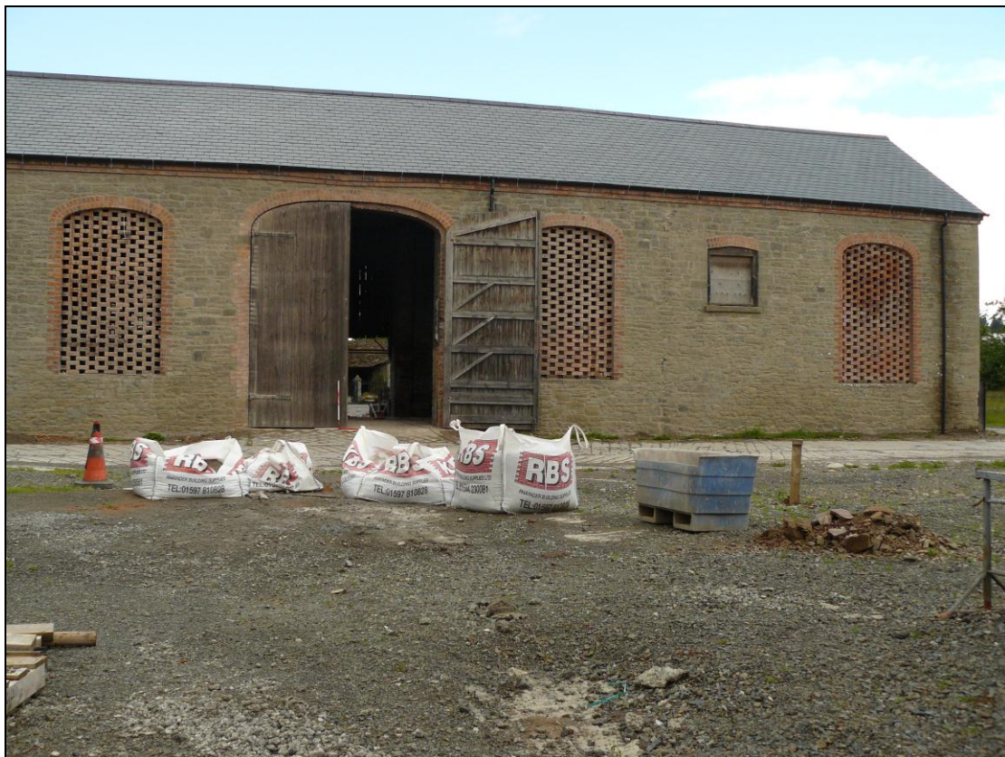
Plate 2: View looking SW showing rear (NE facing) elevation of threshing barn (Building 1) with doorway flanked by chequerboard patterned ventilation windows
