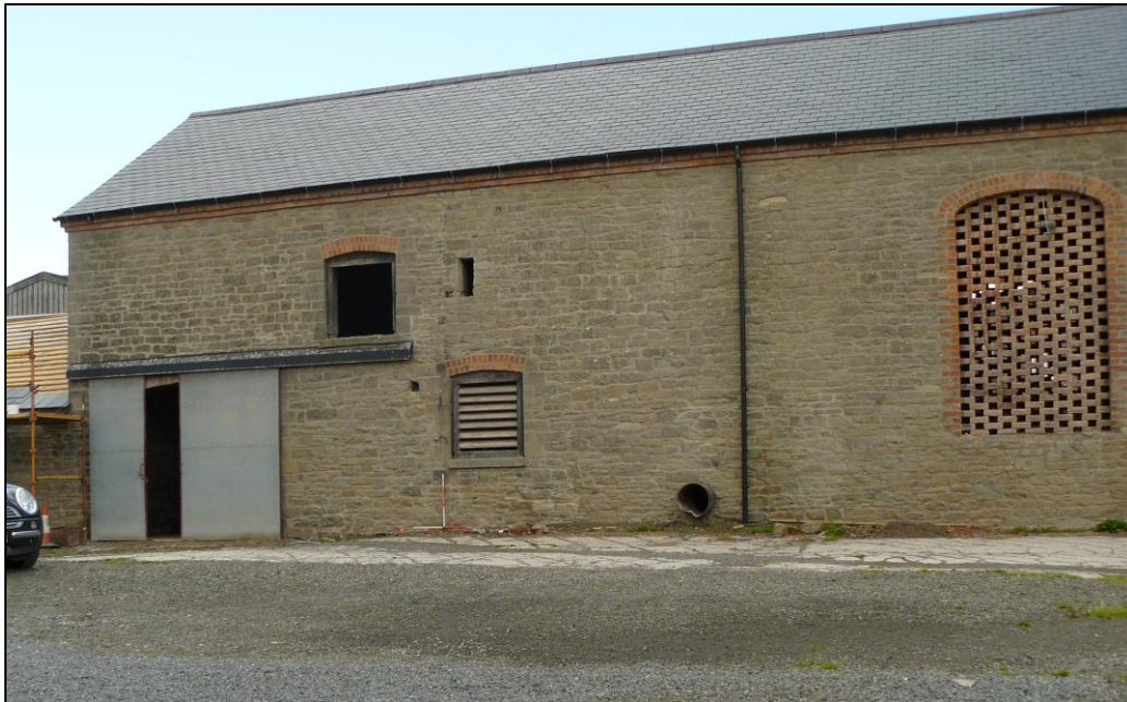
Plate 4: View looking SW showing SE end of rear (NE-facing) elevation of Building 1 with segmental arched doorway (concealed by modern sliding doors and fascia) with loading bay above
