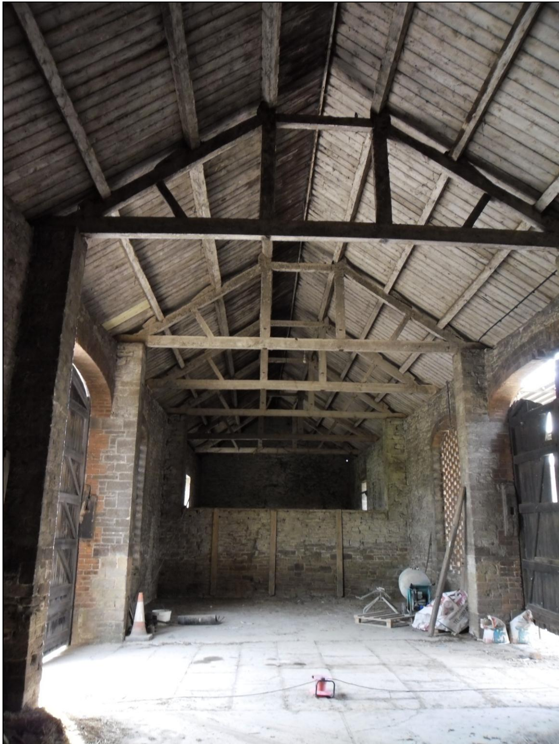
Plate 3: Internal view of threshing barn (Building 1) looking SE showing queen-post roof trusses and stone-flagged threshing floor in central bay, with stone partition wall in background
