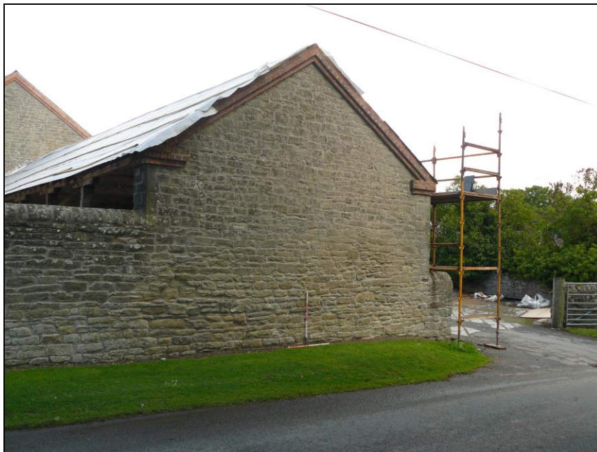
Plate 16: View looking NW showing SE end of Building 4 with pedimented gable and brick cornice
