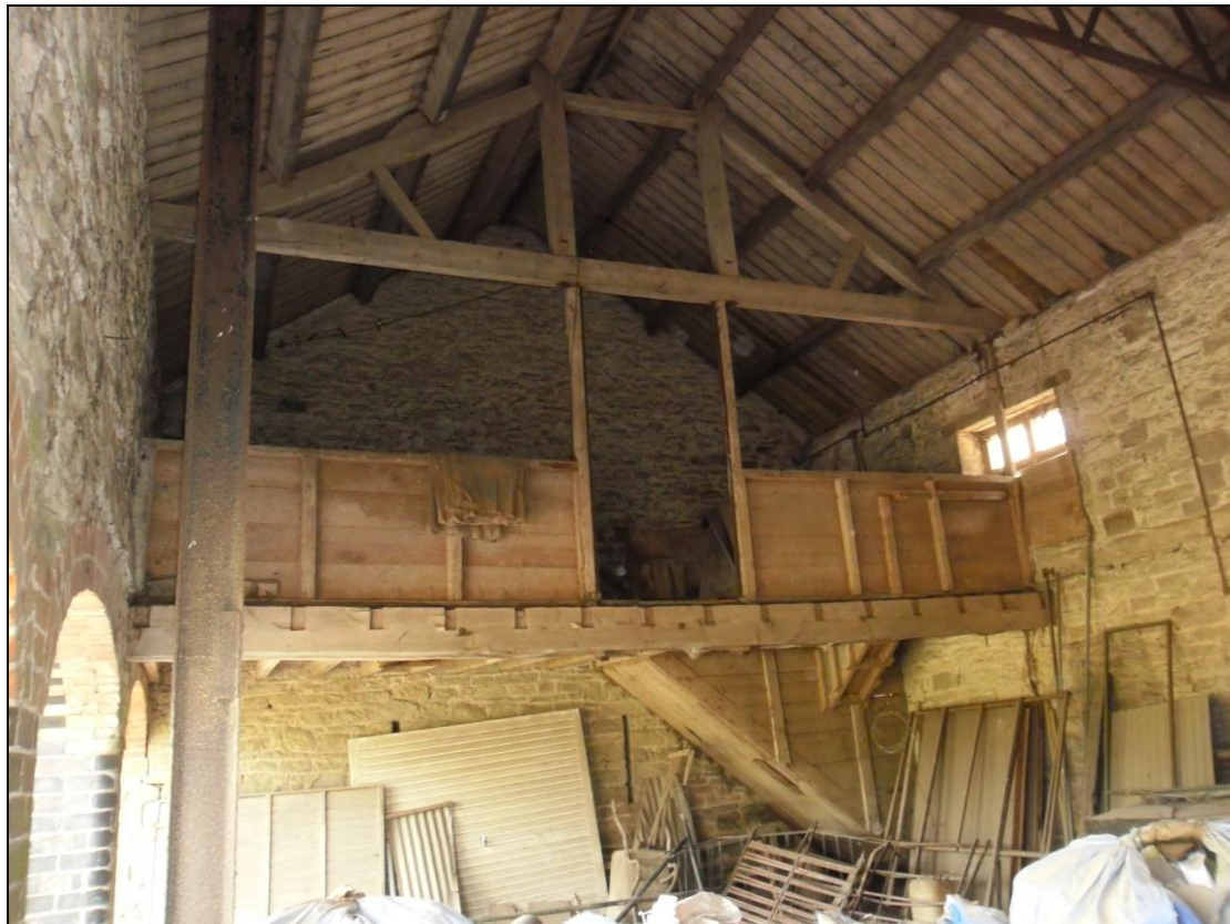
Plate 9: Internal view of cartshed and granary in Building 2 showing queen-post roof construction
