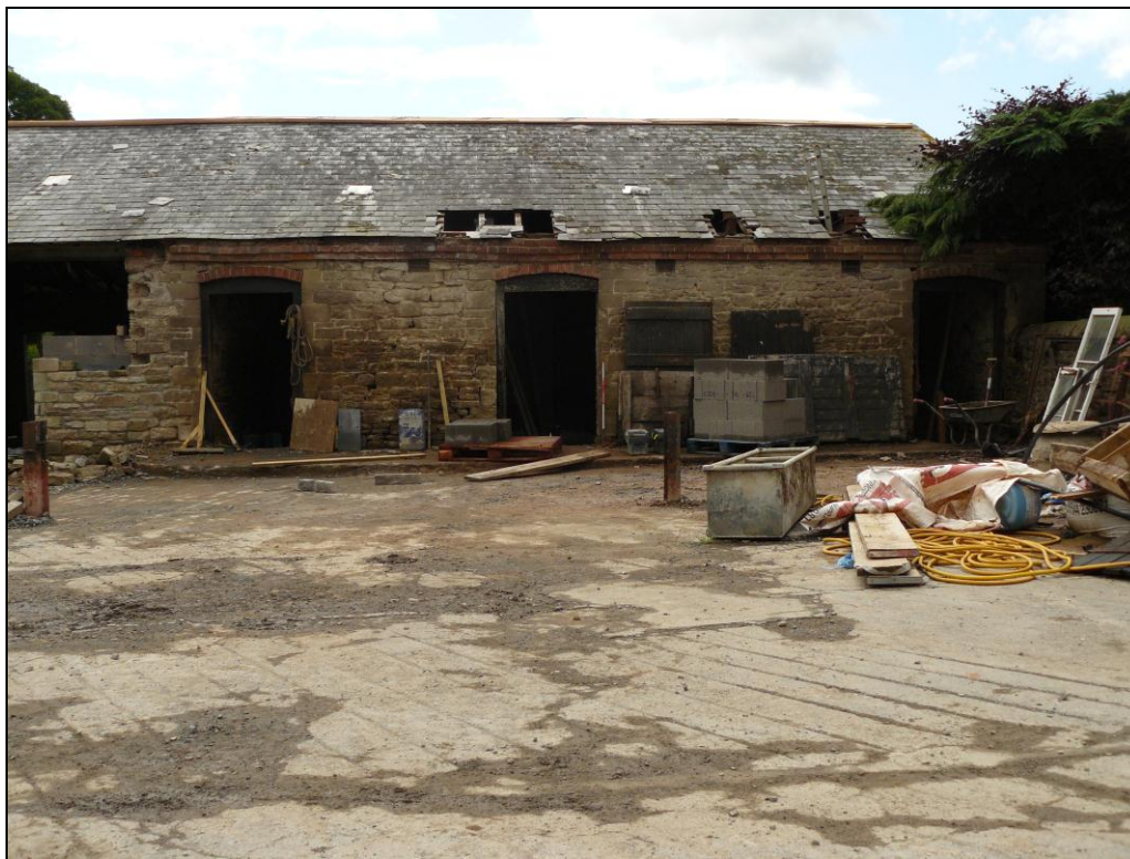
Plate 13: View looking SE showing the three bays at the SW end of Building 3 with brick segmental arched doorways and stepped brick eaves cornice
