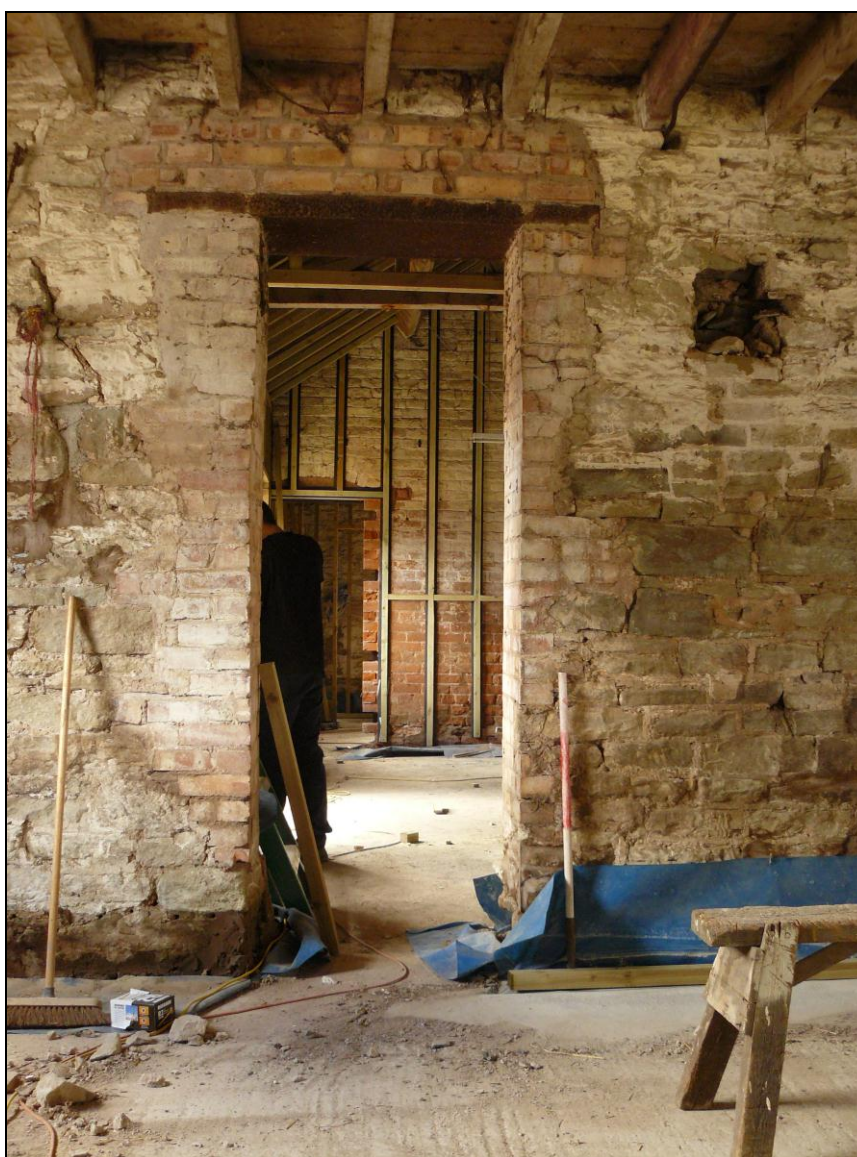
Plate 10: Internal view of Building 2 looking SW showing modern doorway with brick surround inserted into wall of two storey stable and hayloft
