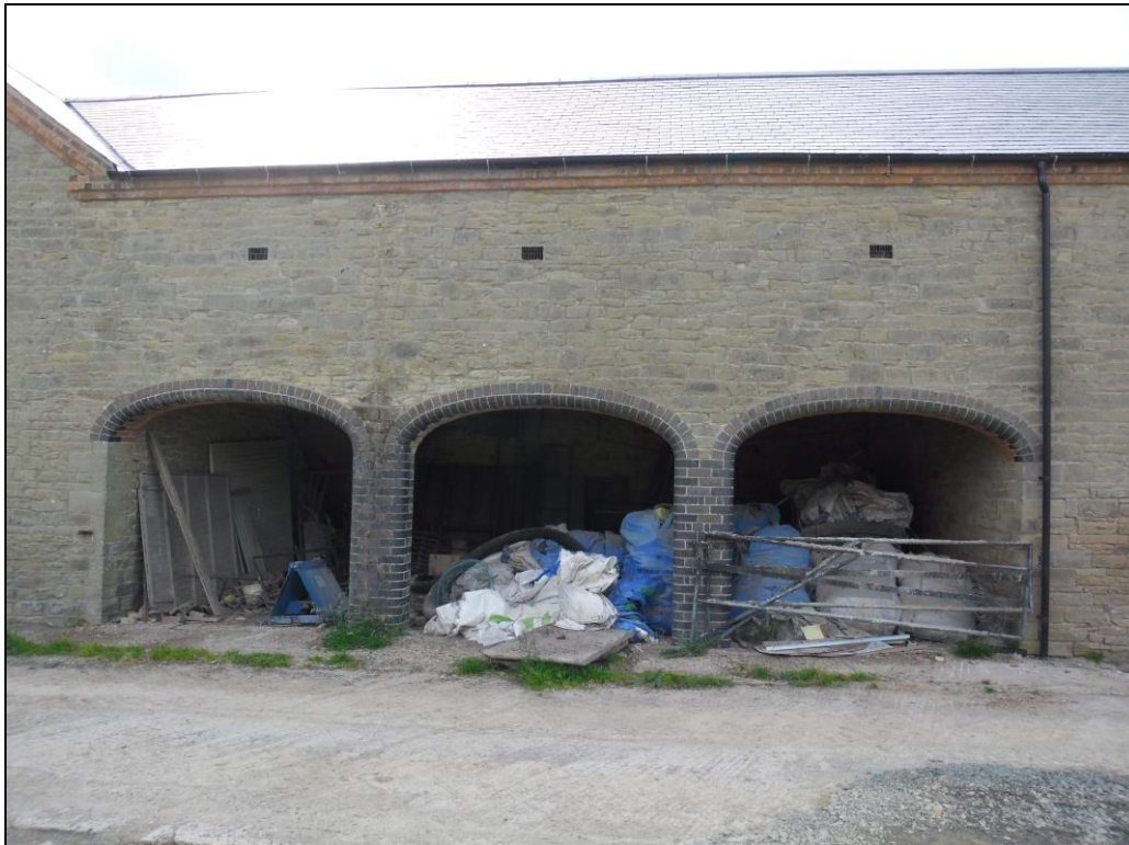
Plate 7: View looking SE showing rear (NW-facing) elevation of Building 2 showing broad arches for cartshed with ventilation grilles for granary at first floor level
