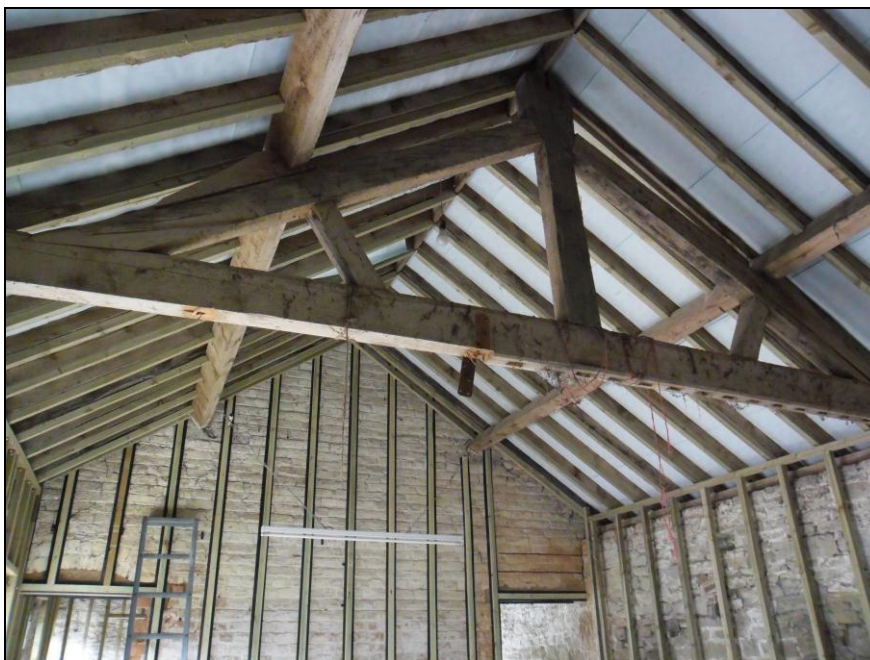
Plate 12: Internal view looking SW showing detail of king-post roof construction and brick partition wall in single storey stable block at SW end of Building 2
