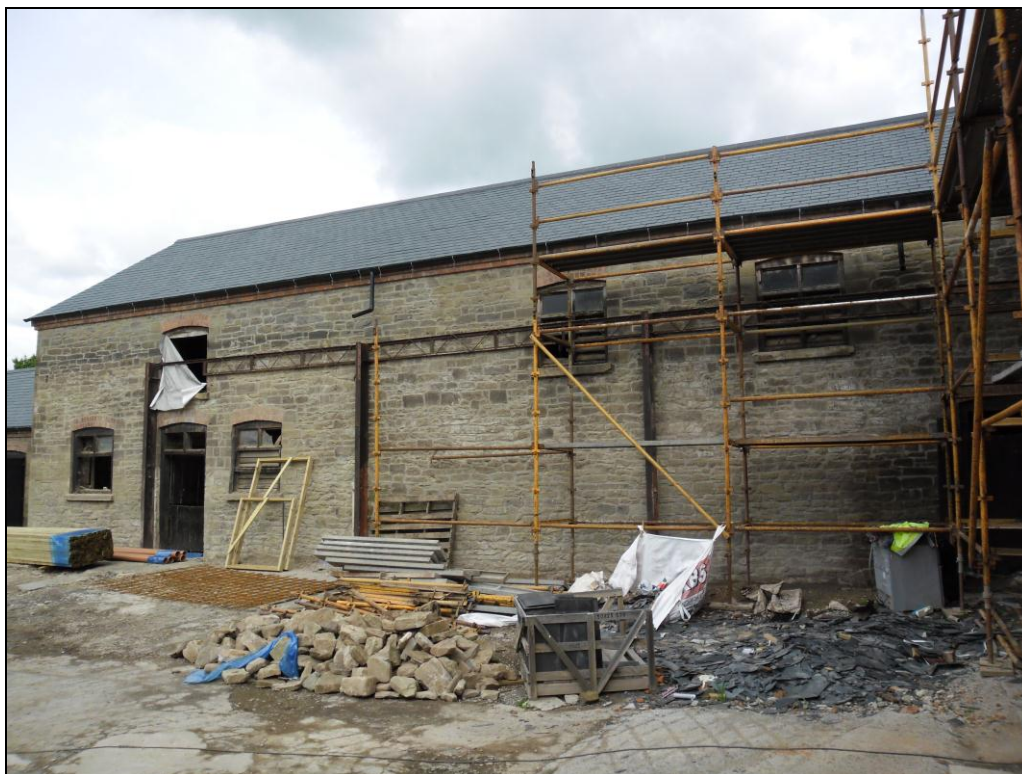
Plate 8: View looking NW showing SE-facing elevation of Building 2 with stable and hayloft to left and granary building (with segmental arched windows at first floor level) to right
