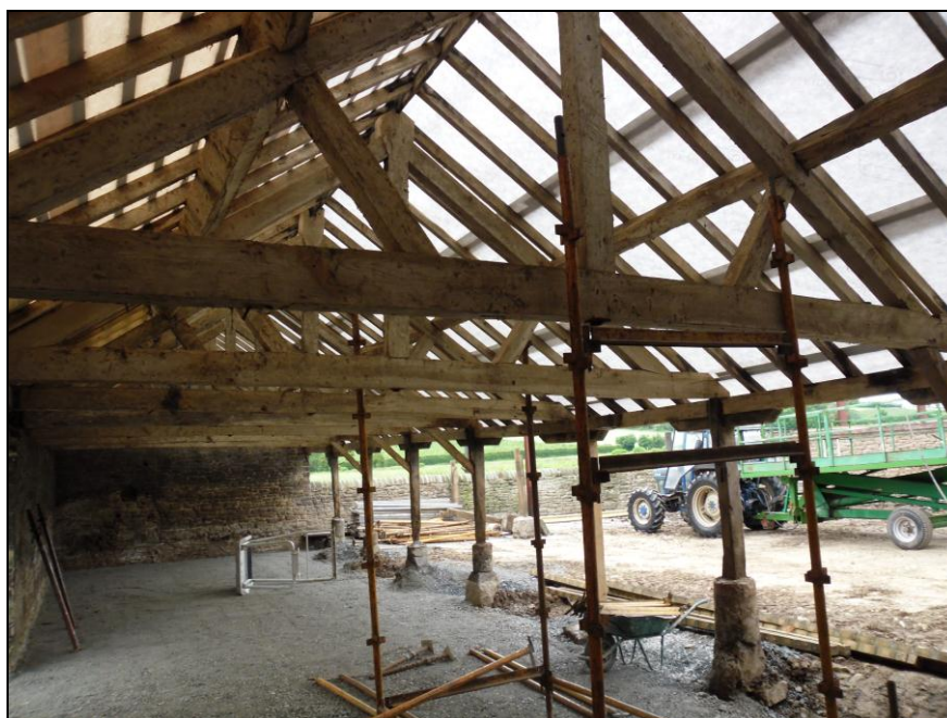
Plate 17: View looking SE of Building 4 showing king-post roof construction
