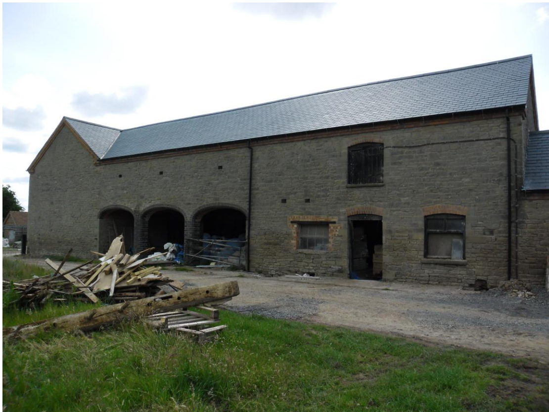
Plate 6: View looking E showing rear (NW facing) elevation of Building 2 with cartshed and granary to left and stable and hayloft (with loading bay window) to right
