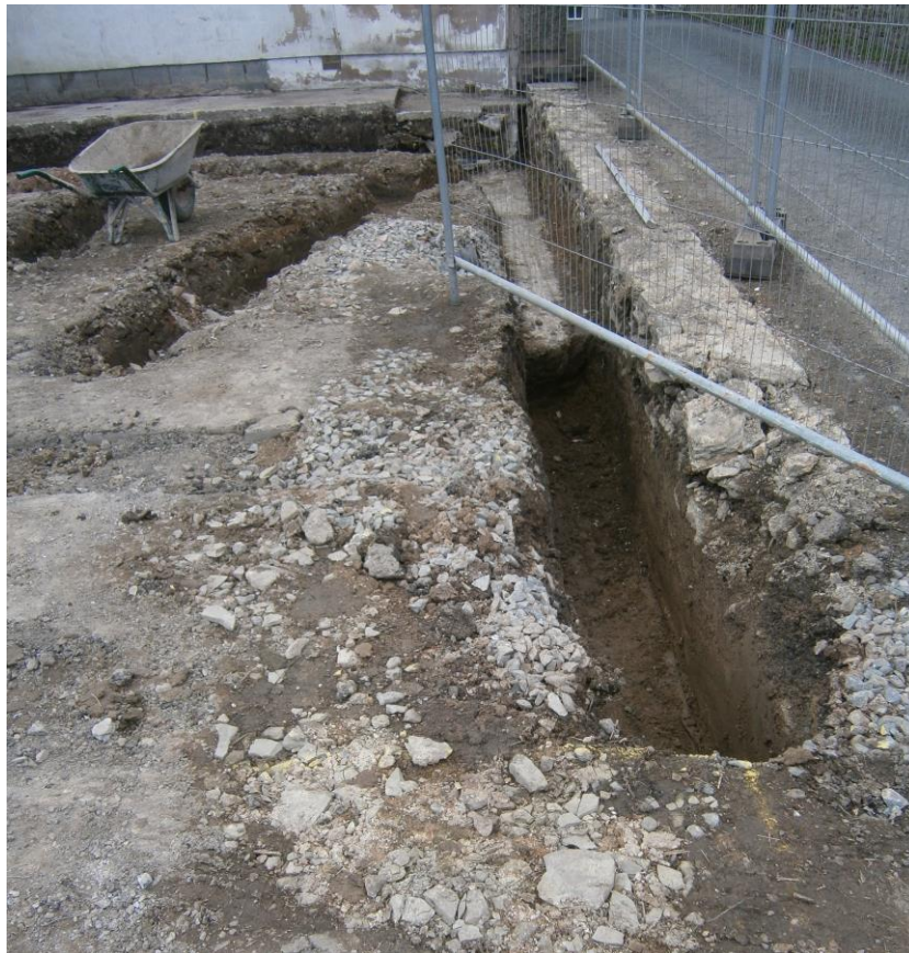
Plate 1: View W showing the scar of the 2010 evaluation trench reflecting the position of the W/E foundation trench.
