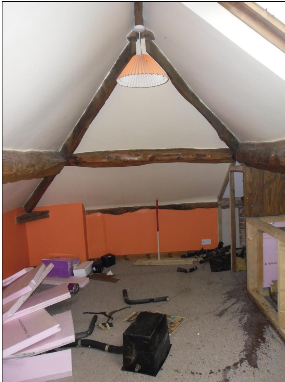
Plate 7: Internal view looking NW showing detail of collar truss roof construction in attic
