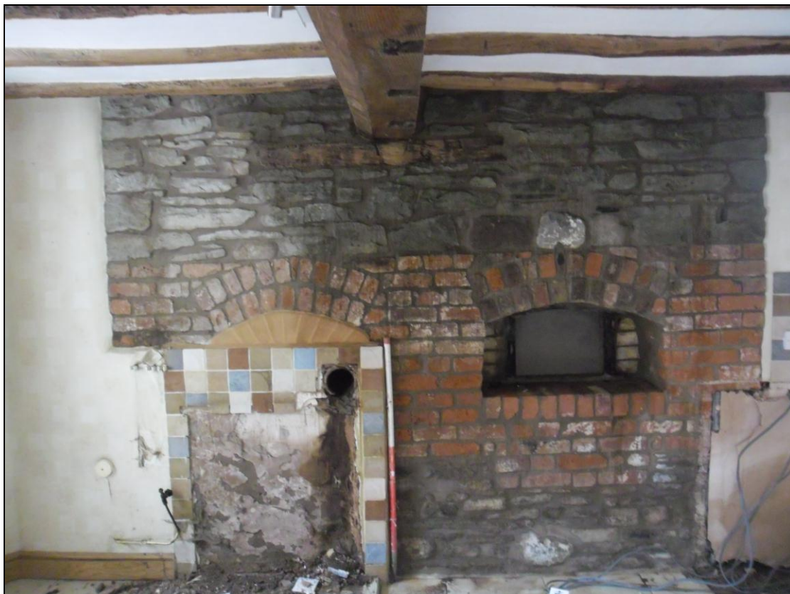
Plate 8: Internal view looking NE showing blocked up segmental brick fireplace and adjacent oven in rear extension (kitchen)
