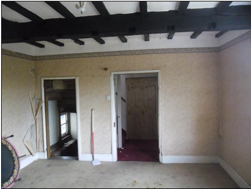
Plate 4: Internal view of living room looking SE showing exposed ceiling beam with mortice slots and doorways to hallway and cellar (to left)
