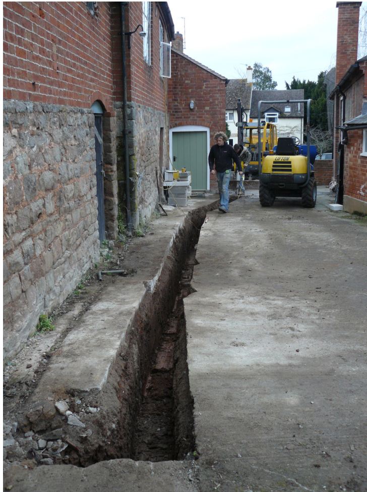
Plate 1: View SW showing extent of trenching
