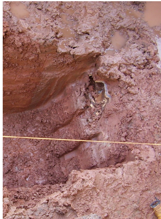
Plate 7: Ceramic drain found in trenching to E of public house: view E
