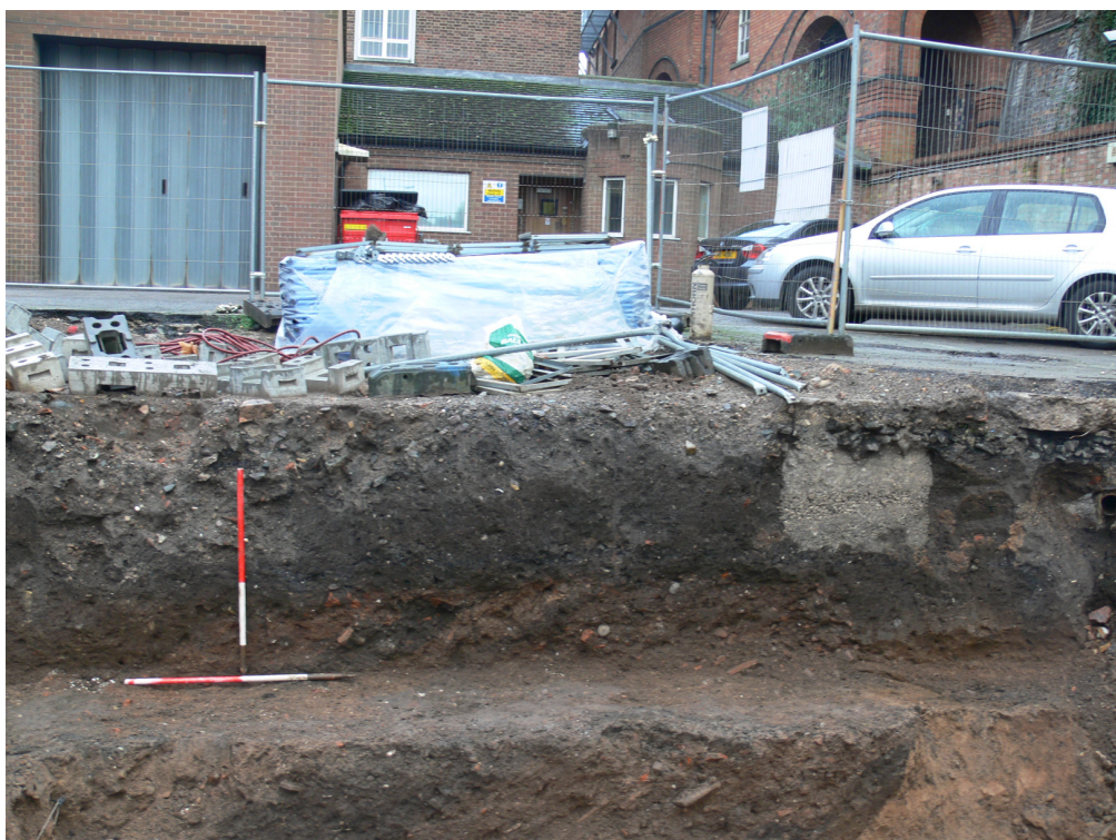
Plate 1: View W showing deposits excavated during initial groundworks
