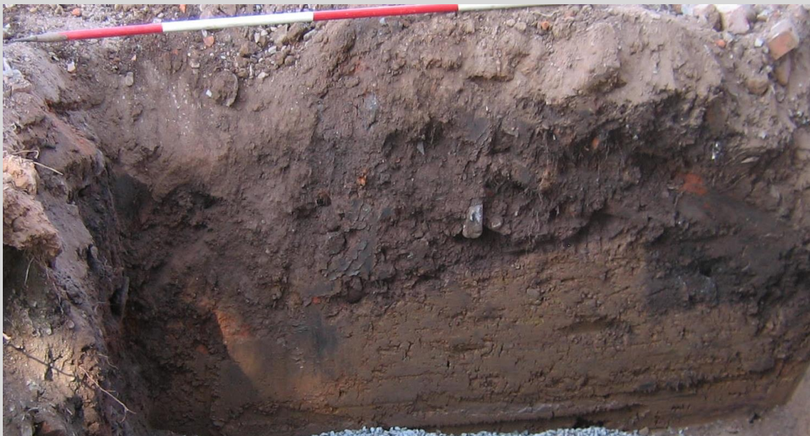
Plate 12: View east of section on east-facing wall of Manhole 3 showing a continuation of the floor seen in Plate 11, which suggests that it too was contemporary with the kilns. This floor has a step [218]. The yellow layer is (217), the dark demolition layer above it (219) and the overlying layer (220)
