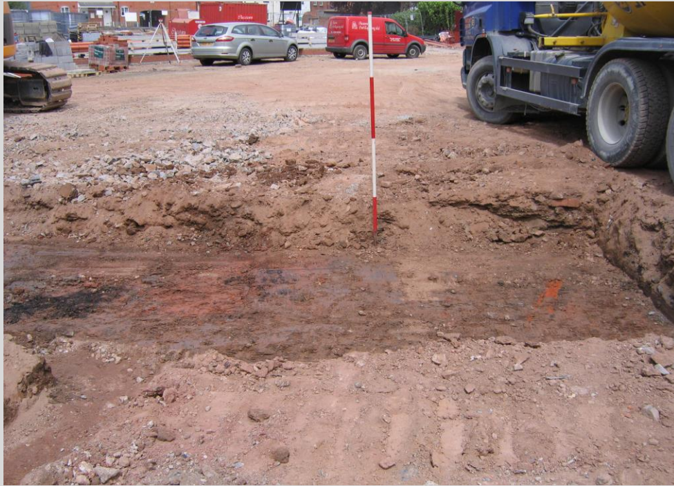
Plate 15: Structures in the porch area on the north side of Trench 25. The brick wall on the right is fill (259) in cut [260]. The burnt area on the left is fill (262) in cut [263] which is cut into demolition layer spread (264). The trench is about 0.5m deep and the photograph is facing northeast.
