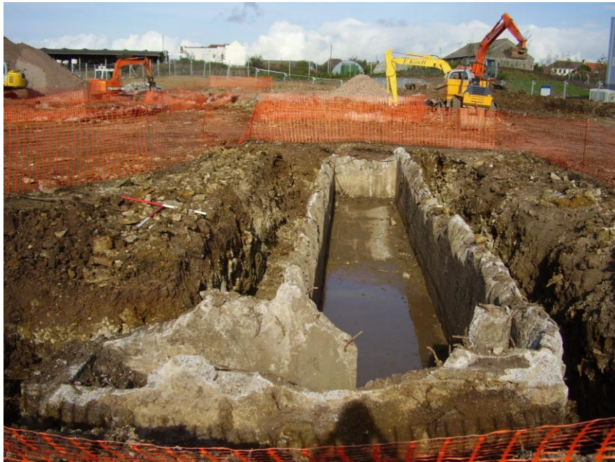
Plate 3: Air-raid Shelter 3, facing NW
