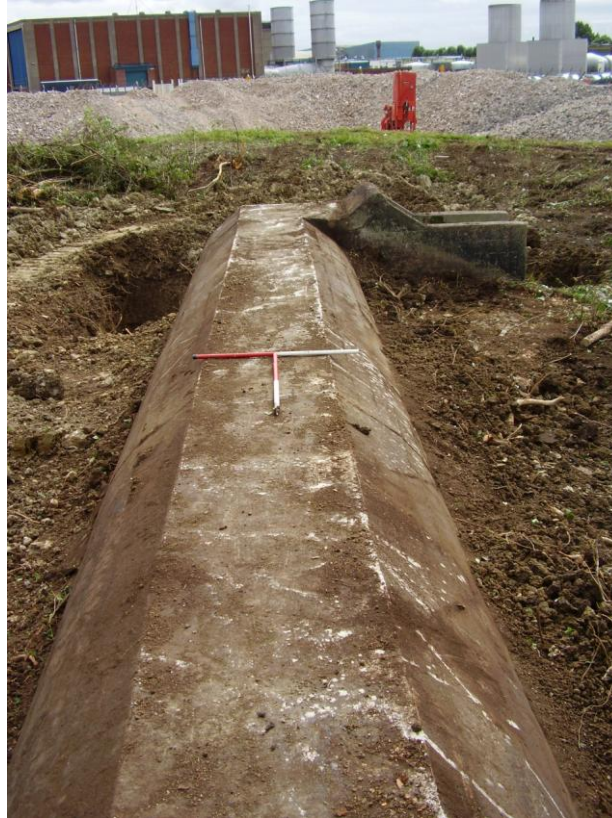
Plate 6: View E showing roof construction
