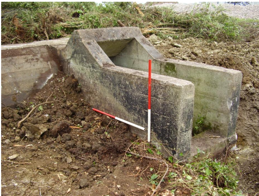
Plate 5: View NE showing entrance construction
