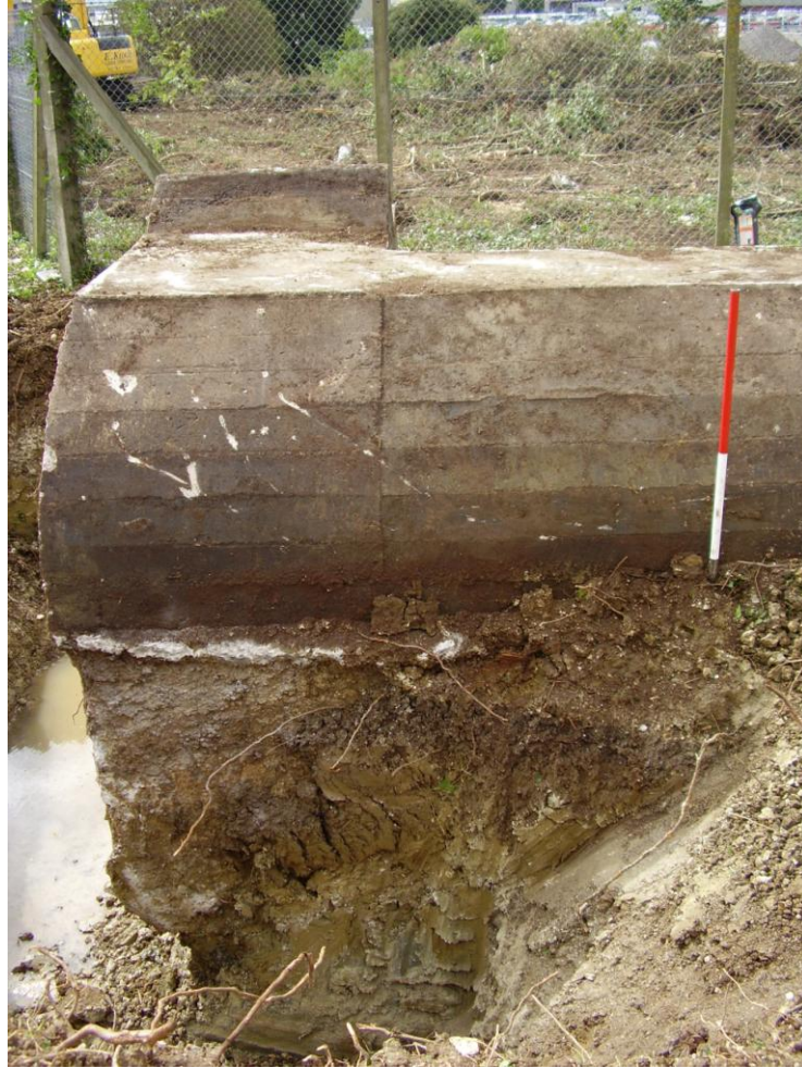
Plate 4: View S showing construction
