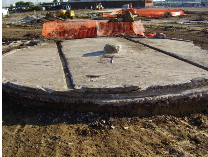
Plate 18: Western filter bed (306), facing SE
