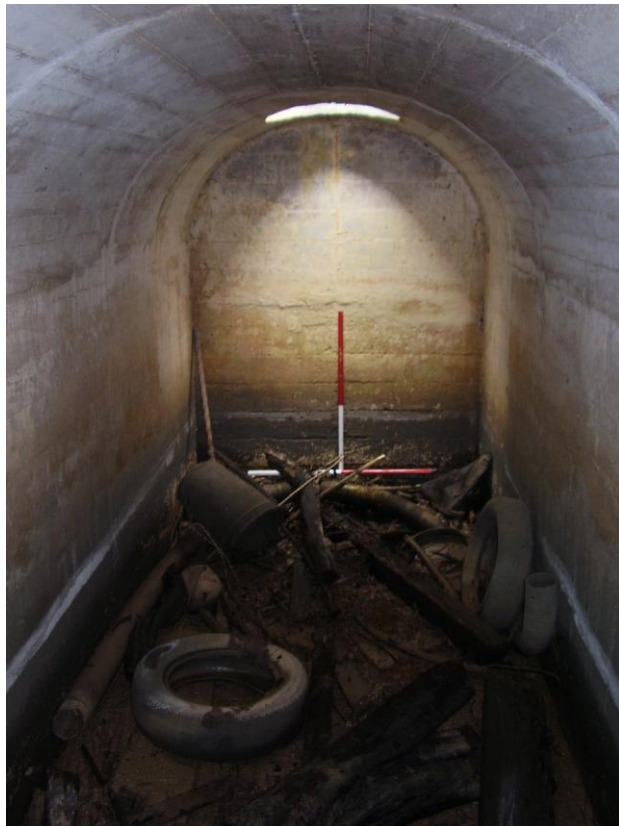
Plate 10: Interior view, looking W, showing vent in roof and internal debris
