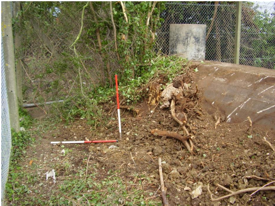
Plate 2: View NW showing location of vent
