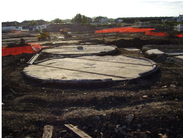
Plate 16: View SW showing filter beds
