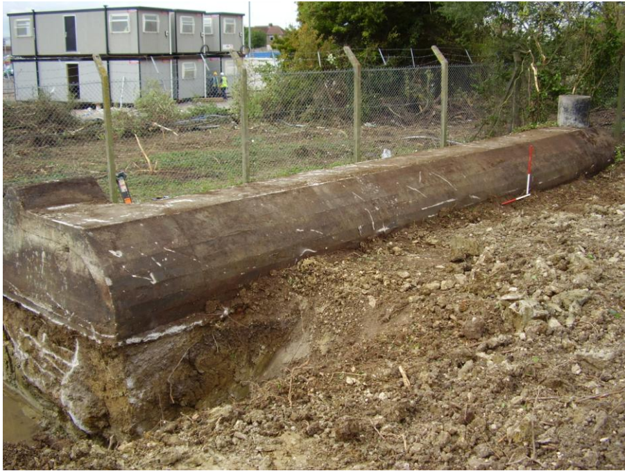
Plate 1: View SW showing external construction of shelter
