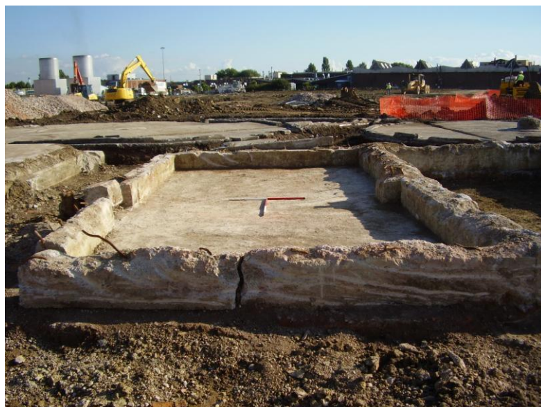
Plate 21: View SE showing holding tank remains (318)
