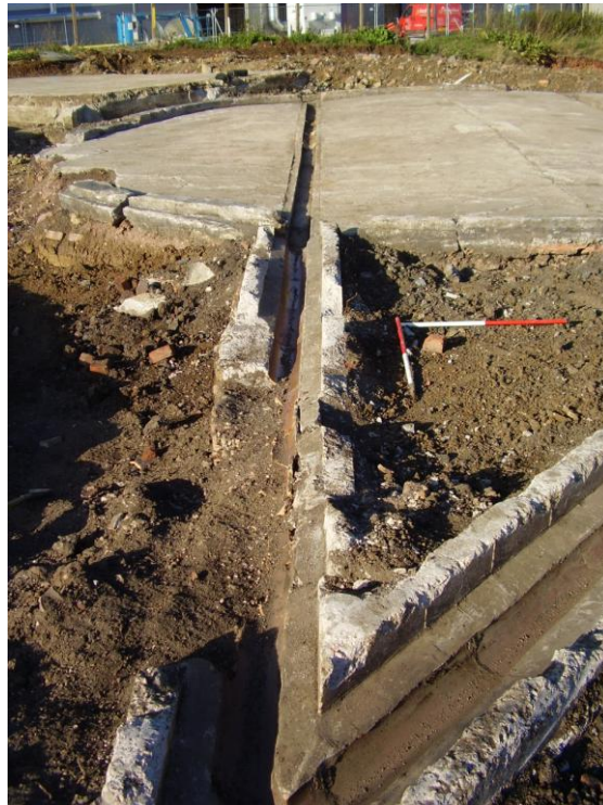
Plate 19: Concrete drains (314), facing NE/E
