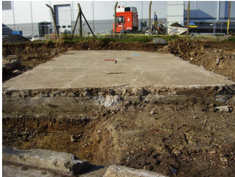
Plate 20: View NW showing concrete platform / holding tank (315)
