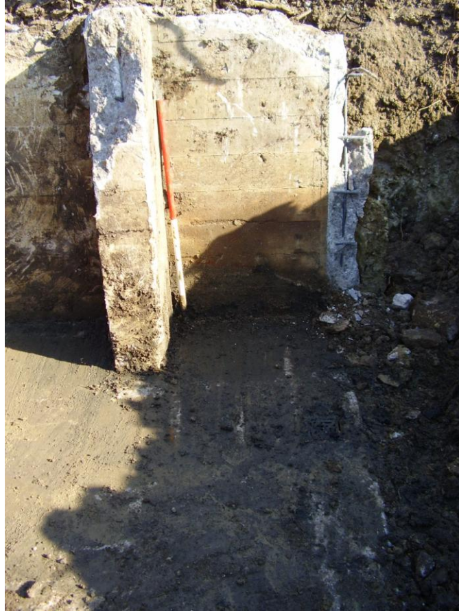
Plate 2: Air-raid Shelter 2 – Entrance. Facing NE
