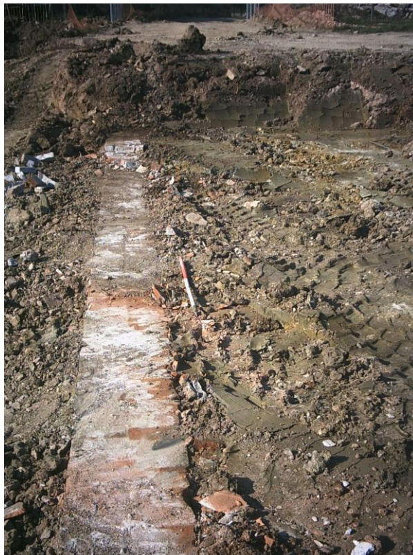
Plate 20: Brick Wall (017). Facing N.
