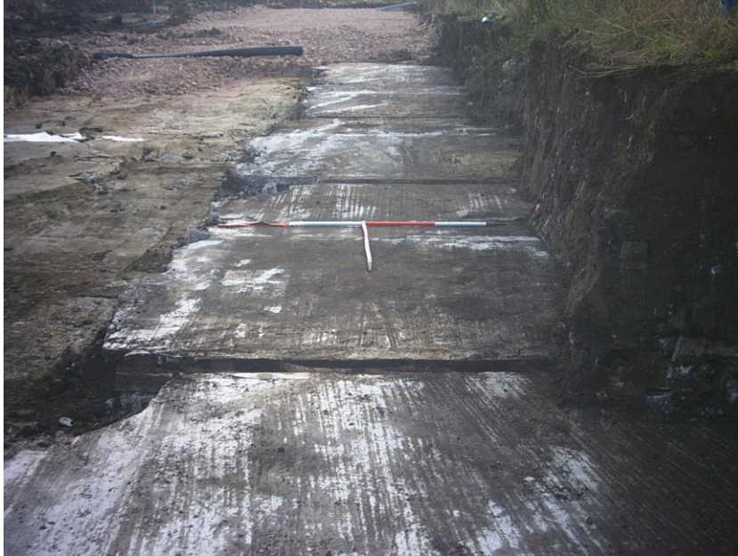
Plate 11: Concrete surface adjacent to central part of N-facing section. To left of picture the concrete has been cut to insert a utility trench. Facing E.
