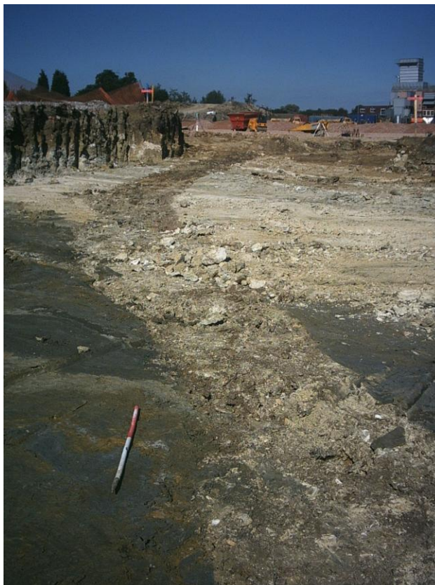
Plate 8: Utility cut [026] and fill and recurrence of slate/shale geology in SW 'turning' area, facing N
