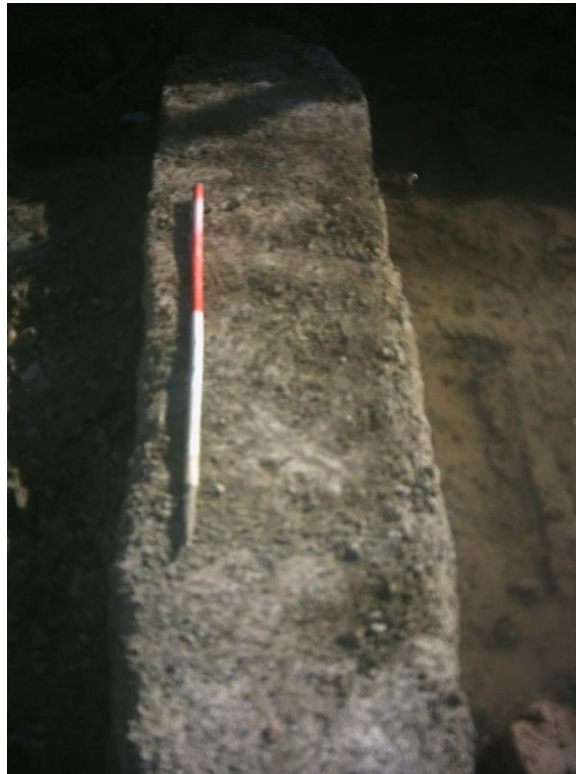
Plate 19: Concrete foundation (047). Facing E.
