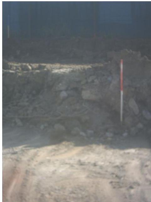
Plate 17: Concrete surface (046) and overlying demolition material (019). Facing E
