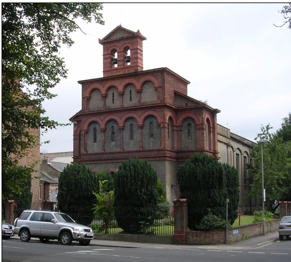
Plate 2: Photograph of the present W front of Christ Church, Brunswick Square, built in 1899-1900
