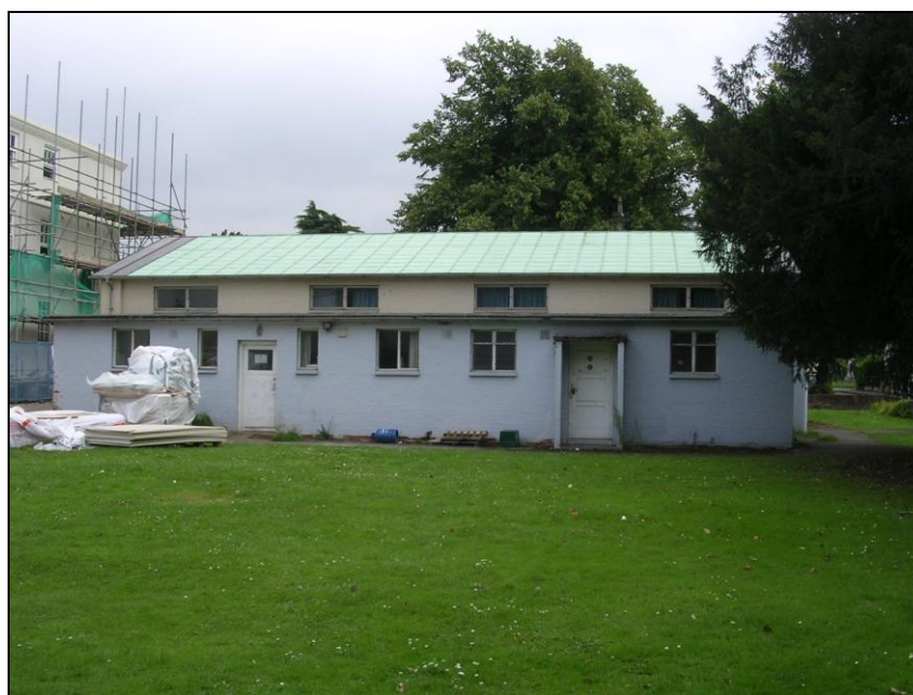
Plate 3: View looking E showing W front of Christ Church Hall, opened in July 1950
