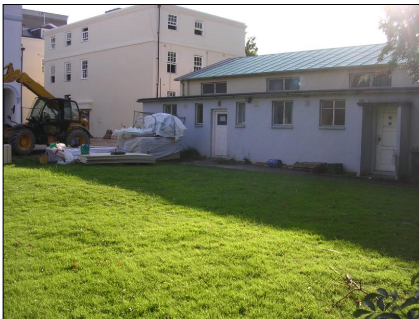
Plate 4: View looking NE showing shallow depressions aligned E-W, located on the grass lawn immediately W of Church Hall
