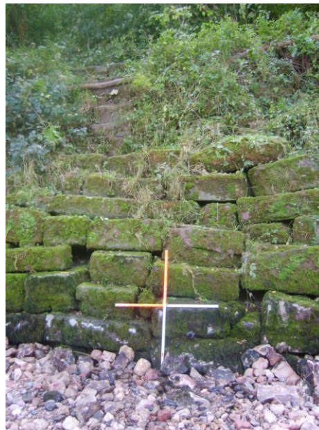
Plate 6: Revetted embankment on the E side of the river
