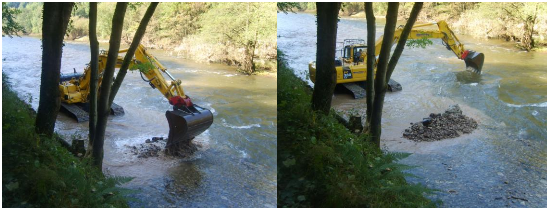
Plates 1 & 2: Removal of material from the river channel for access platform
