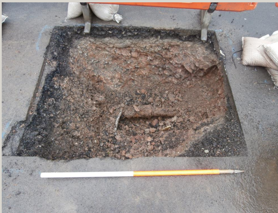
Plate 14: View NE of Trench of 13
