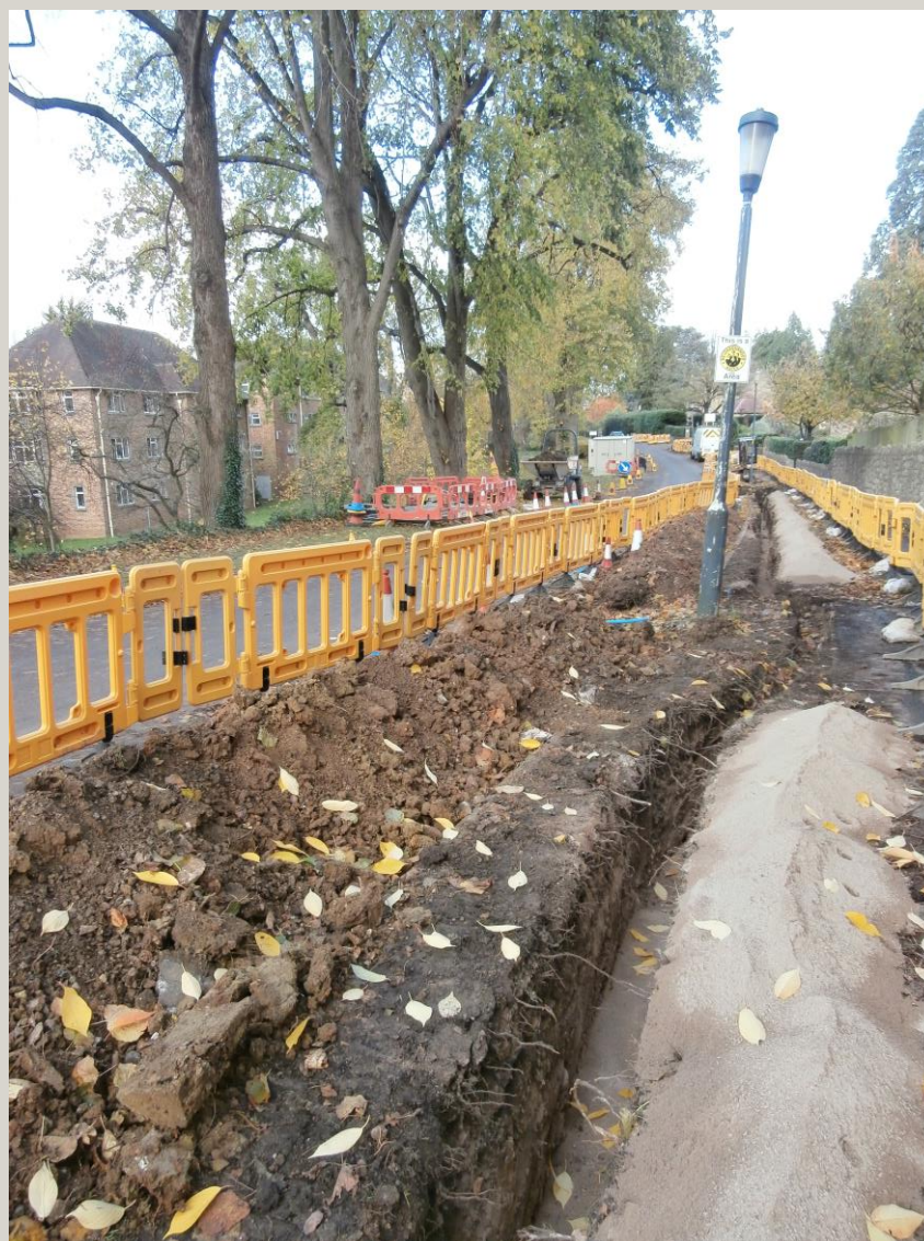
Plate 3: View to the NE, Trench 4 on Stoke Park Road
