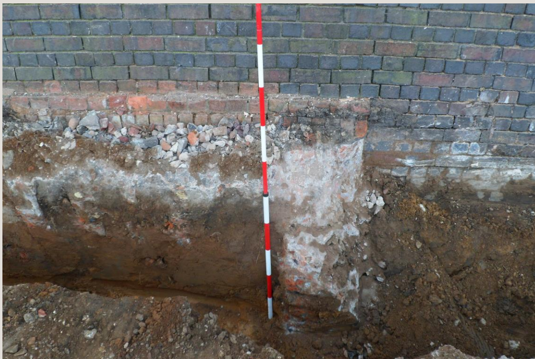
Plate 3: View SE showing termination of (102) as defined by remains of brick pier/wall (105) with deposit (111) shown right of picture
