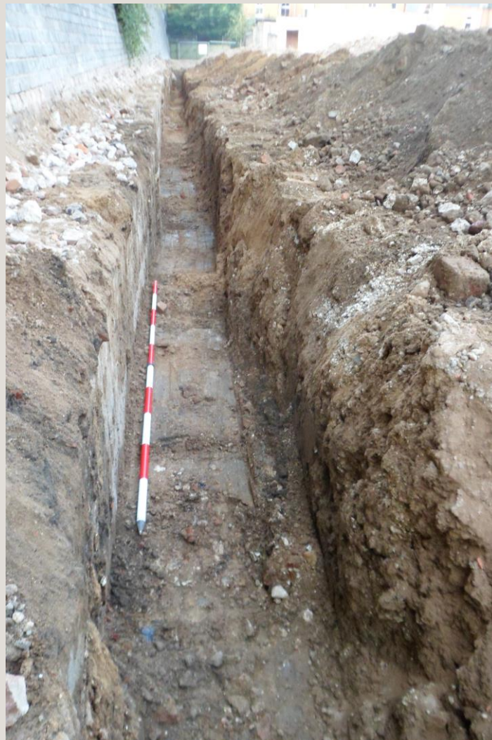
Plate 7: View SW towards Market Street showing extent of trenching
