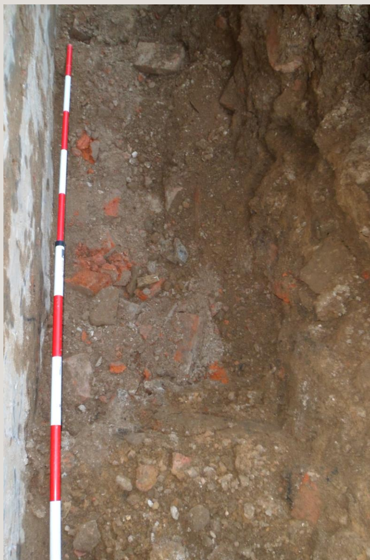
Plate 6: View of trench base showing demolition rubble (113) revealed in places along the trench
