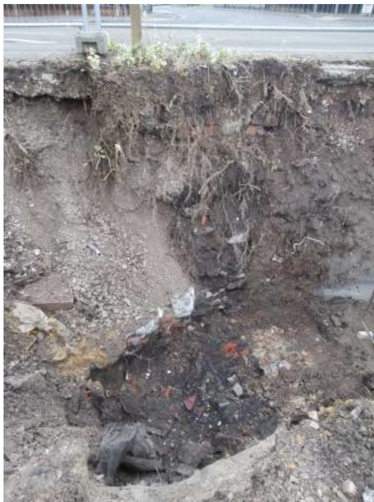
Plate 9: View to the NE of wall (1019)
