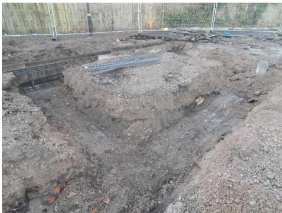
Plate 2: View to the SW depicting the modern made ground and levelling layers present across the site
