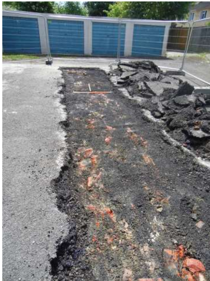
Plate 2: View S showing remains of brick carpark surface or hardstanding
