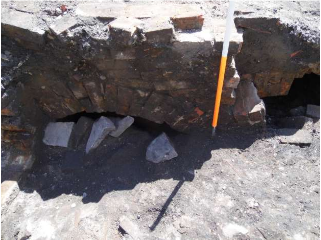
Plate 2: View S of barrel-vaulted roof of cellar (106)
