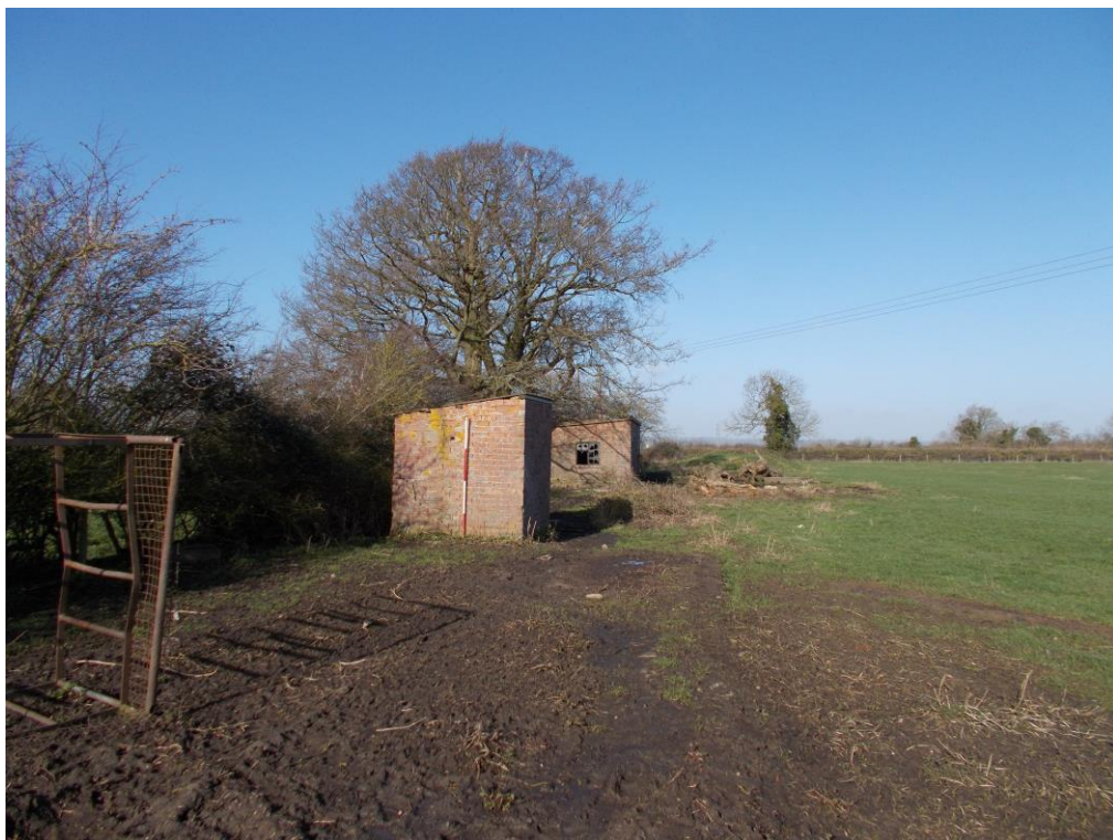
Plate 27: View W showing full extent of concrete plinth for hut to SE of Building G
