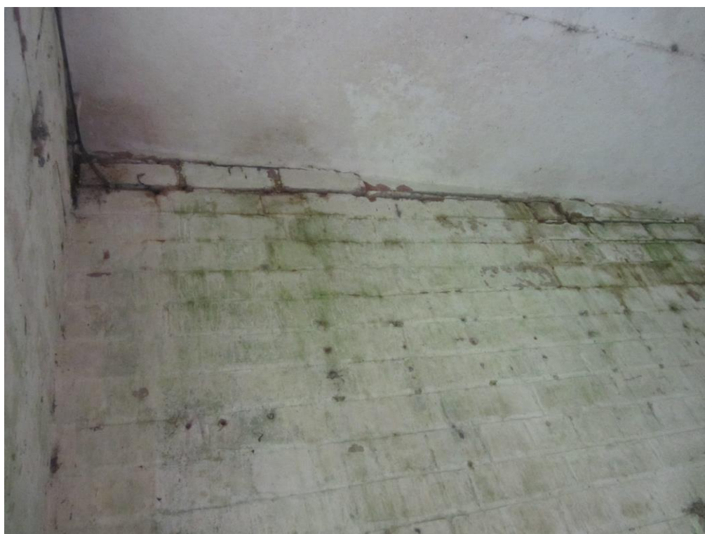
Plate 15: Detail showing indentations for shelving in SE compartment of Building B
