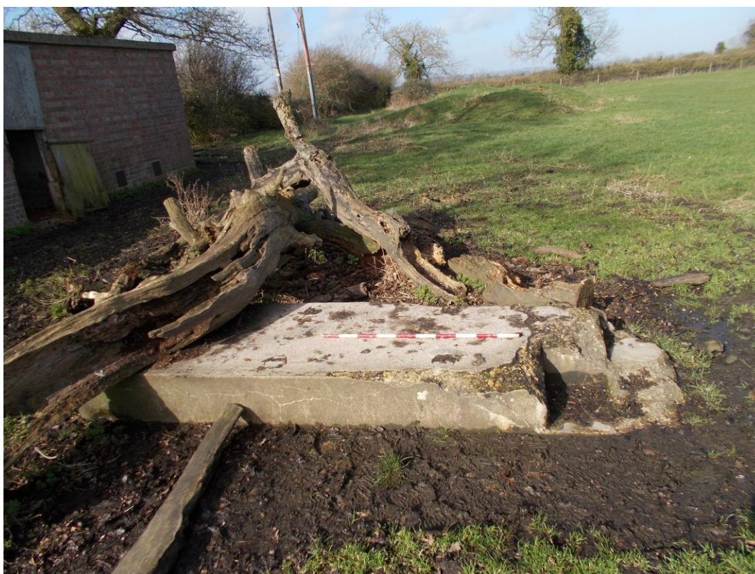
Plate 17: View looking NW showing concrete machine base, probably for a generator, standing upon a rectangular foundation plinth for a prefabricated structure (Building D)
