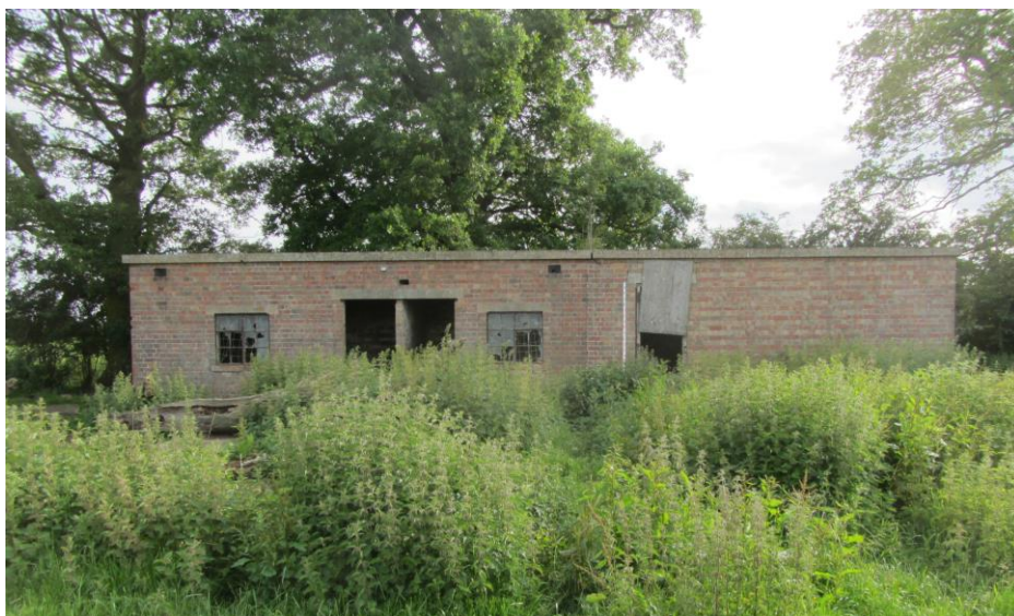
Plate 1: View looking SW showing principal NE-facing elevation of Buildings A & B
