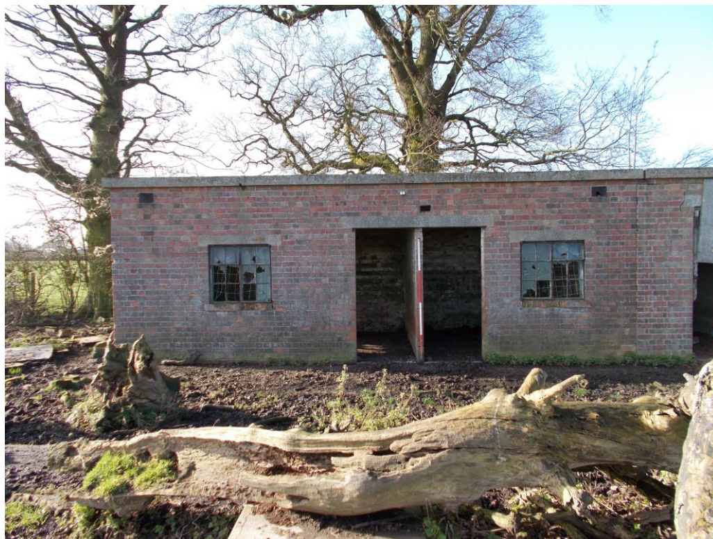
Plate 2: View looking SW showing detail of NE-facing elevation of Building A
