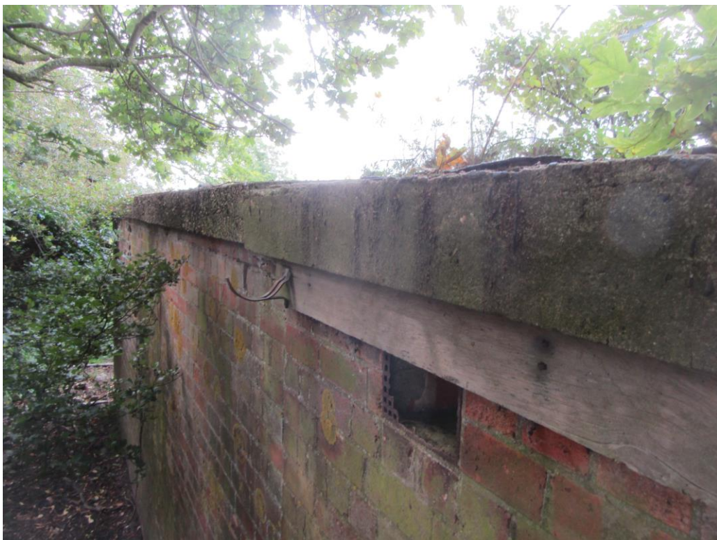
Plate 8: View looking NNW showing rear elevation of Building B
