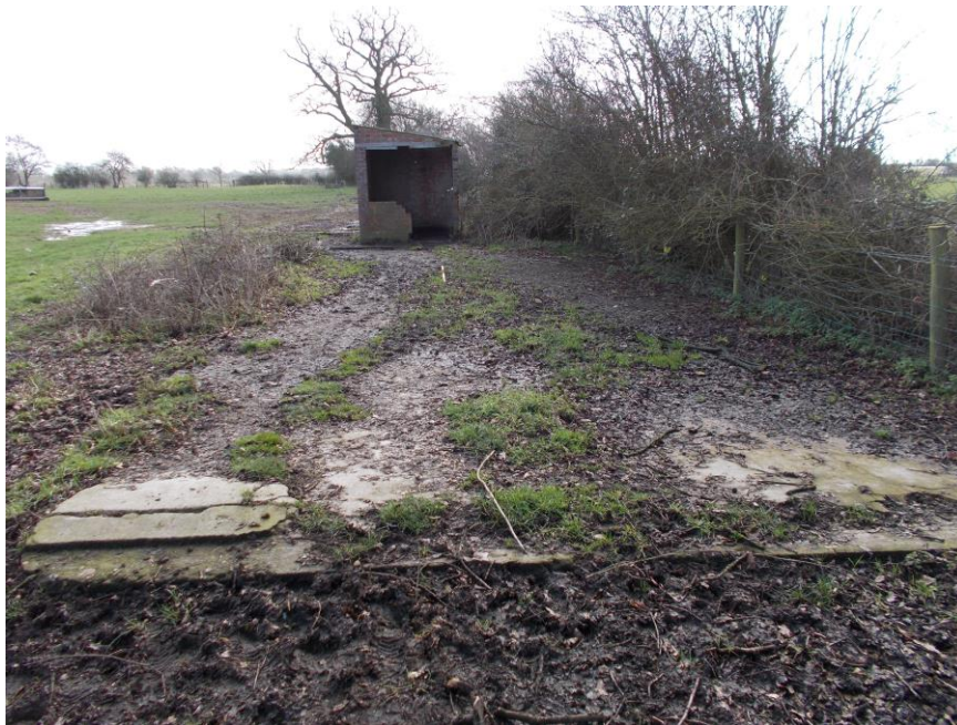
Plate 23: View SE showing rectangular concrete plinth for prefabricated hut (Building F), with Building G in background
