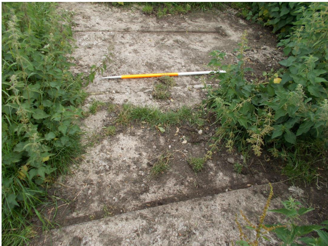
Plate 22: Detail showing divisions for cubicles within the toilet or washhouse block (Building E)
