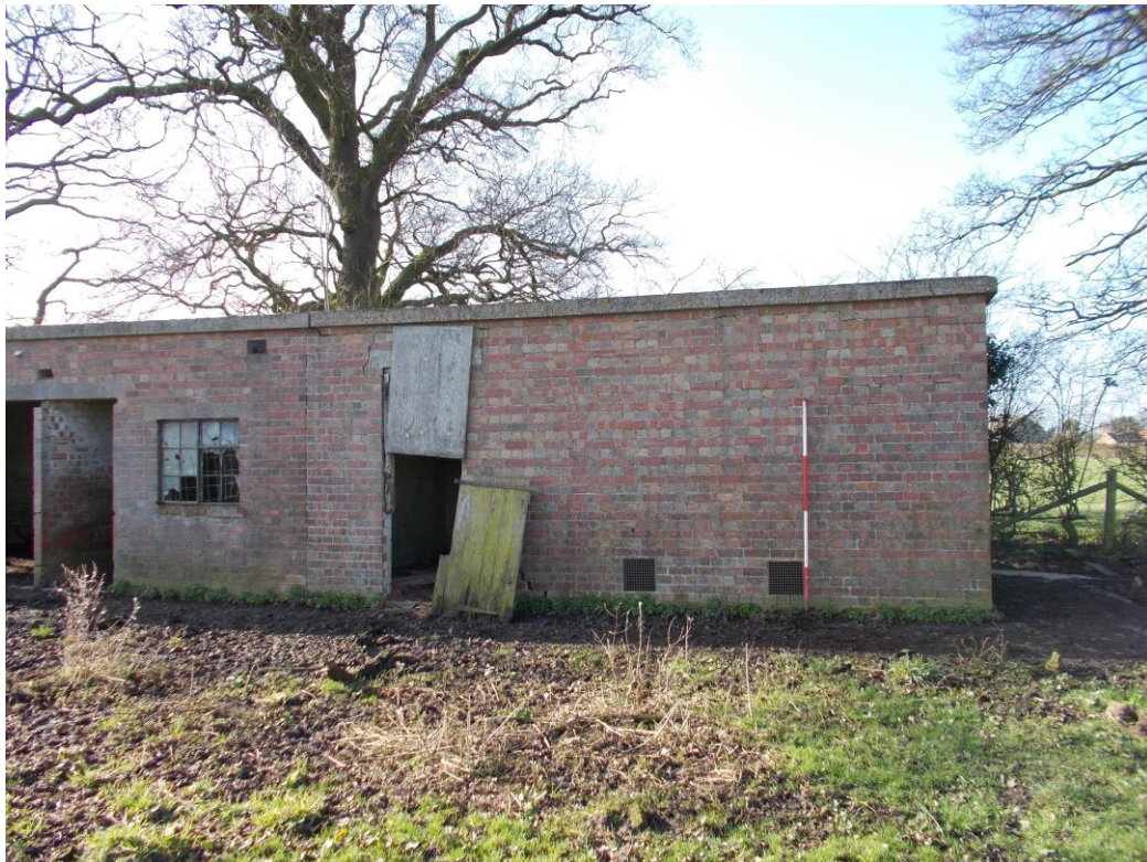
Plate 4: View looking S showing NE-facing elevation of Building B
