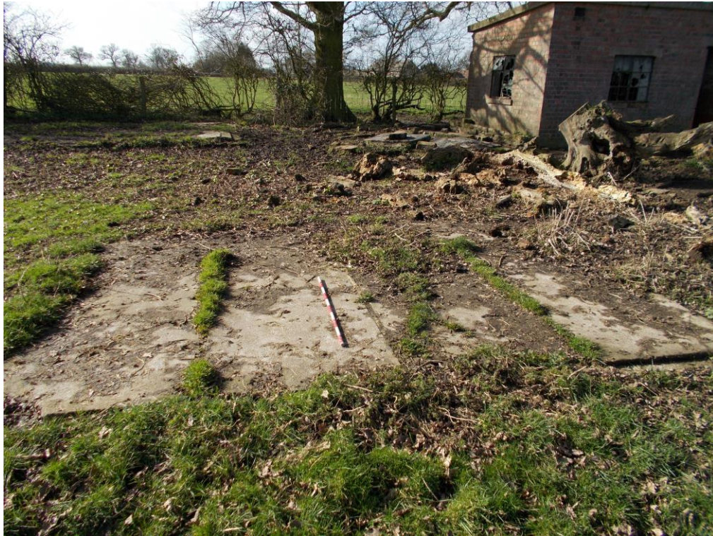
Plate 21: View SW showing concrete foundations of probable toilet or washhouse block (Building E)
