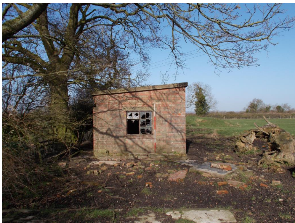
Plate 3: View looking NW showing SE-facing elevation of Building A
