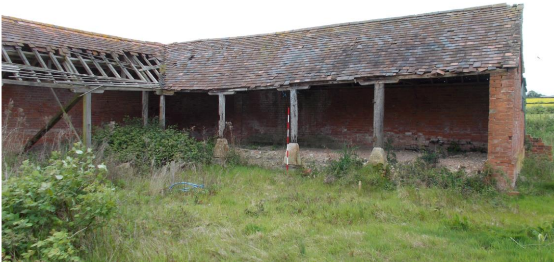
Plate 11: View looking southeast showing L-shaped range of animal shelters with partially denuded tiled roof to south of Building A
