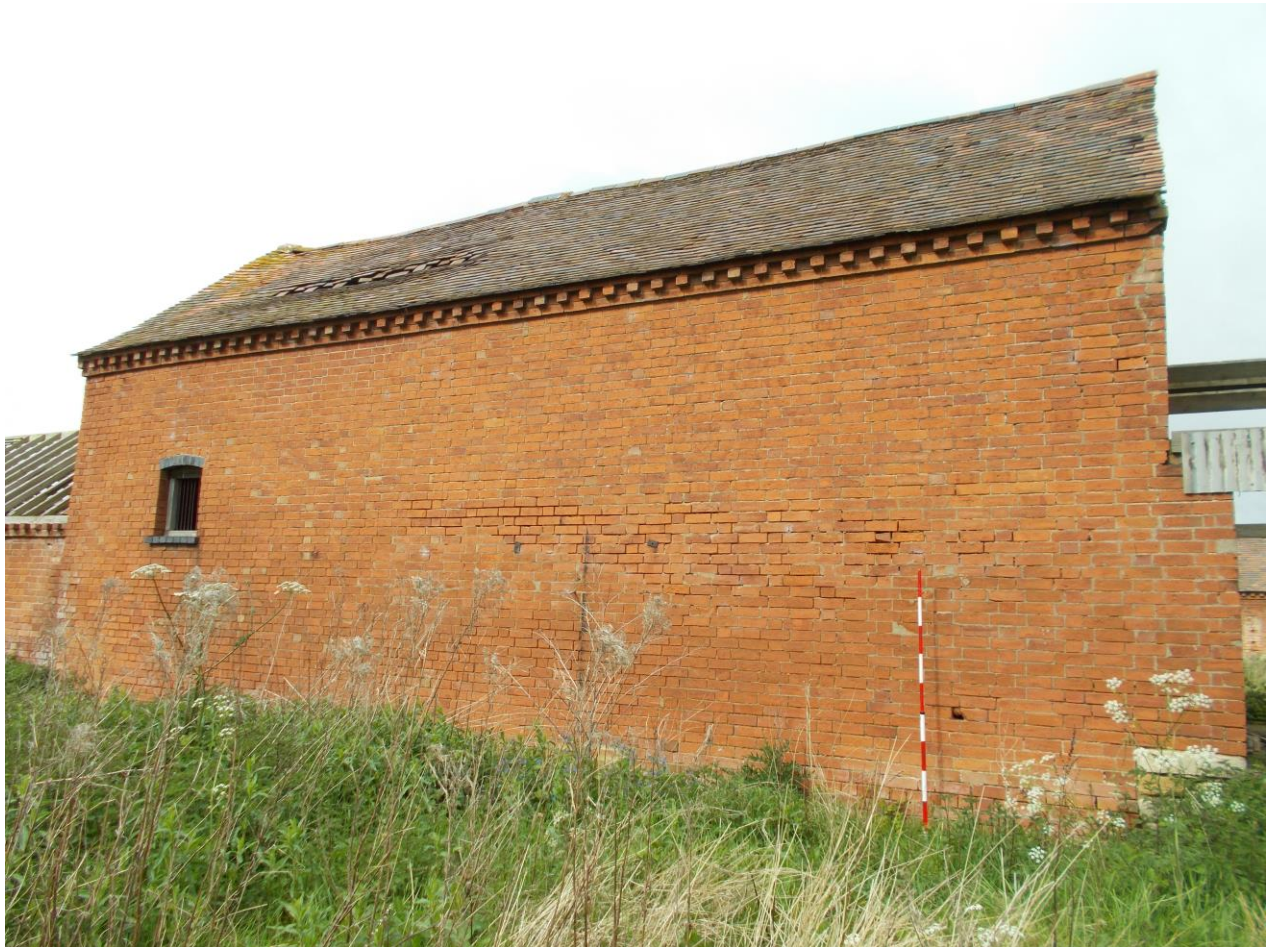
Plate 6: View looking west showing rear (east-facing) elevation of Building A with dentilled cornice at eaves level
