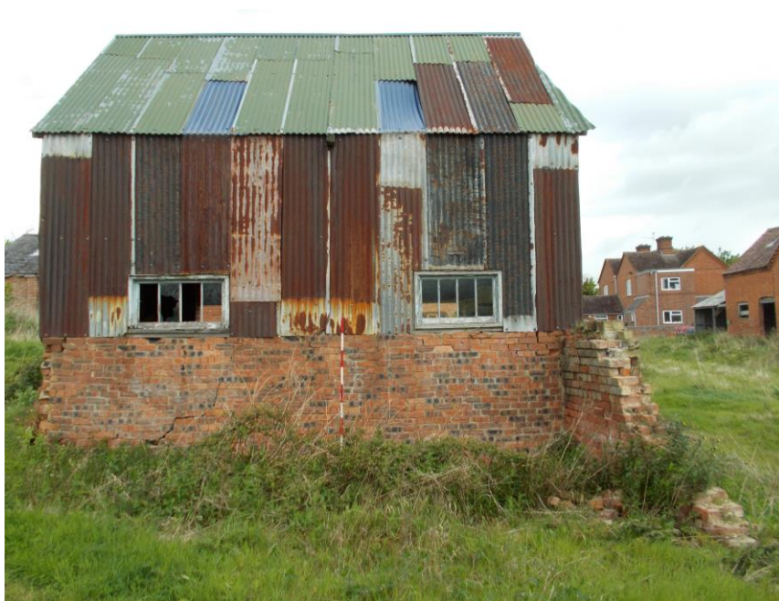
Plate 17: View looking north showing south-facing elevation of Building B showing wall stub representing remains of barn wall
