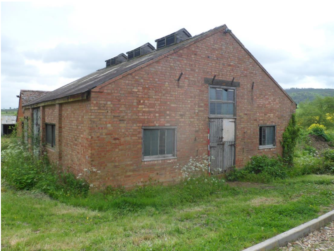
Plate 23: View looking east southeast showing west-facing gable elevation of Building D
