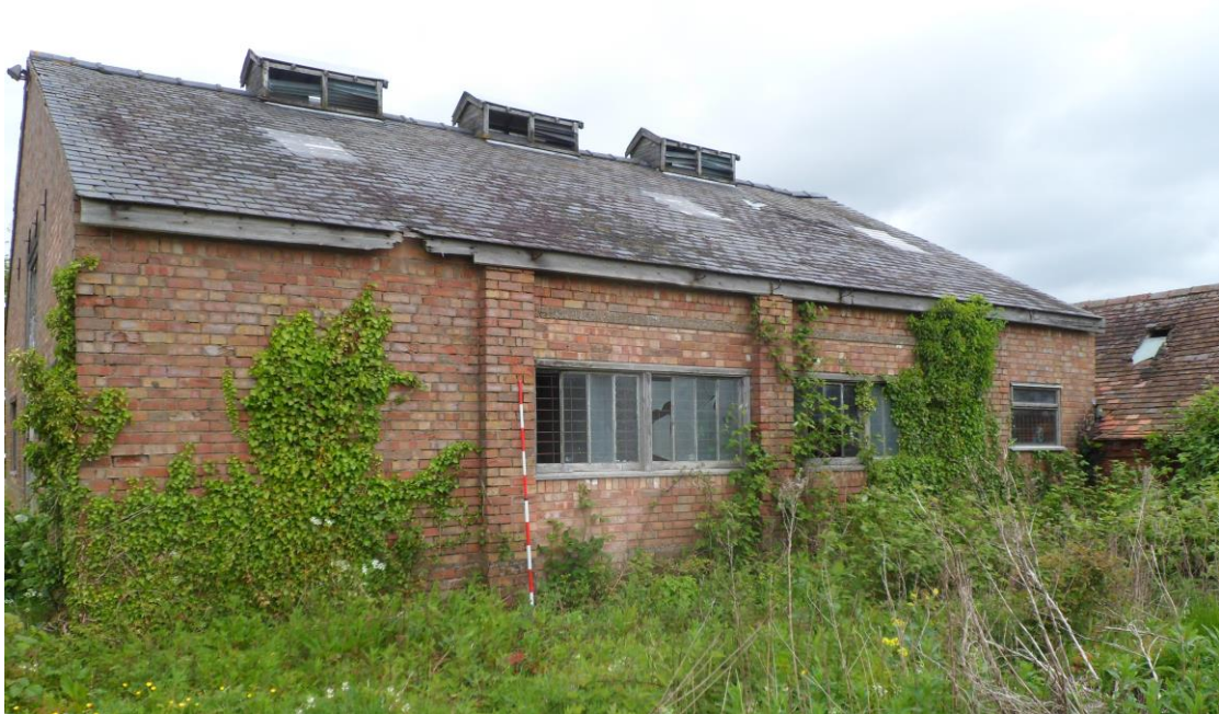
Plate 24: View looking north showing south-facing elevation of Building D
