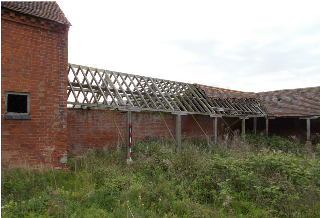
Plate 2: View looking southeast showing L-shaped open fronted range of livestock shelters to south of two storey main block (Building A)
