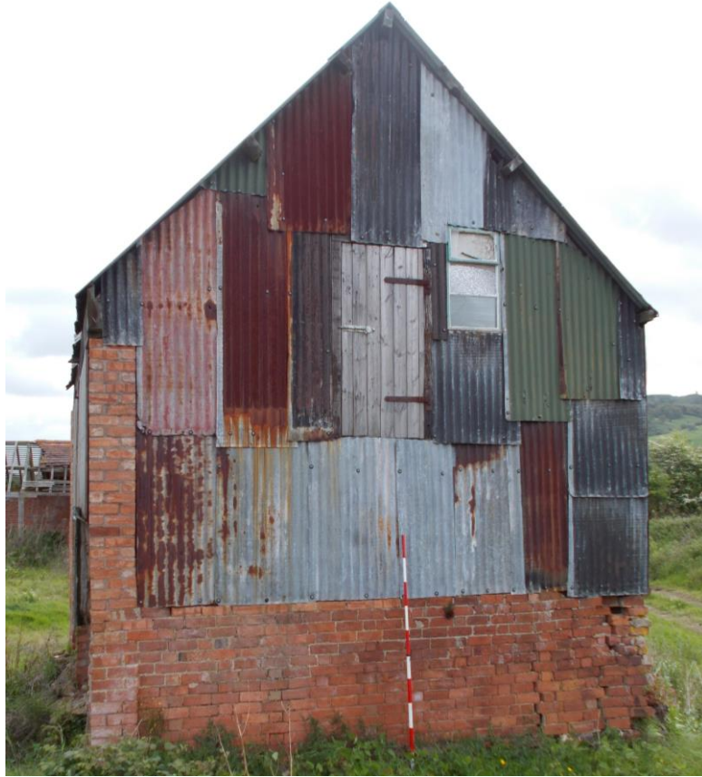
Plate 16: View looking east showing west-facing elevation of Building B with corrugated metal cladding upon a brick wall
