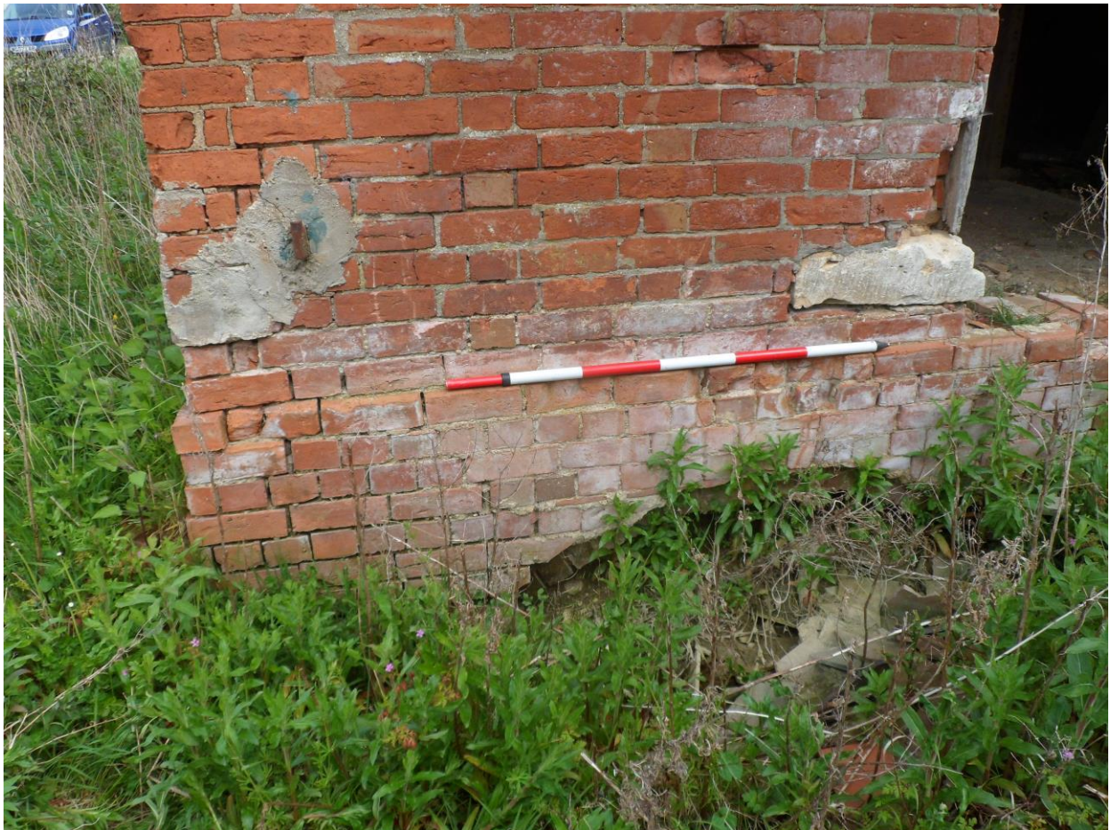
Plate 4: Detail showing arched culvert beneath doorway in south gable end of Building A
