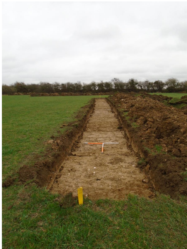
Plate 8: View NE along Trench 6
