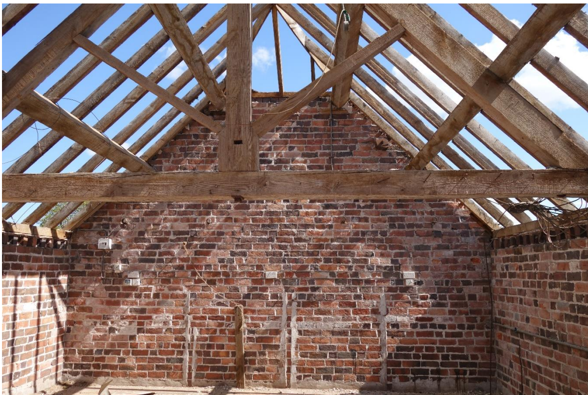
Plate 10: Internal view looking NE showing interior of granary with kingpost roof structure
