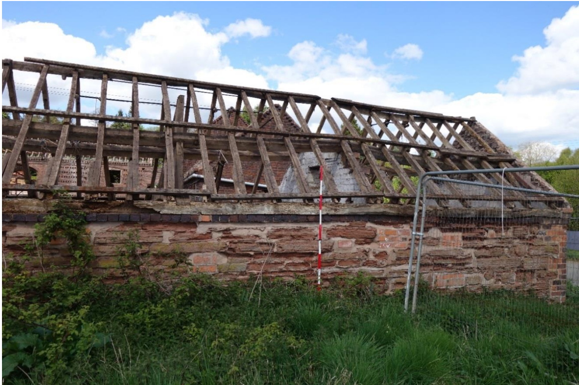
Plate 23: View looking NW showing SE-facing elevation of Building C
