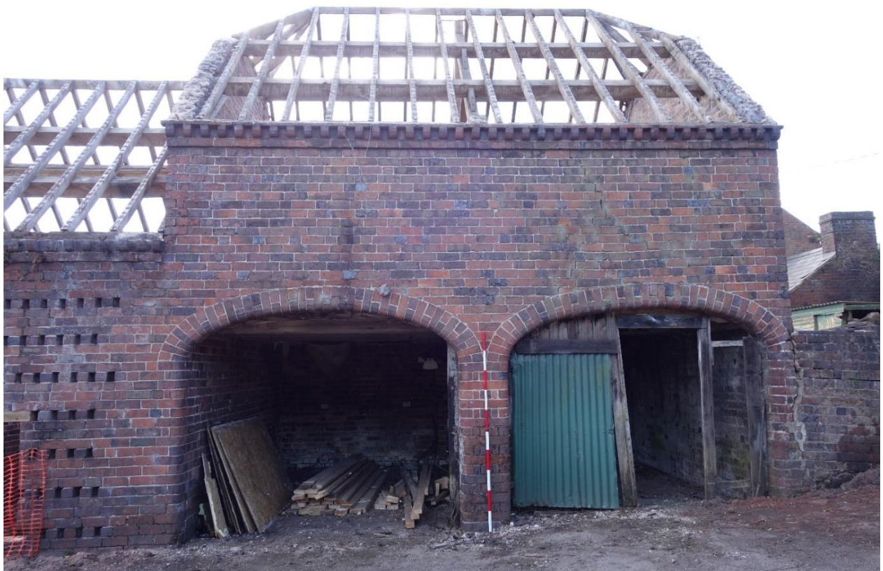
Plate 9: View looking SE showing NW-facing elevation of granary and cartshed, showing two depressed arched openings with brick voussoirs at ground level
