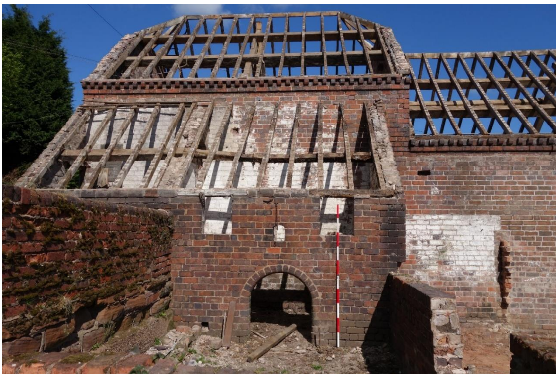
Plate 11: View looking NW showing SE -facing elevation of lean-to piggy structure with wall stub of demolished lean-to building visible to right of picture
