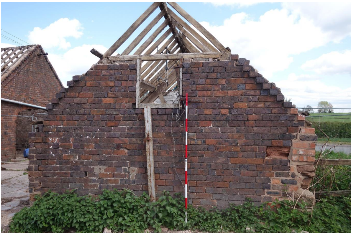
Plate 22: View looking NE showing SW gable end of Building C
