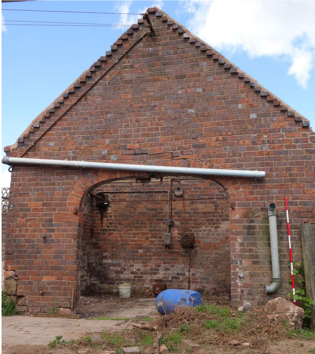
Plate 16: View looking NW showing SE gable end of Building B with a centrally placed, depressed arched opening with brick voussoirs and imposts and dentilled decoration along the roofline of the gable
