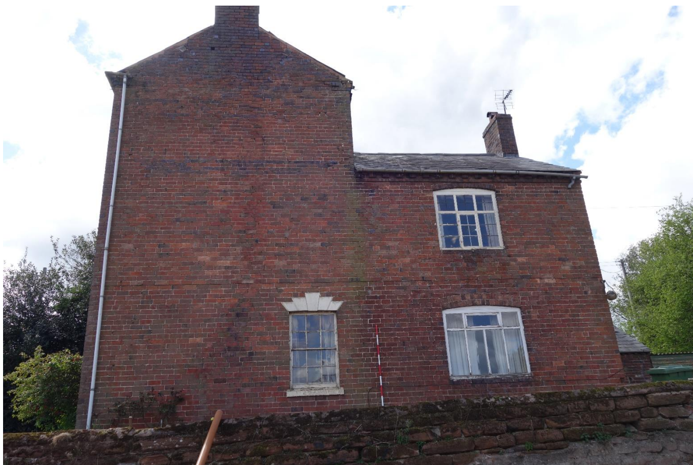
Plate 30: View looking SW showing the NE -facing elevation of the farmhouse with double-pile gabled block to rear
