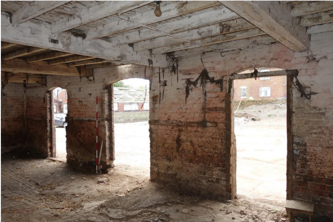
Plate 18: Internal view looking S showing interior of four-bay stable block with segmental-arched doorways
