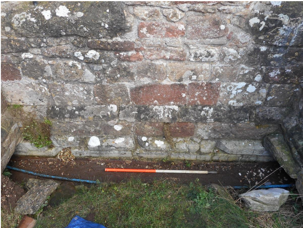
Plate 1: View N of South Cloister wall and slate drainage channel (203)
