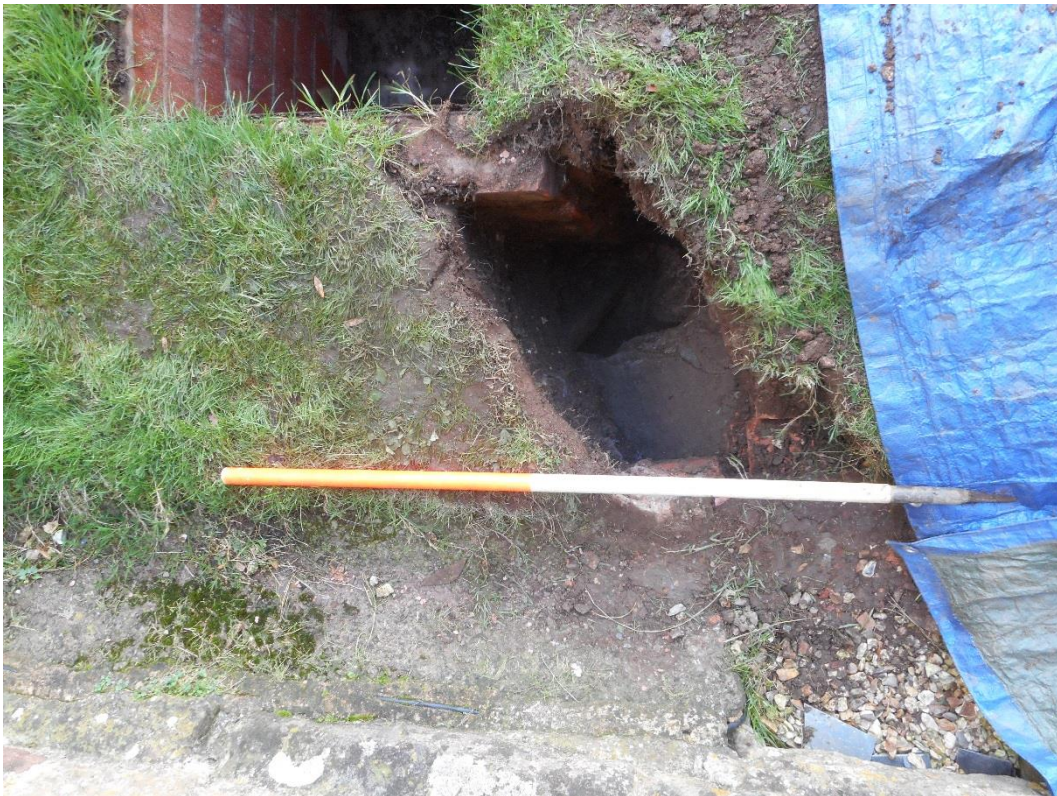
Plate 2: View S of Pit 2 during excavation showing exposed slate layer (203)
