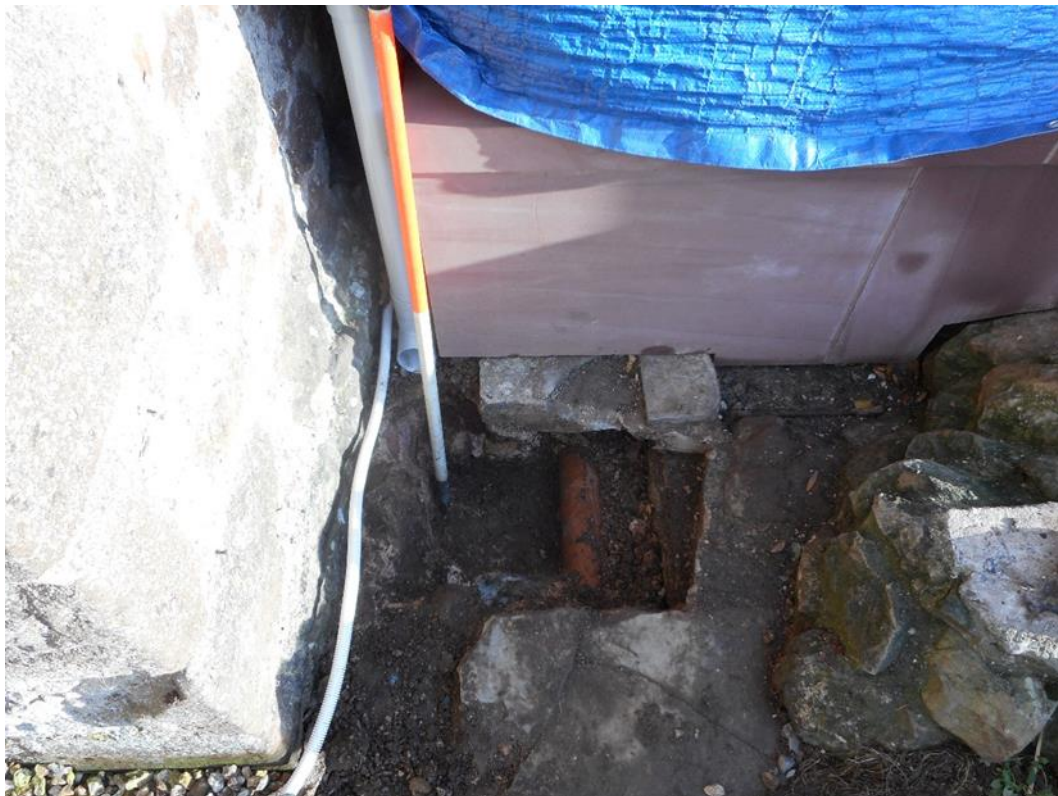
Plate 4: Post-excitation view E showing partially removed wall footing (302)
