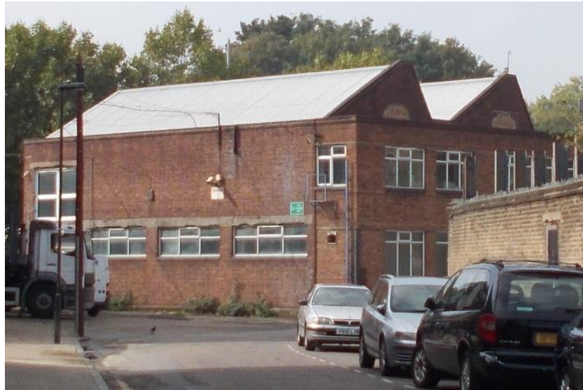
Plate 2: View looking WSW showing Dowding and Mills premises fronting onto White Post Lane
