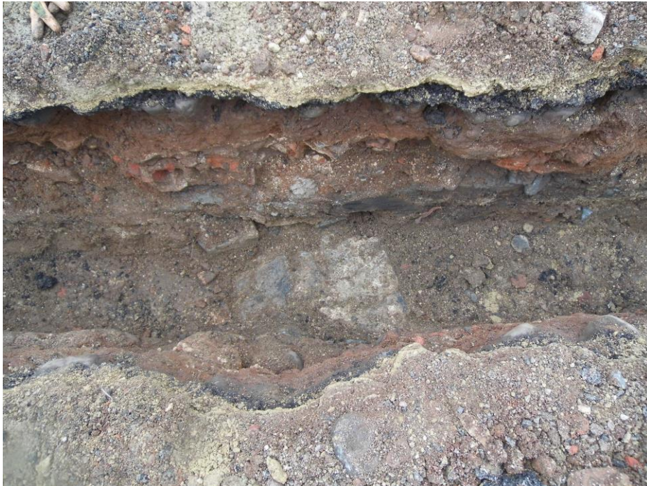
Plate 1: Wall (511) in the base of the trench; view N
