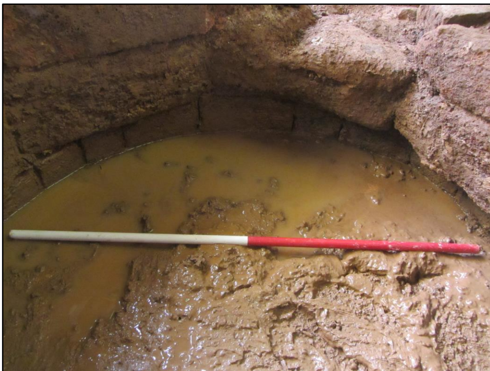
Plate 2: View SE showing Heavitree masonry upper courses (1002) with smaller-sized stones lining the shaft
