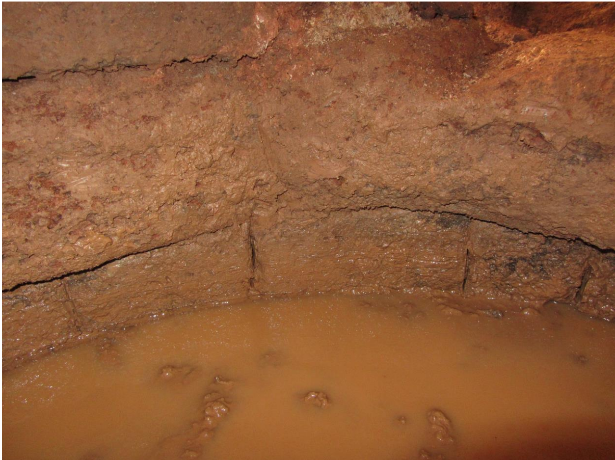
Plate 3 View of lower stone course (1002)
