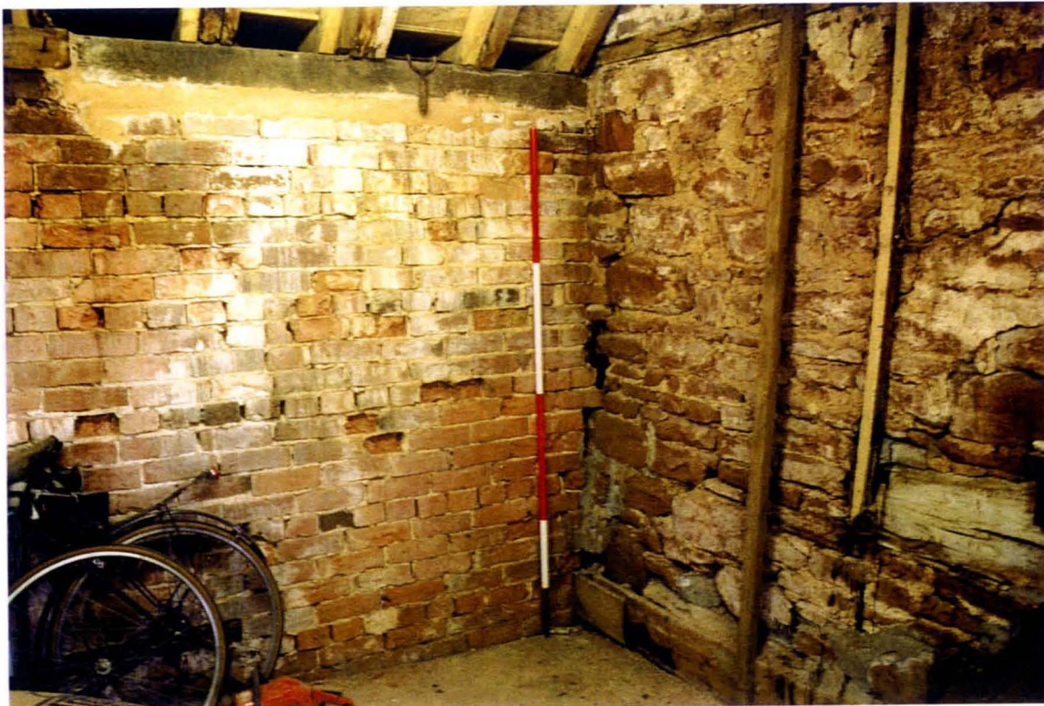
PLATE 5 FIRST FLOOR PARTY WALL ROUGHLY TIED INTO EAST ELEVATION
