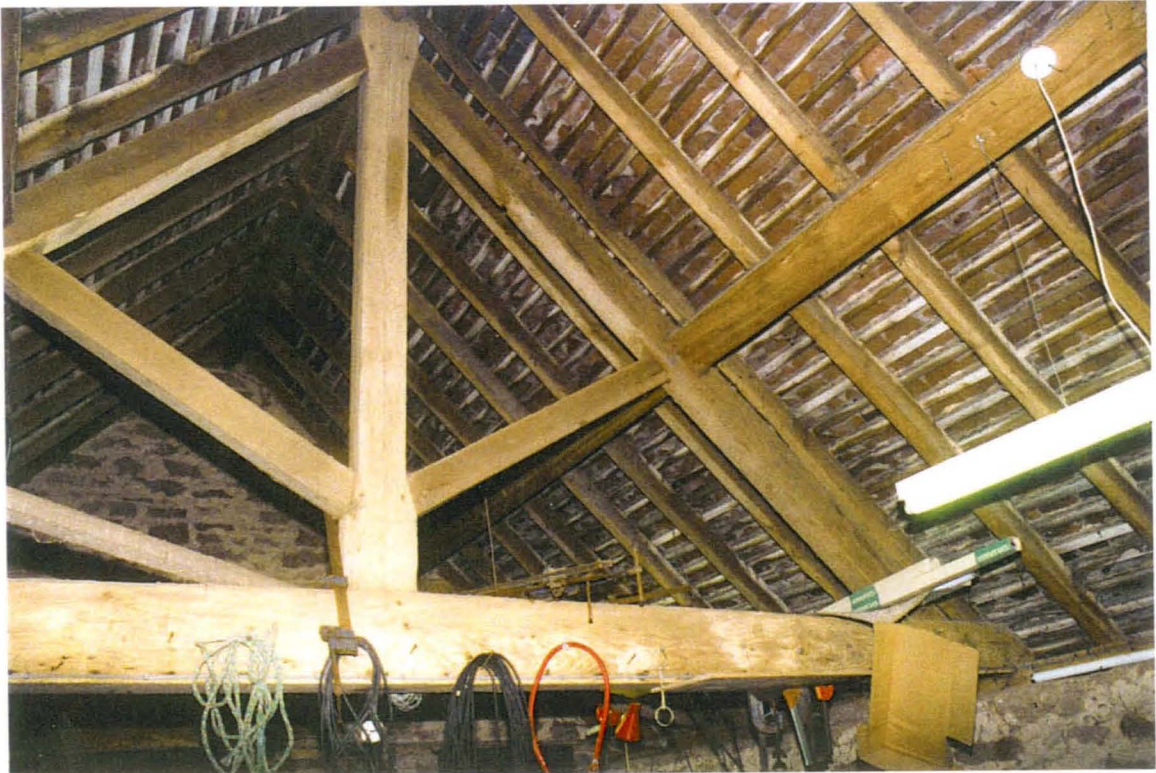
PLATE 7 A-FRAME - LOCATED IN THE NORTHERN SECTION OF THE BARN
