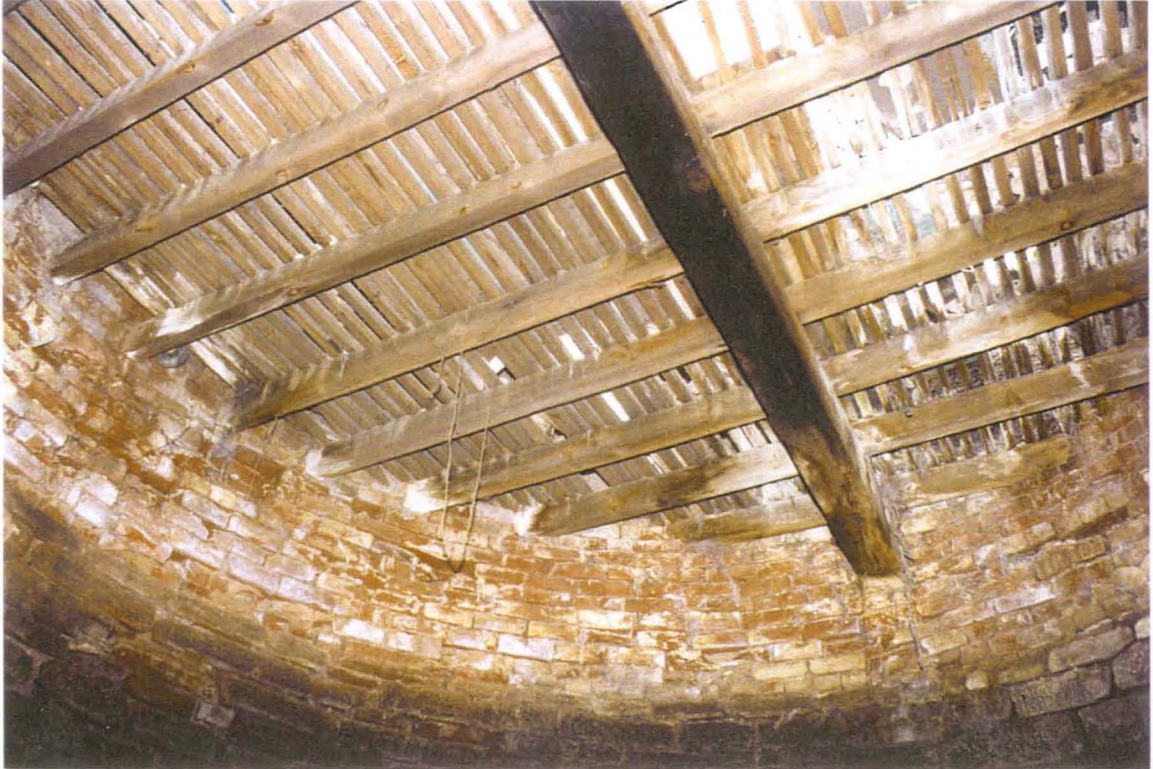
PLATE 9 DRYING UNIT IN THE NORTHERN KILN LOOKING NORTH-WEST
