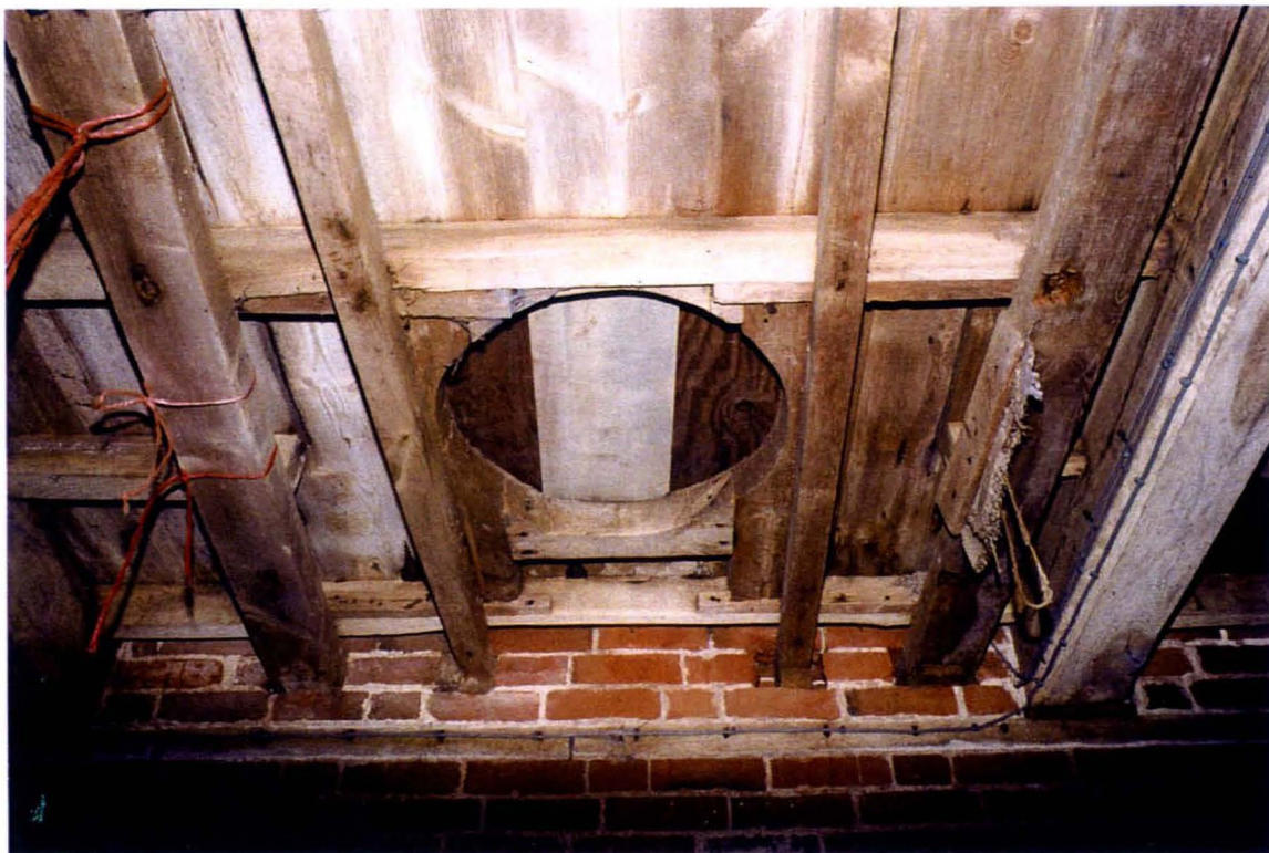
PLATE 6 POCKET HOPPER LOCATED CUT INTO 1st FLOOR OF THE BARN
