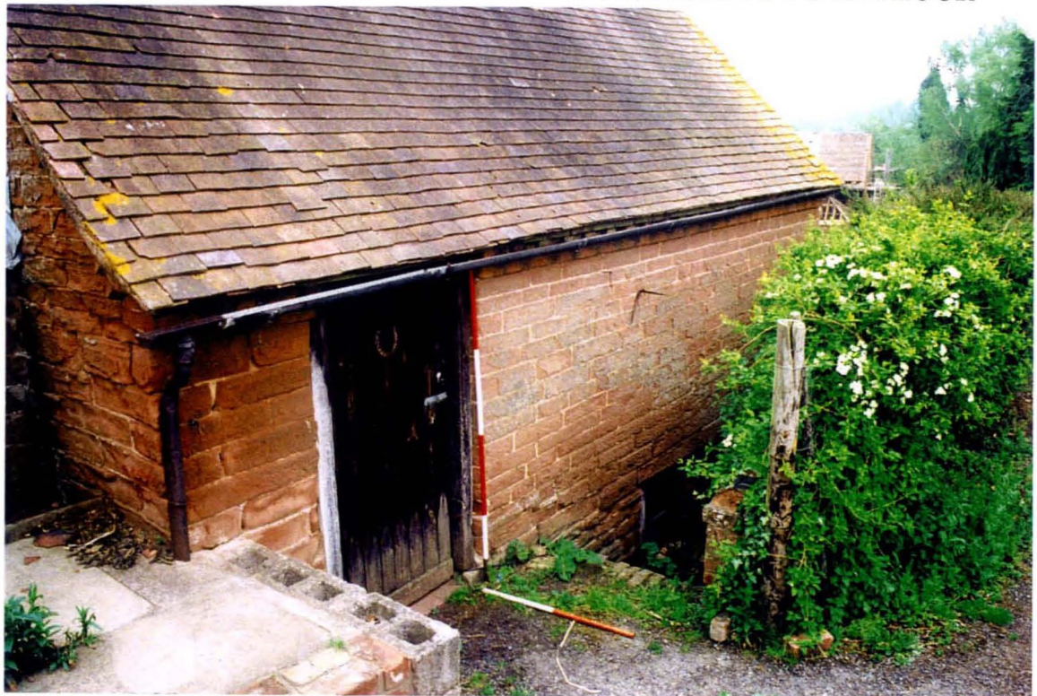
PLATE 4 S. ELEVATION OF BARN AND DOOR LEADING TO 1st FLOOR
