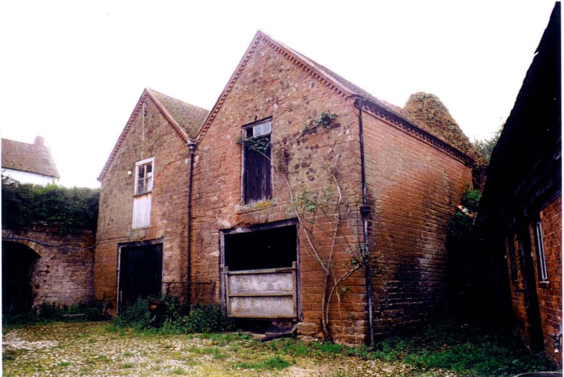
PLATE 1 EASTERN ELEVATION OF THE BARN LOOKING NORTH-WEST
