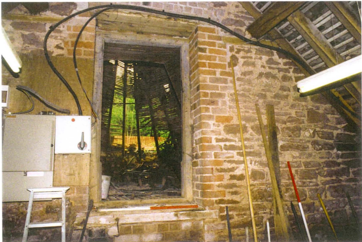
PLATE 8 DOOR OPENING TO UPPER SECTION OF THE SOUTHERN KILN
