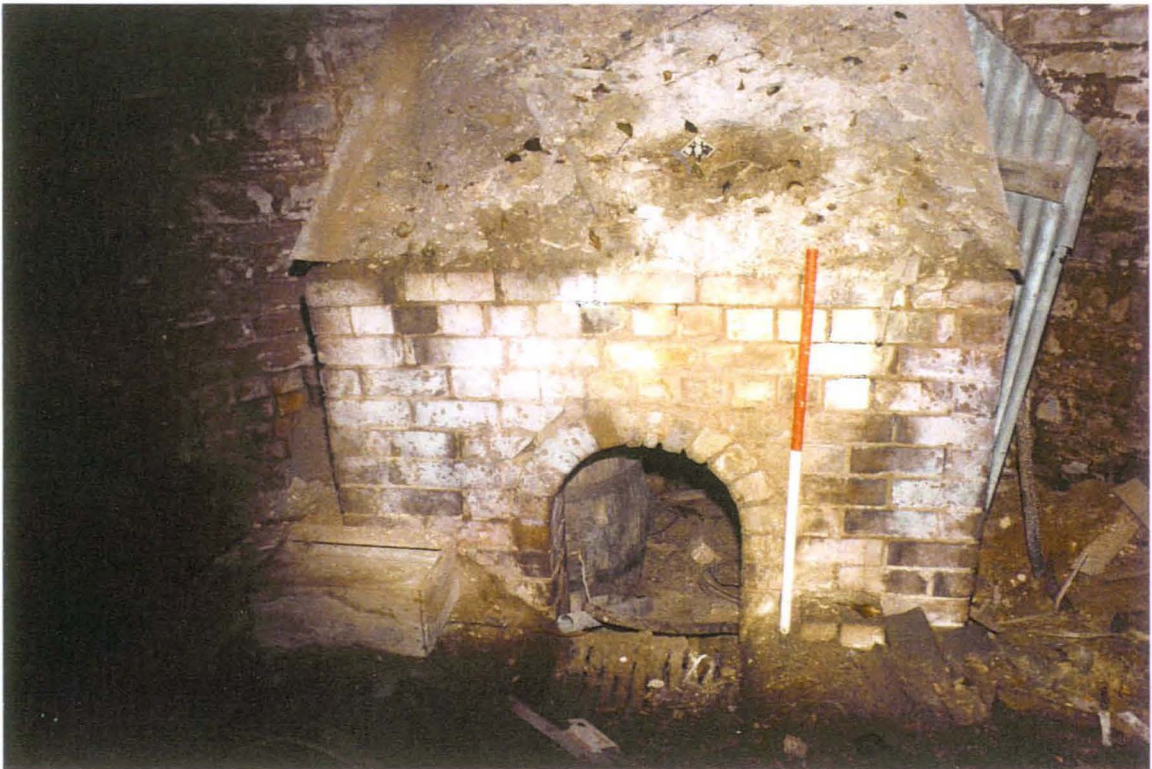
PLATE 10 OVEN IN NORTHERN KILN
