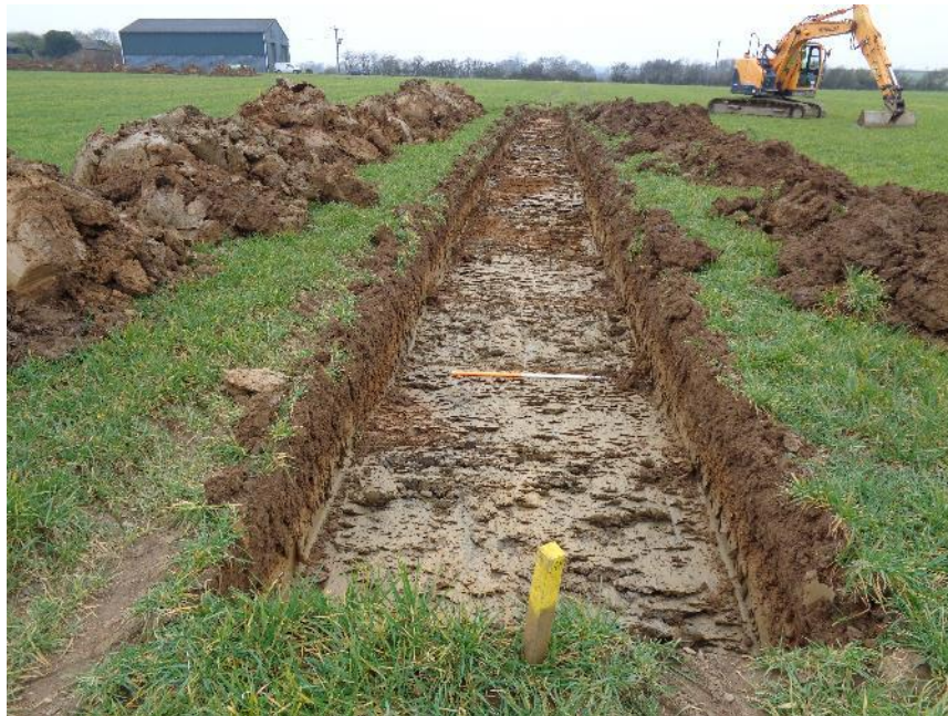
Plate 31: View WNW of trench 014
