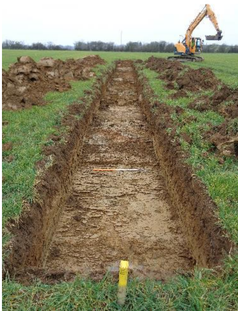
Plate 22: View WNW of trench 010
