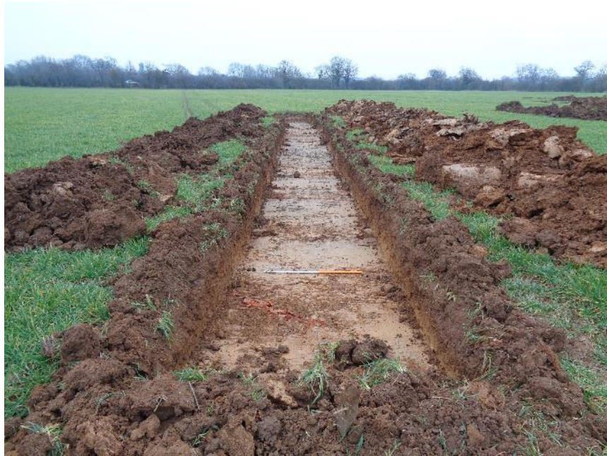
Plate 25: View SE of trench 011
