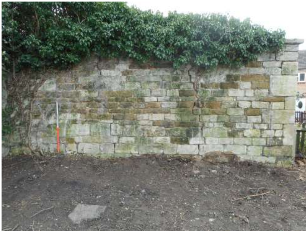
Plate 7: N-facing elevation of wall (501)
