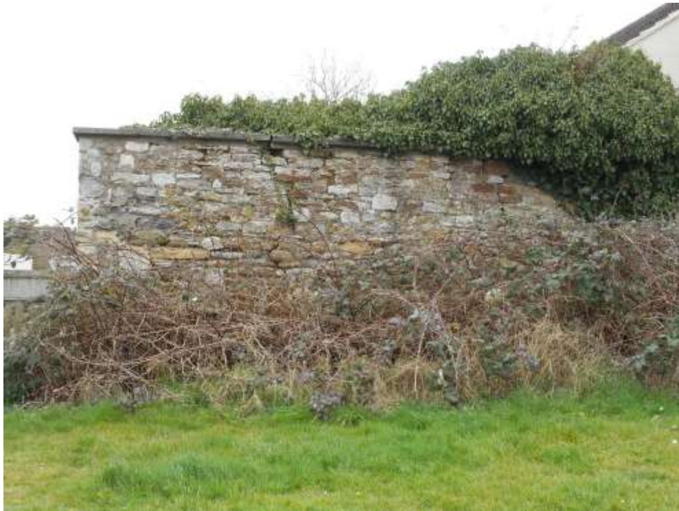
Plate 8: S-facing elevation of wall (501)
