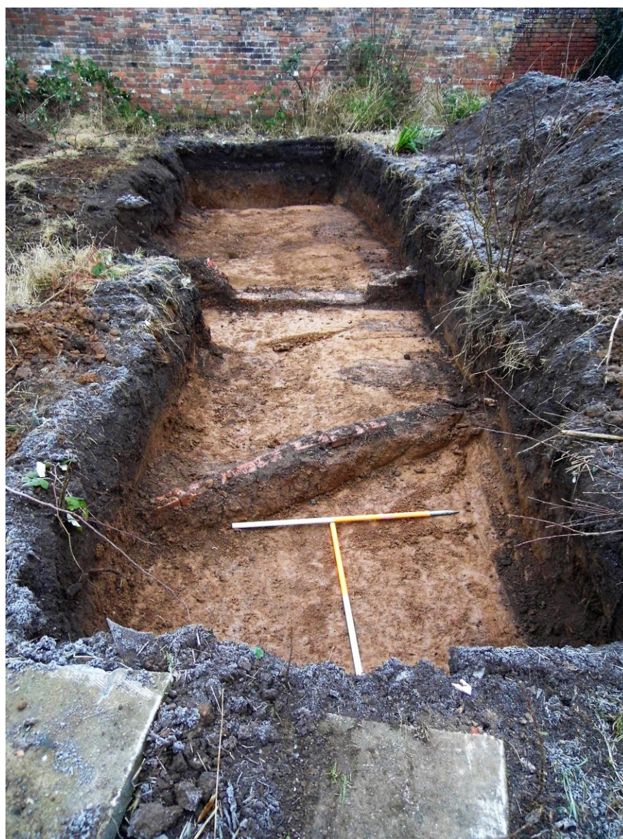
Plate 1: View NW showing structure (105) and electricity cable duct (112) (foreground)
