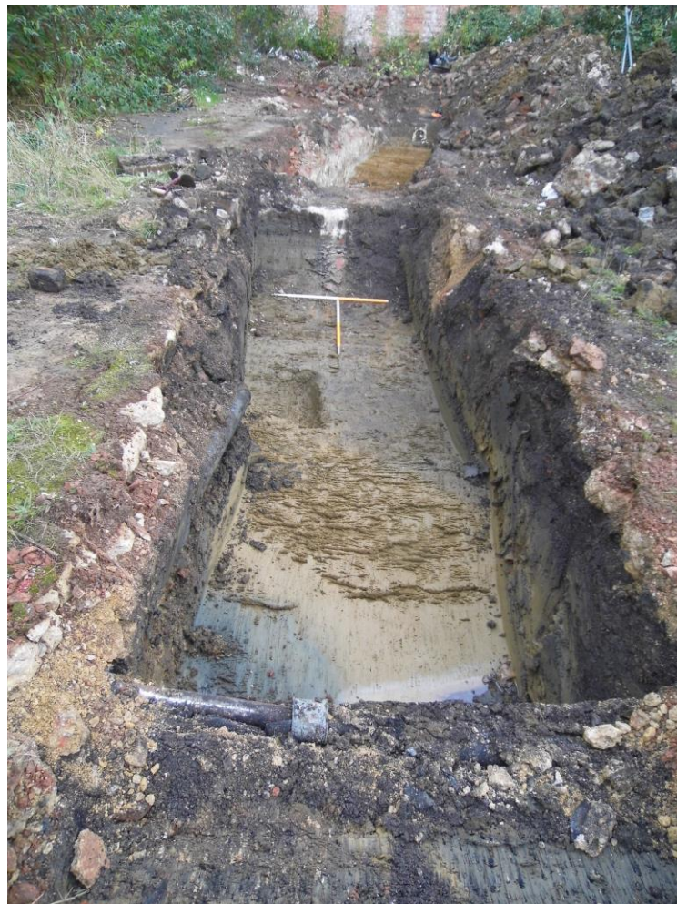
Plate 3: View NW of Trench 4 showing hand-dug sondage into fill (406) and footings (407), (410), with diesel contamination shown in corner of trench
