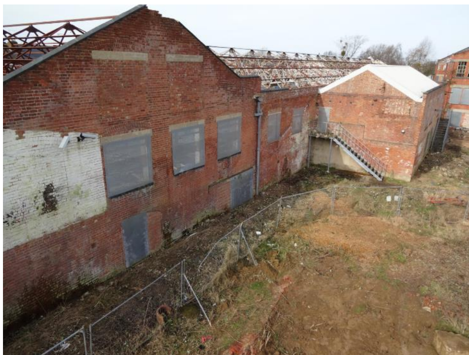
Plate 42: View NW of E elevation of Building 6 adjoining Building 5
