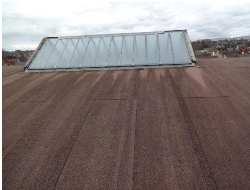
Plate 33: Detail of external roof structure of Building 3 showing lantern
