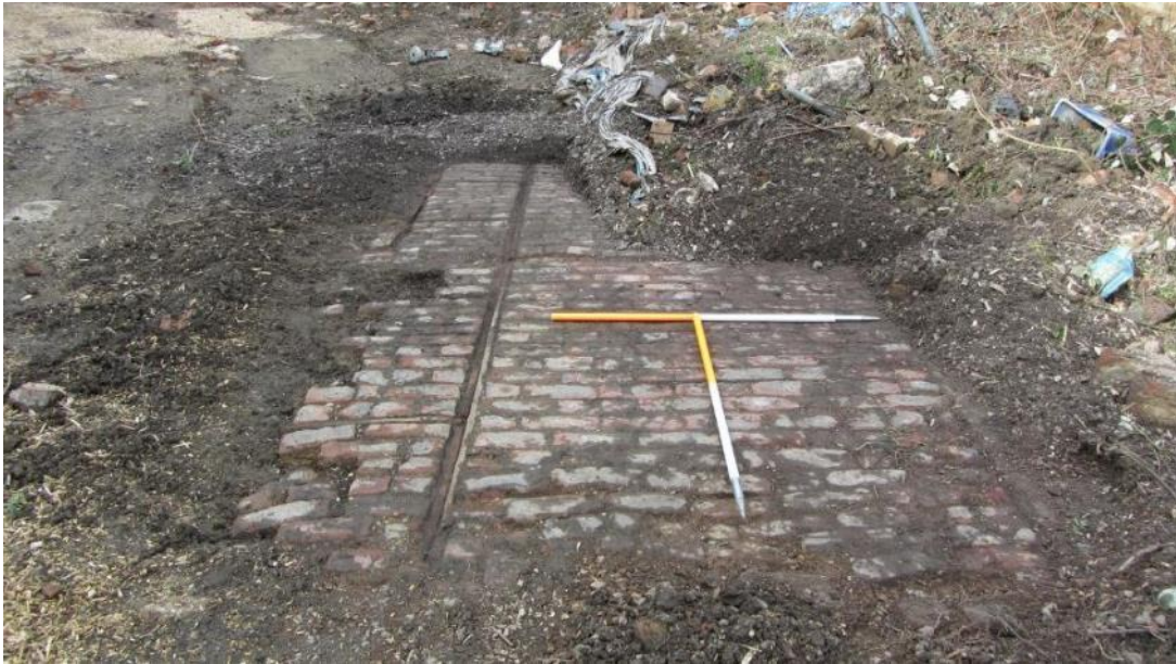
Plate 37: View NW showing extant remains of 'tramway' showing wooden rails and associated brick yardage
