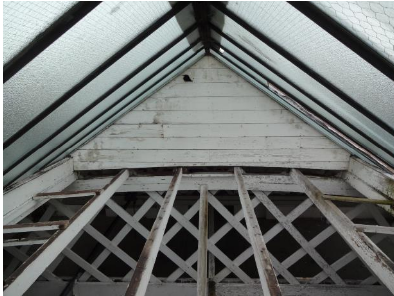
Plate 32: Internal detail of central lantern
