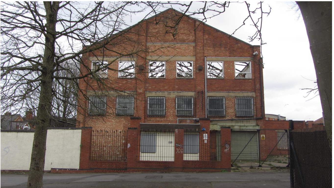
Plate 10: View SE of NW gable Building 1
