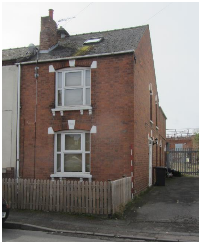
Plate 6: View SW showing Works access off No 116 Melbourne Street West
