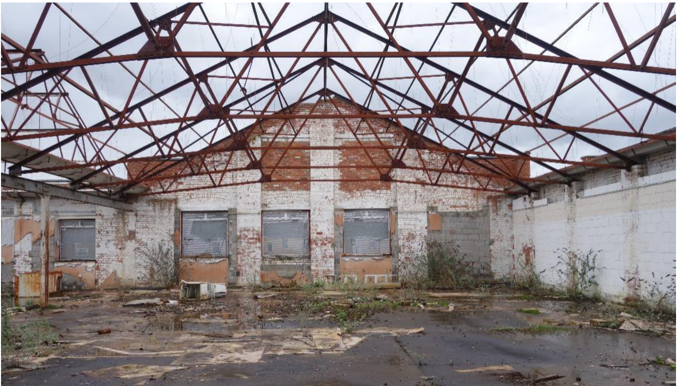
Plate 48: Interior of Building 6. View E showing roof structure and internal gable.
