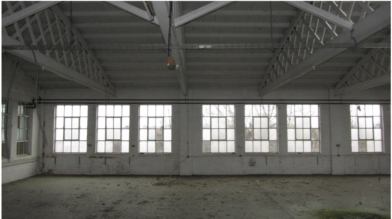
Plate 31: View E showing internal fenestration at upper-storey level
