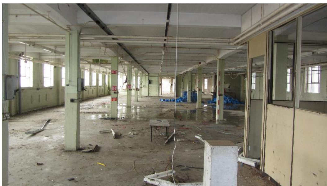
Plate 18: View showing interior of Building 2
