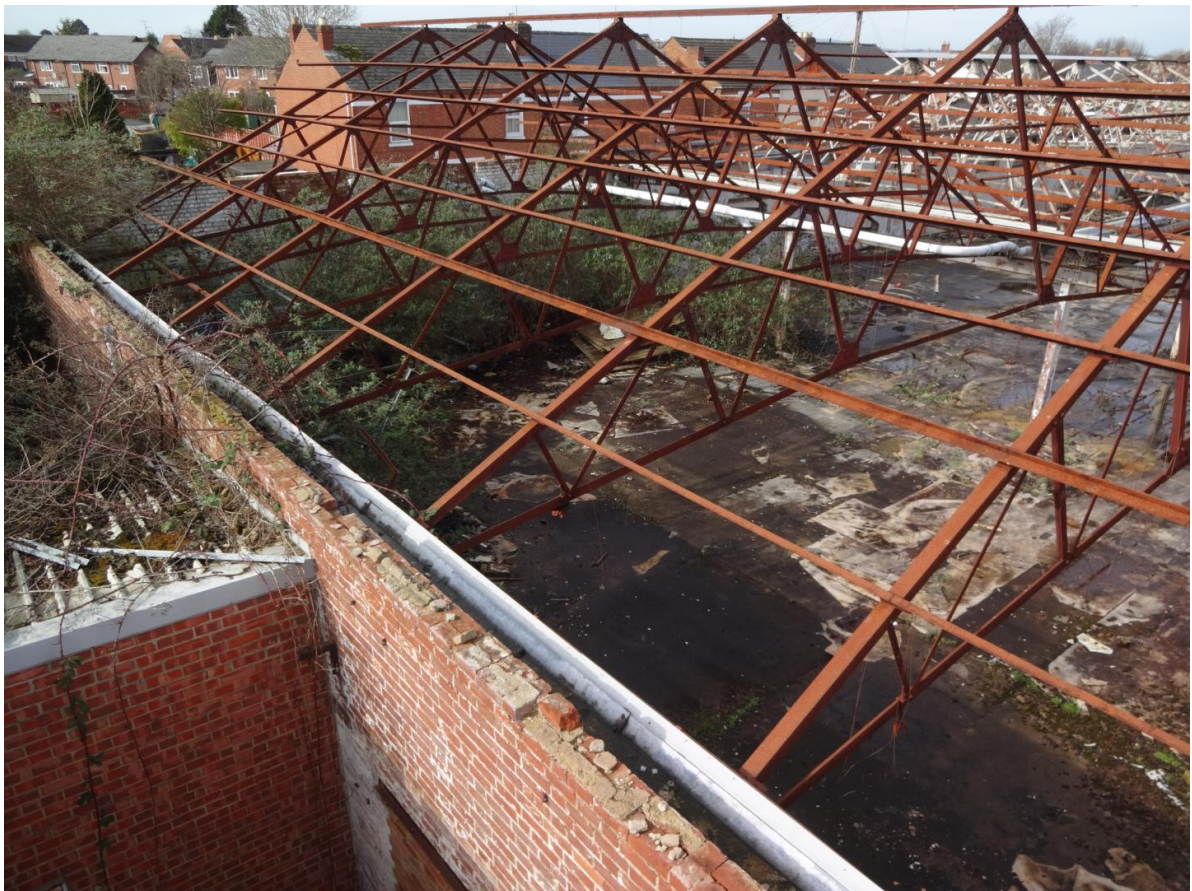
Plate 44: View W of Building 6 showing roof structure
