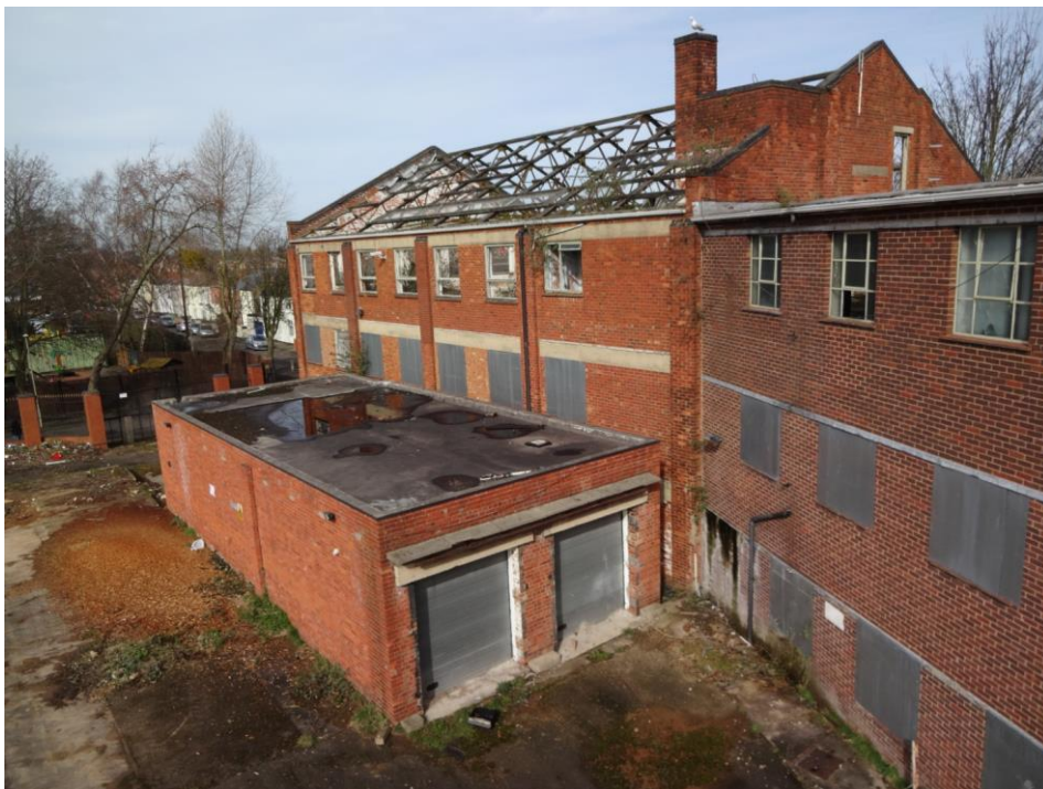
Plate 3: View N showing Buildings 1, 1a & 2
