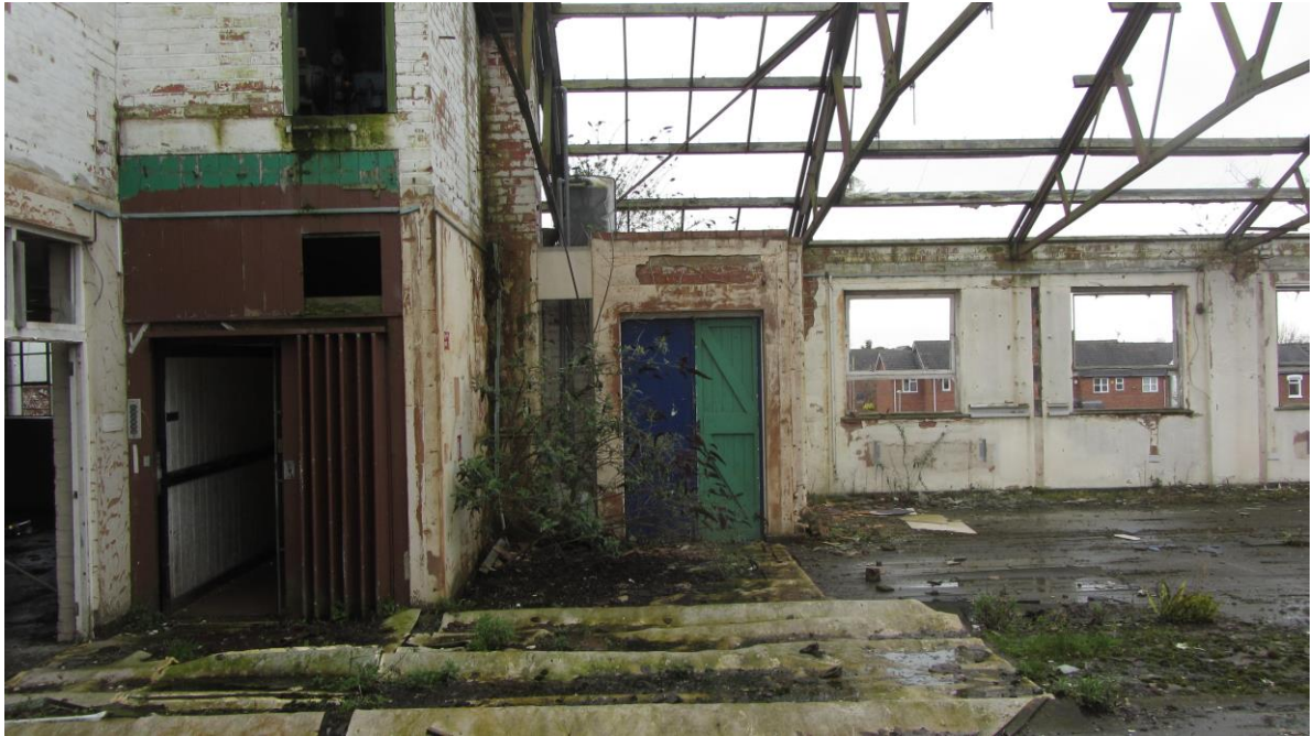
Plate 16: View NW showing goods elevator shaft and adjoining stairwell at upper storey level Building 1
