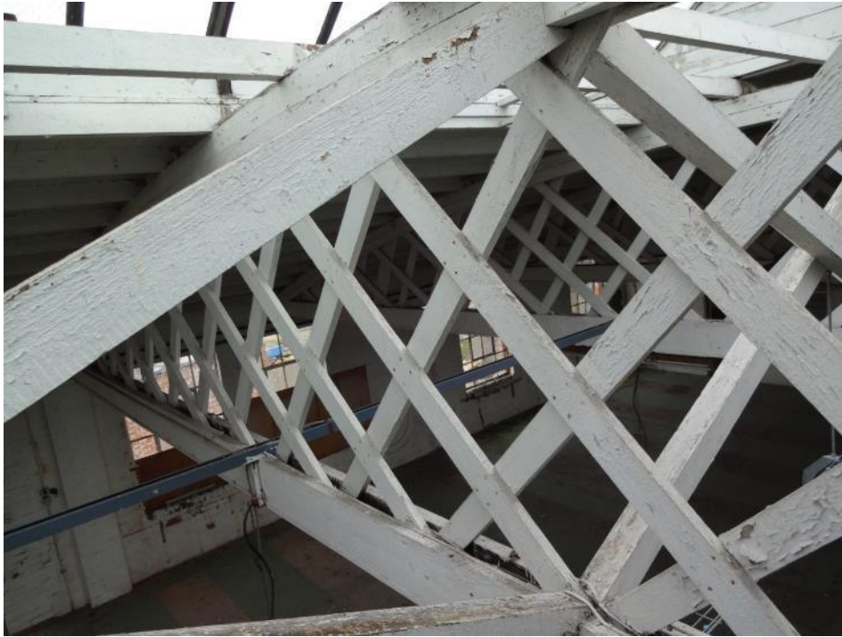
Plate 36: Detail of roof construction – Building 3
