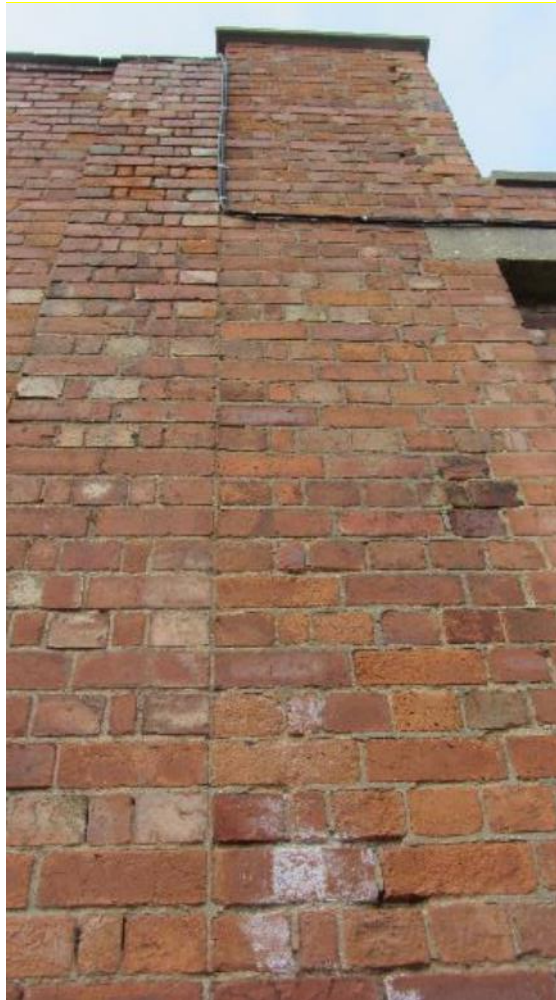
Plate 47: View from Hatherley Road showing construction break
