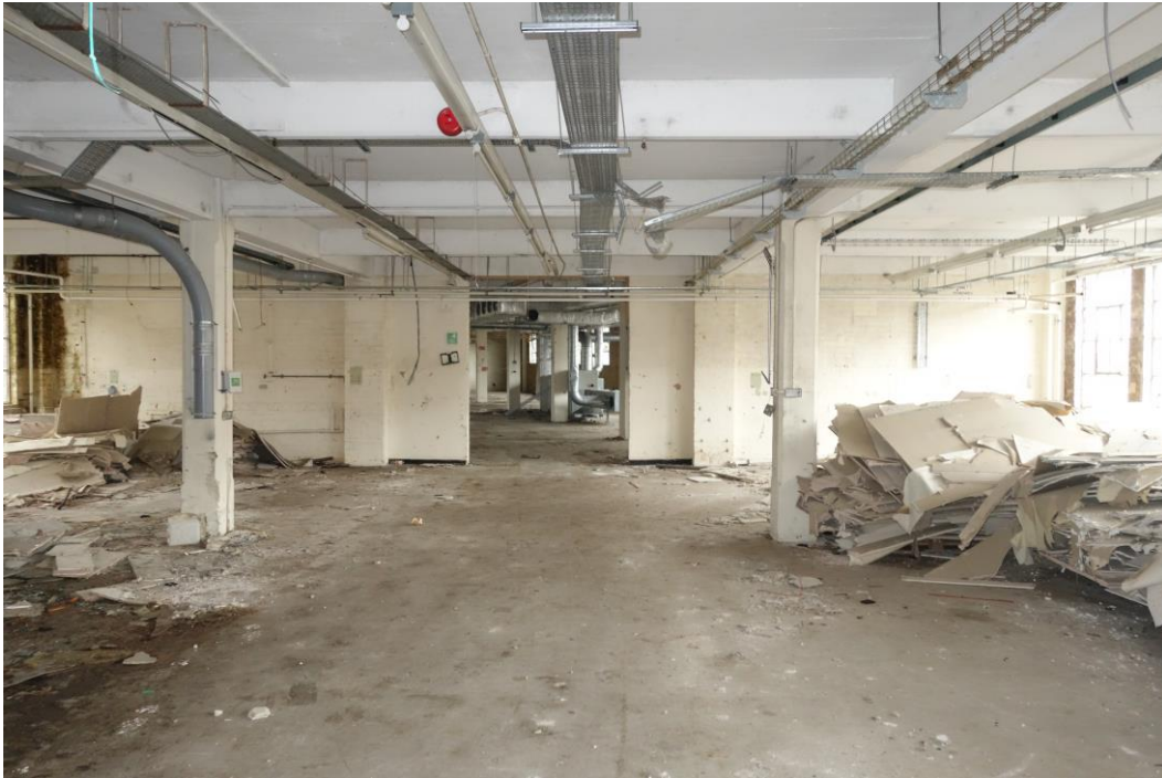
Plate 24: View NW showing internal cross-section consistent with Section B-B shown on 1942 plan (fig. 5)
