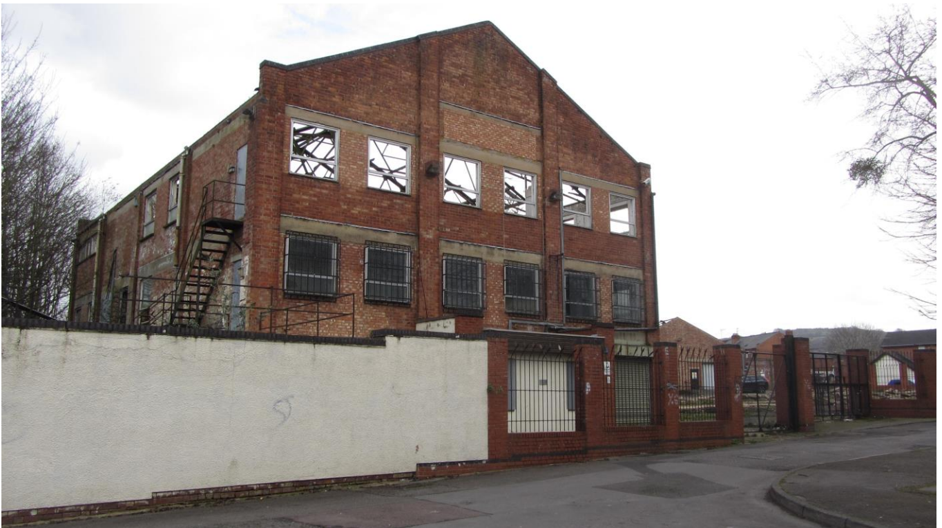
Plate 11: NW gable and NE elevation of Building 1
