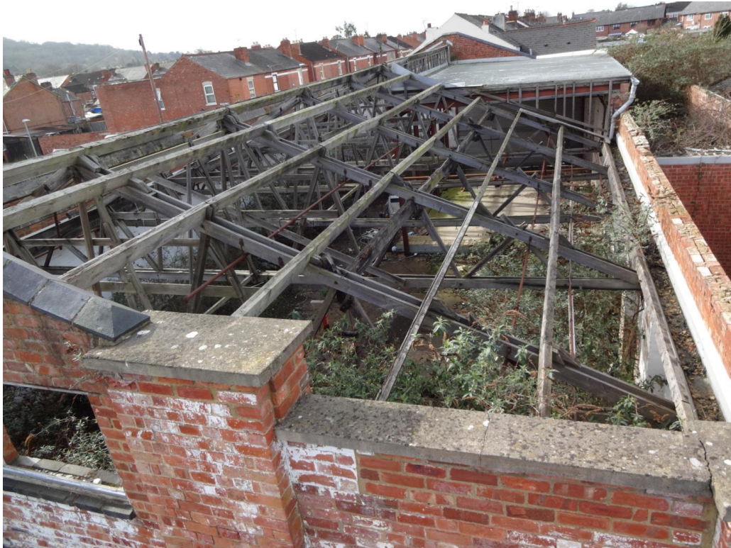
Plate 45: View SW of Building 7 showing roof structure
