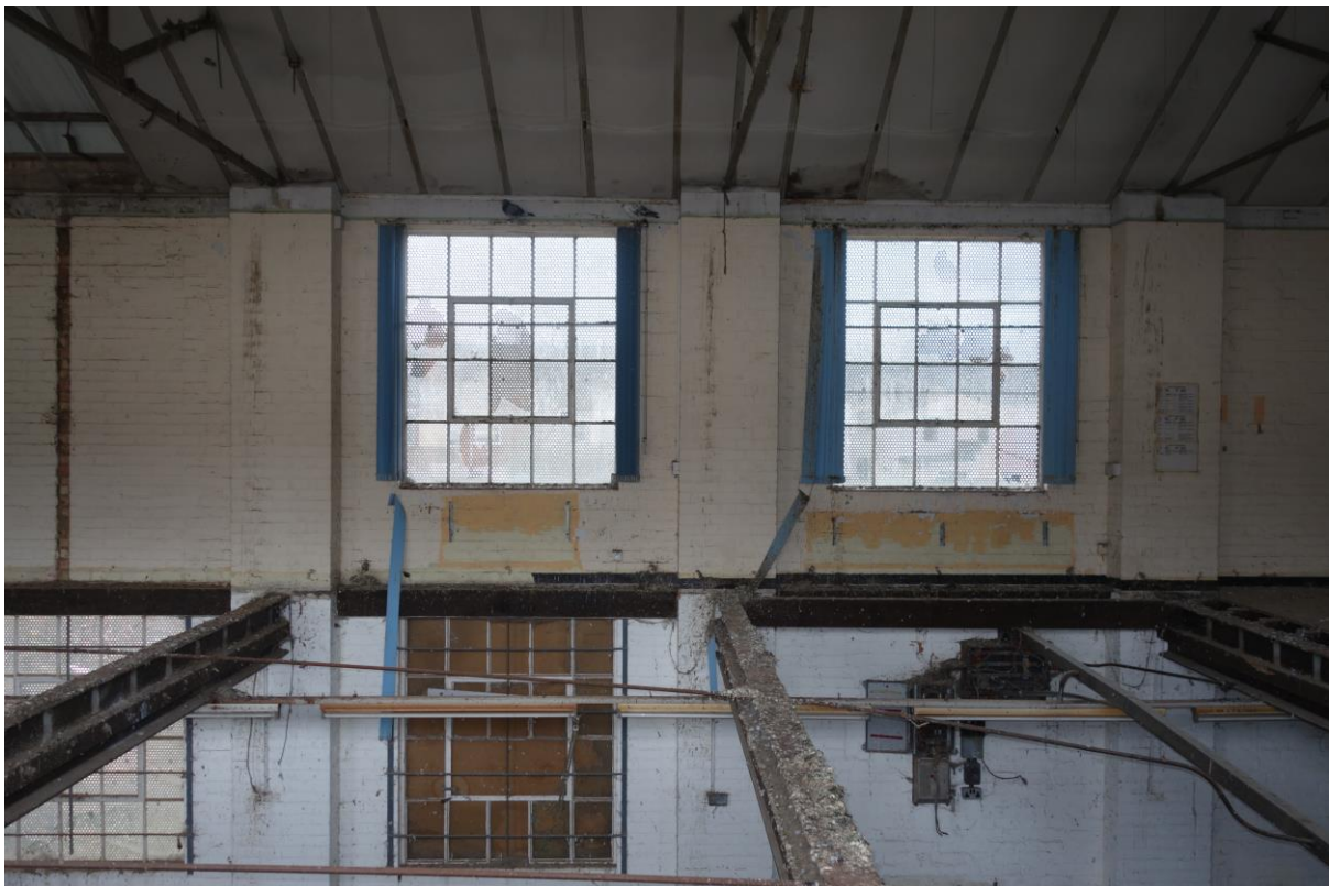
Plate 39: View NE of Building 4 showing internal structural detail
