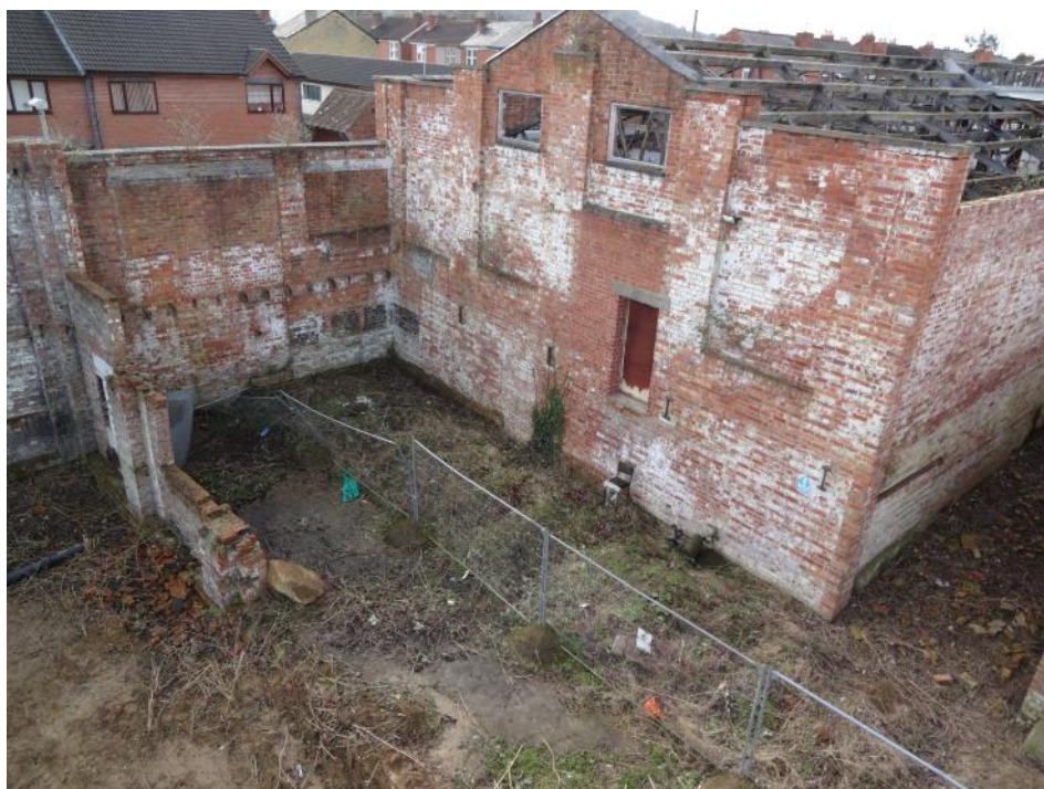
Plate 43: View of E elevation of Building 7
