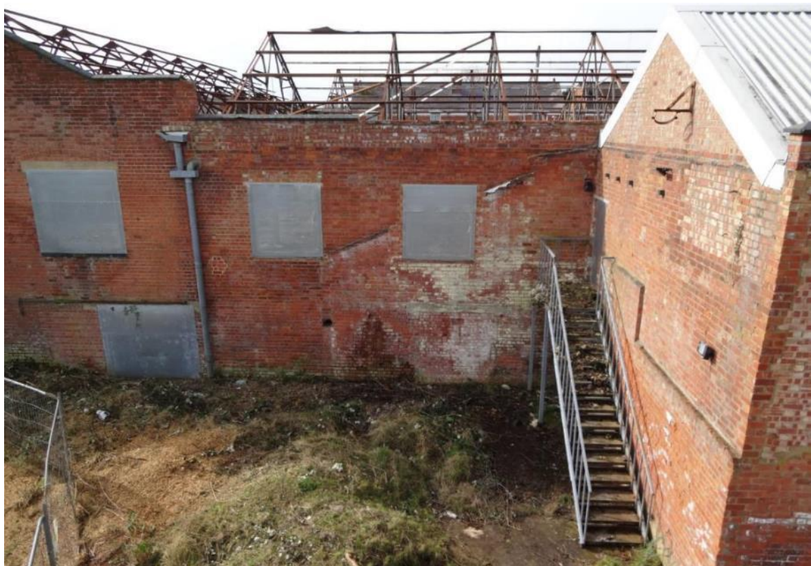
Plate 7: View SW showing stepped mono-pitch profile of building formerly attached to Buildings 4 and 5
