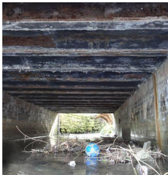
Plate 5: View of Sud Brook spanned by former Works buildings
