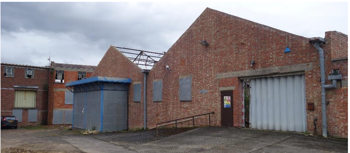
Plate 40 View E of NW elevation of Building 5 showing modern frontage with horizontal concertina folding door and concrete loading ramp
