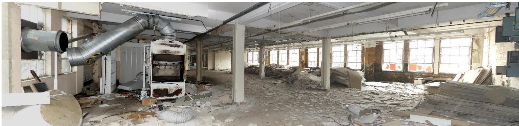
Plate 28: View showing ground floor of Building 3
