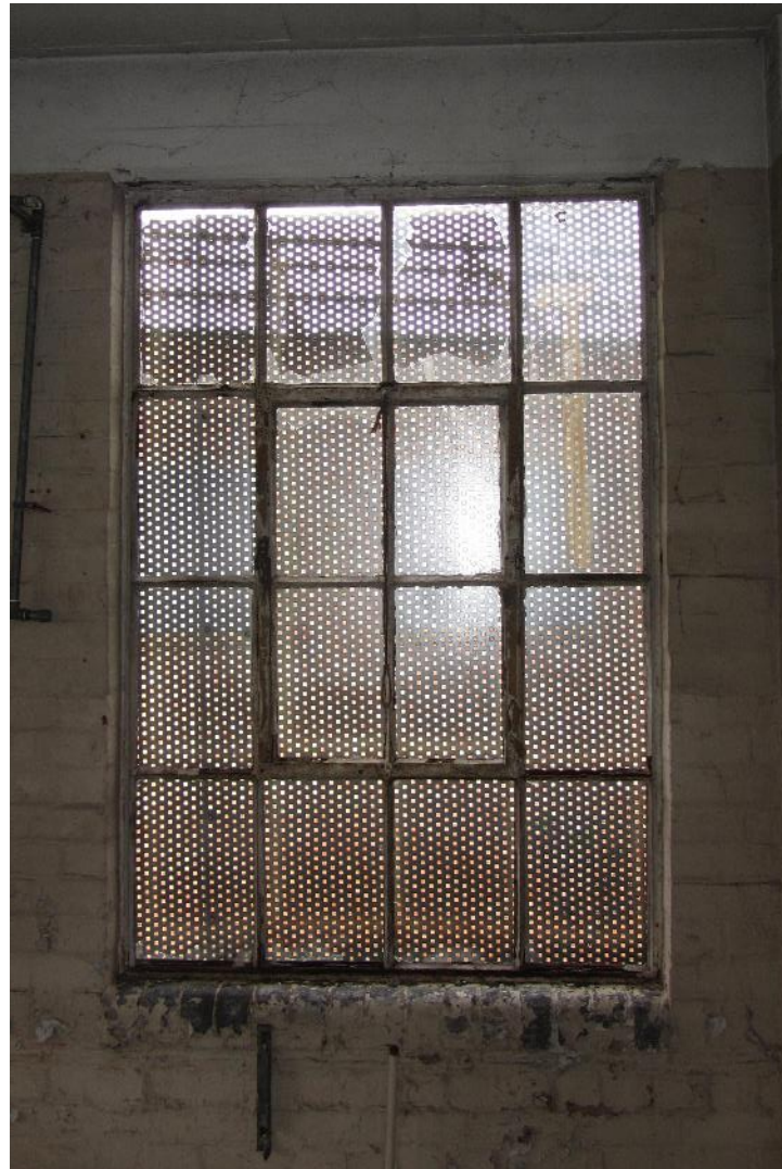
Plate 20: Detail of window in upper storey elevation of Building 3
