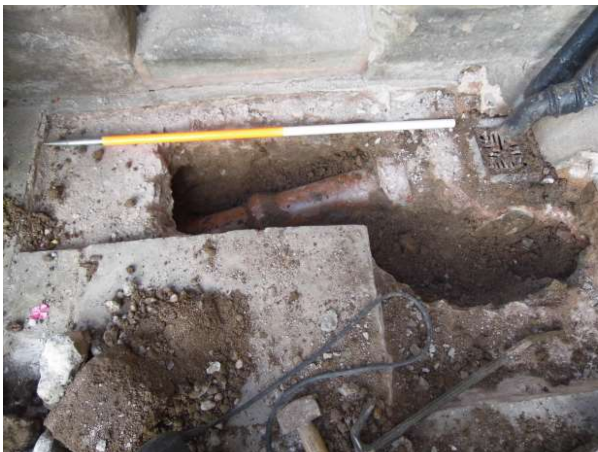
Plate 1: View W showing the existing drain following excavation
