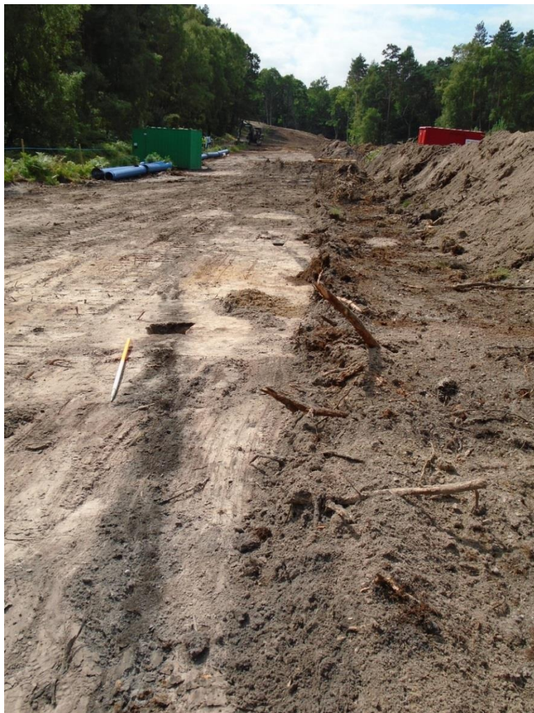
Plate 6: General view to the SW of plantation gullies [302] and [304]
