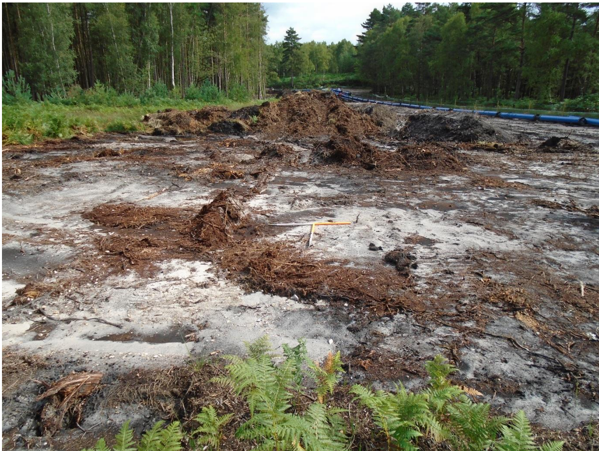
Plate 11: General view E of the site compound strip
